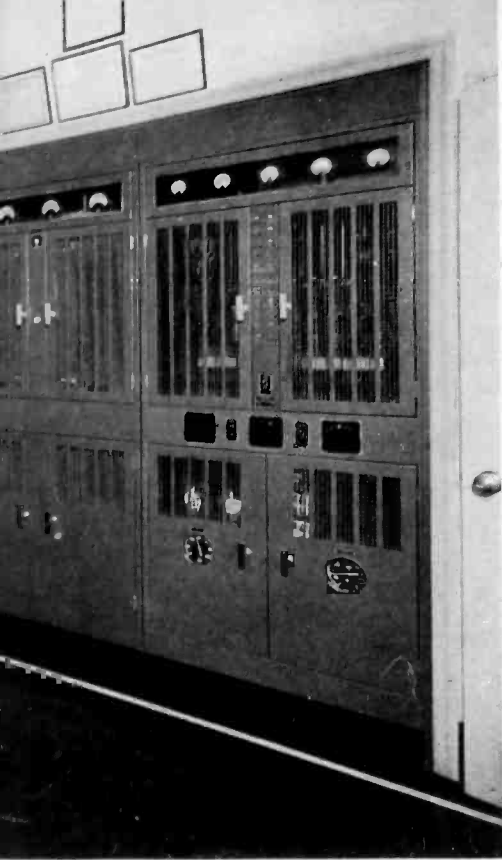
Control room showing Western Electric 5,000 watt transmitter neatly paneled along the wall. The speech input equipment with the 110A Amplifier is installed at the left of the operator's desk.
