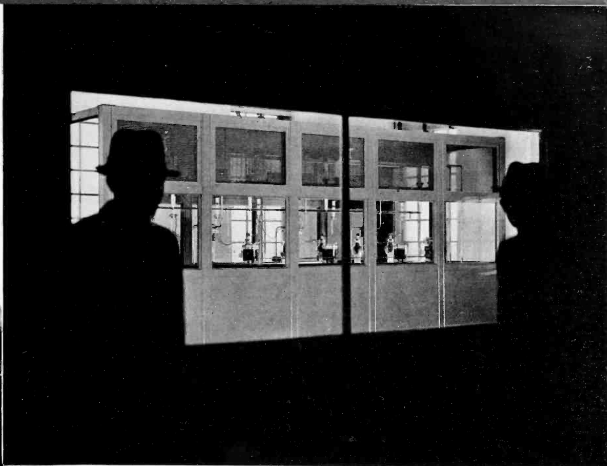
High-voltage rectifier tube unit showing 10 ampere rectifier tubes.
