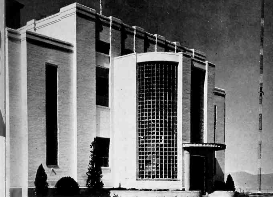
KSL transmitter building's new face and new 455 foot antenna. Circular structure at front encloses the new entrance stairway.
