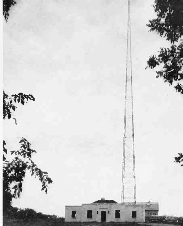
WKAR's 300-foot Blaw Knox shunt fed radiator.
