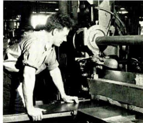
**E. L. Langford shearing a sheet of metal on the Niagara Shear.**
