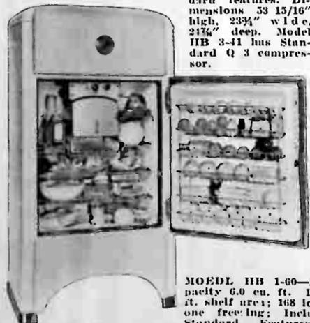
**MODEL HB 1-60**—Net capacity 6.0 cu. ft. 14.43 sq. ft. shelf area; 168 ice cubes one freezing; Includes all Standard Features with Hermetic Unit T 1 with still air condenser. Dimensions 58 7/16" high, 31" wide, 25 1/16" deep. Model HB 3-60 has Standard Q 3 type compressor.
