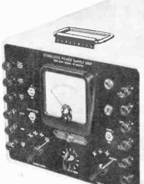
Type 1930; + 220 to 380V variable; • 100mA; regulation '5%; ripple 2.5mV. Negative stabilised—150V at 20mA. Delivery ex Stock
