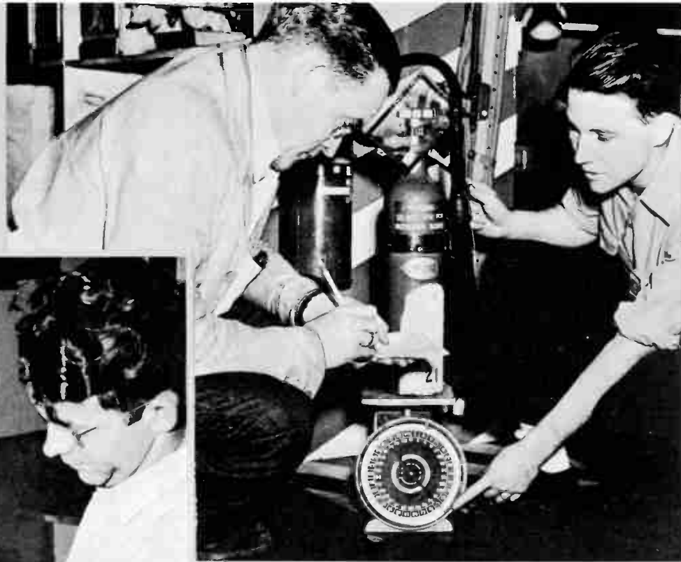
Vic Robelet is shown here weighing a CO 2 extinguisher and Jack Smith is recording their findings on a card. If the cylinder shows a loss of weight it indicates it has either been used or that it is leaking and the cylinder is replaced by a spare while it is sent out to be recharged and checked.
