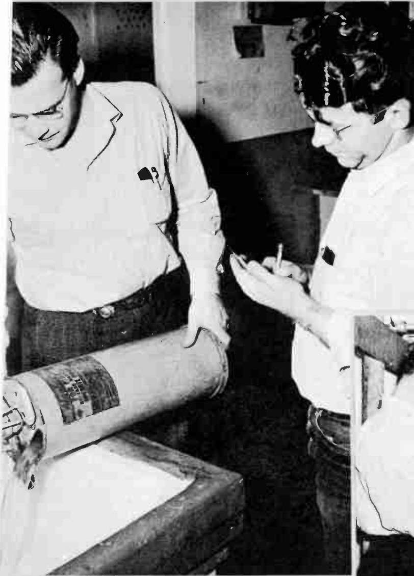
Regular hand pump types of extinguishers which contain plain water are placed all around the plant. In this picture, Bob Pearl is emptying one of the Chemical department water extinguishers. Dave Book records the date of the emptying. Although this type of extinguisher is emptied, cleaned and refilled but once a month, the fire crew still checks them on their weekly tour along with the other type extinguishers—the Pyrene, Foamite and CO 2 .
