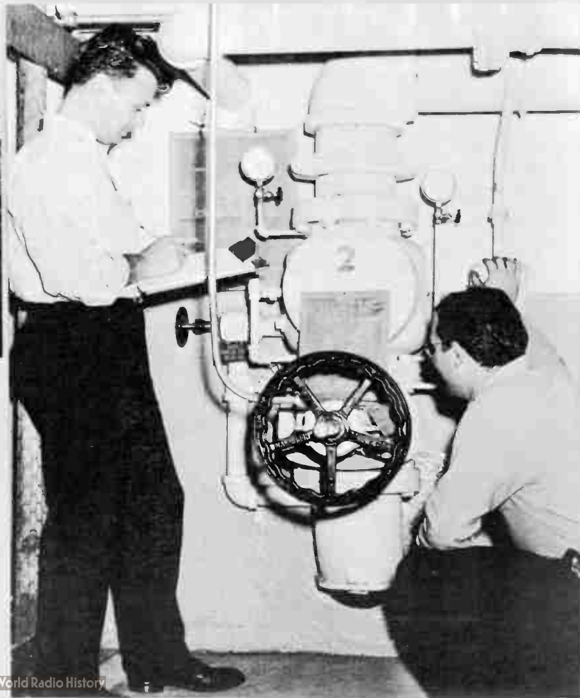
Vic Robelet is shown here weighing a CO 2 extinguisher and Jack Smith is recording their findings on a card. If the cylinder shows a loss of weight it indicates it has either been used or that it is leaking and the cylinder is replaced by a spare while it is sent out to be recharged and checked.
