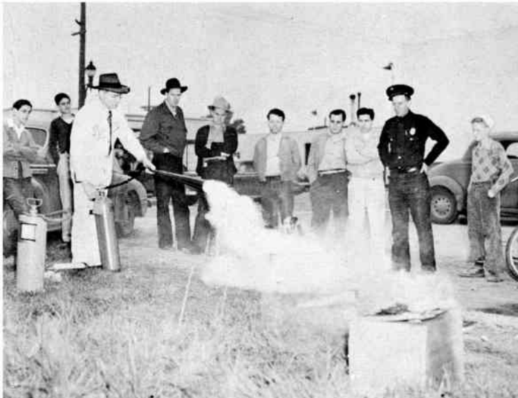
Members of the day shift fire crew gathered in a neighborhood lot to witness a demonstration of various fire extinguishers under fire. At left, a Co2 type is used to smother the flame, while a pyrene type is used at right. The Co2 is used chiefly to combat electrical fires—the pyrene for any type fire
