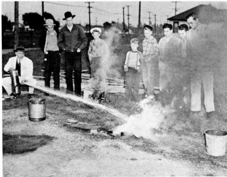
Members of the day shift fire crew gathered in a neighborhood lot to witness a demonstration of various fire extinguishers under fire. At left, a Co2 type is used to smother the flame, while a pyrene type is used at right. The Co2 is used chiefly to combat electrical fires—the pyrene for any type fire
