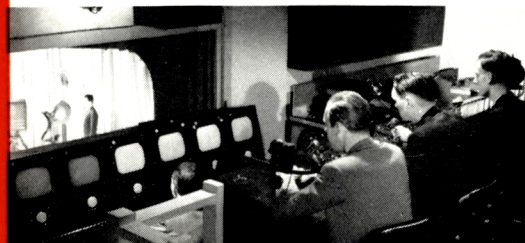
2. In the control room, the directors watch the monitors to see what each camera is picking up, and indicate which picture is to be sent out over the air.
