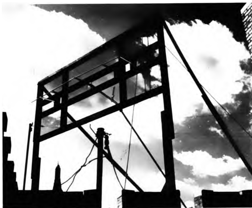
TRANSMITTING antenna, here shown in experimental form, is a Franklin type completely enclosed and mounted on the roof of a 62-floor building
