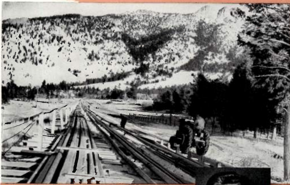
Half-mile lengths of cable sheathed in steel pipe wait in the shadow of the Rockies to be drawn into the tunnel mouth. The sections travelled on the dollies lying on the tunnel's floor (below), and were joined and hung from the ceiling.
