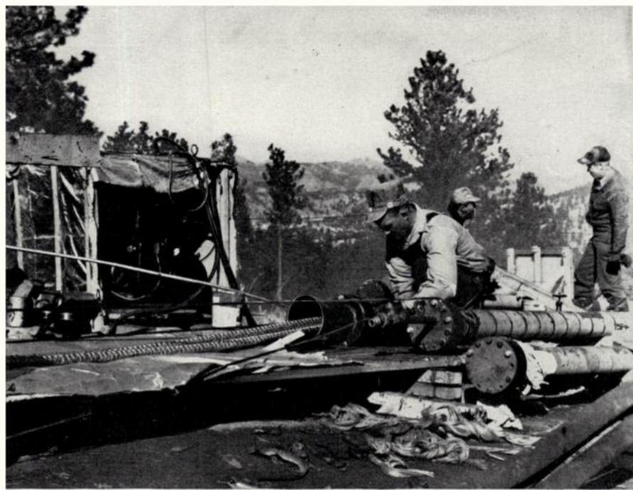
Getting the cables into a half mile of pipe was tricky. A plunger hooked to a light wire was blown through with air. The wire was used to pull a winch line through, and the line, in turn, dragged the cables into place.
