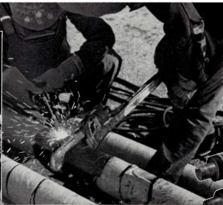
When the steel casings were welded together, the joints between them had to be not only watertight but airtight, in order to contain a protective atmosphere of nitrogen.
