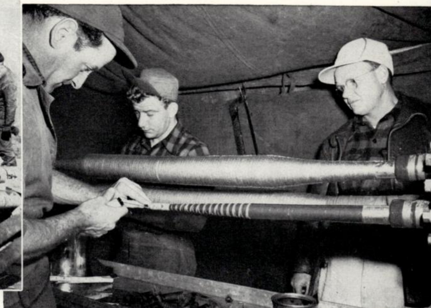
When the cables were moved into the tunnel, the sections had to be joined to form a continuous line. Here, three men splice two of the long sections.
