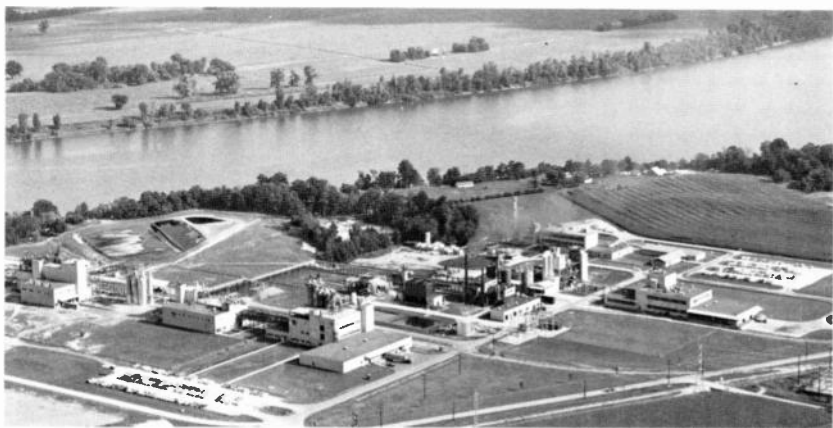
TOP PLANT: The Company's LEXAN® polymer plant at Mt. Vernon, Indiana has been named one of the top ten U.S. manufacturing plants of 1966 by Factory magazine. The facility was selected from over 1500 others that began operations last year and cited for its autonomous layout and heavy emphasis on employee safety. The plant is operated by the Chemical Materials Department and is the country's largest facility for the production of polycarbonates. Receiving the Factory award were Dr. George E. McCullough, manager of the Mt. Vernon plant, Walter J. Dugan, department general manager, and Dr. Charles E. Reed, vice president and general manager of the Chemical and Metallurgical Division. In the 33-year history of the "Top Ten" competition, General Electric Company has earned eight awards — the highest number given any company. Other GE award-winners: Tiffin, Ohio (1947); Coshocton, Ohio (1948); Schenectady, N.Y. (1950); Louisville, Ky. (1955); Bloomington, Ill. (1956); Tyler, Texas (1957); Valley Forge, Pa. (1962).
