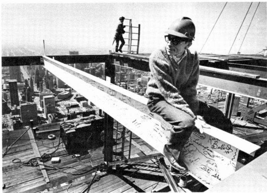
GE COMPUTER ENGINEER WALT ANDERSON CHECKS CHICAGO'S VIEW FROM 100 STORIES UP.
