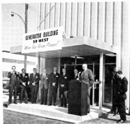
DEDICATING BUILDING 59 WEST
