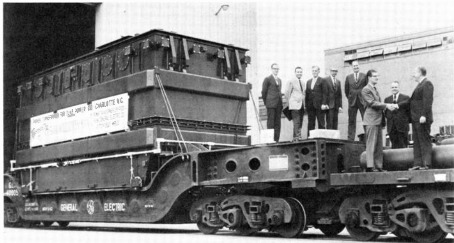
A MIGHTY BIG TRANSFORMER ROLL-OUT AT PITTSFIELD
