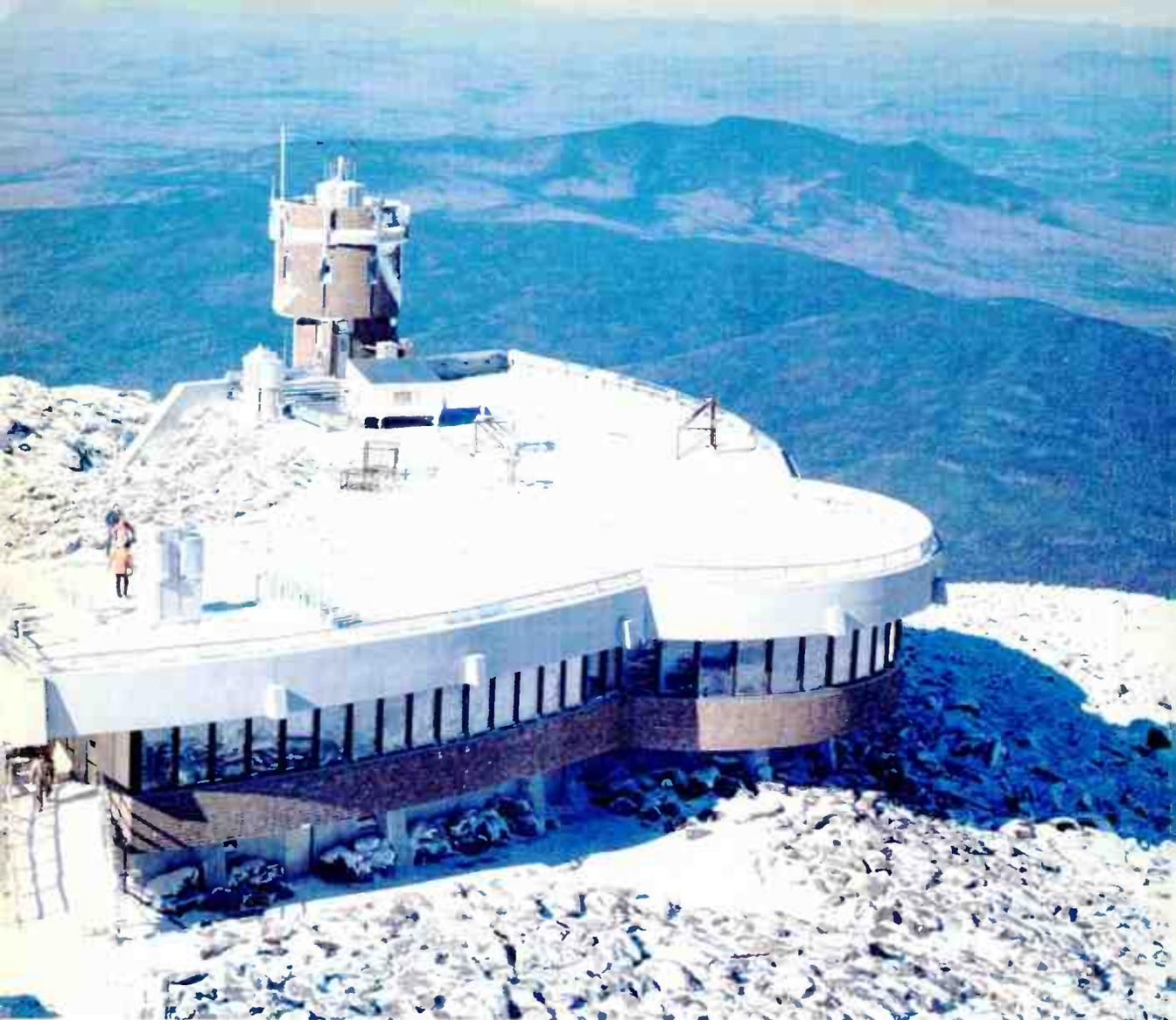
GE engineered materials provide builders with new techniques in designing new buildings and preserving older ones. Above: New Mount Washington State Park Summit Building utilizes Lexan® sheet as glazing material. Right: Lexan sheet protects valued stained-glass windows at Bethel AME church in Bridgeport, Conn. Below: GE silicone roofing system is applied over older roof at Monument Mountain School in Great Barrington, Mass.
