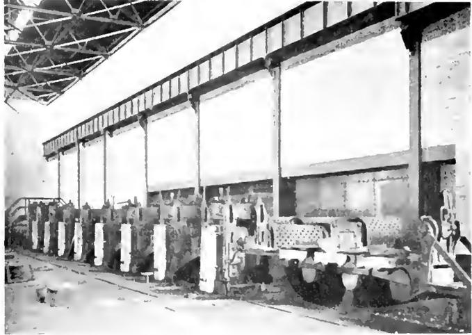
Fig. 3. Sheet Bar Mill, Showing Eight Stands of Rolls, Steam Flying Shear and Crop Shear
