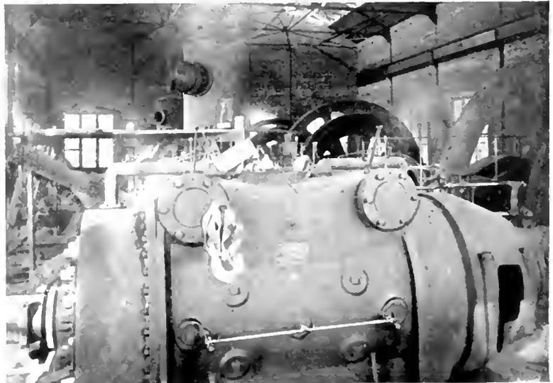
Fig. 25. Interior of Hoist Compressor Plant During Construction
