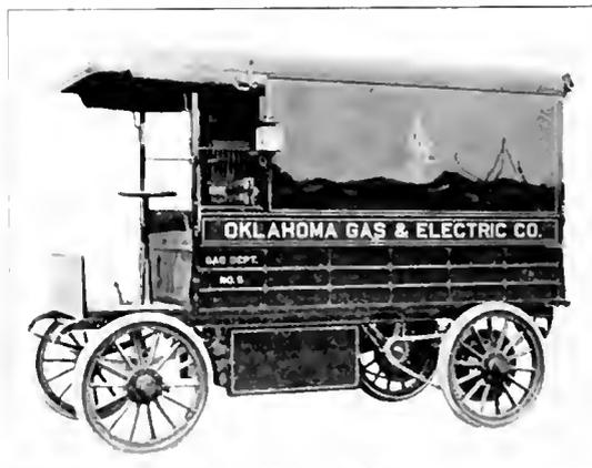
Fig. 7. 2000 Lb. Electrically Propelled Truck
