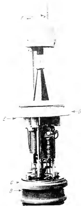
Fig. 16. Method of Insulating Lamp from Ornamental Post
