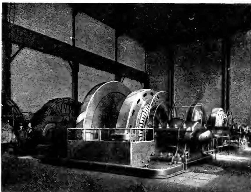
Fig. 5. 2000 H.P., 214 R.P.M. Induction Motors with 100,000 Lb. Laminated Steel Flywheels
