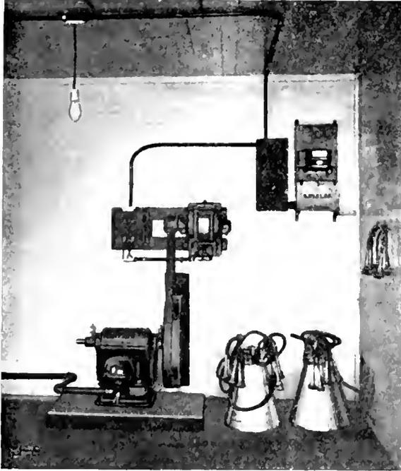
Fig. 3. Motor-Driven Vacuum Milking Outfit
