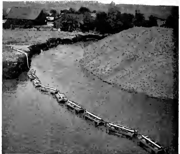
4000 Volt Armored Shore Cable Connecting High Tension with Transformers on Dredge
