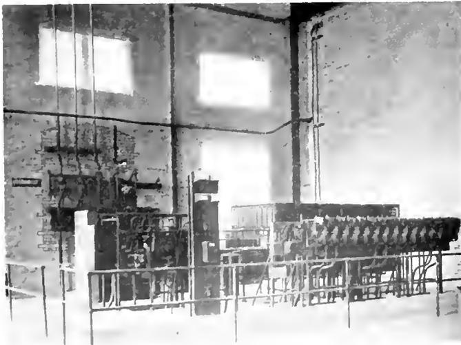
Fig. 2. Primary and Secondary Control Equipment for 6000 H.P. Motor
