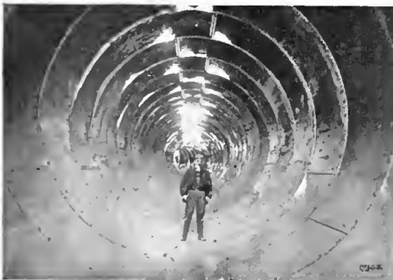
Fig. 8. Interior of One of the 15 Ft. 6 In. Steel Pipes
