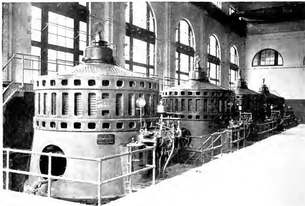
3000 Kw., 40 Cycle, 3-Phase, 4400 Volt, 300 R.P.M. Waterwheel-Driven Alternators
