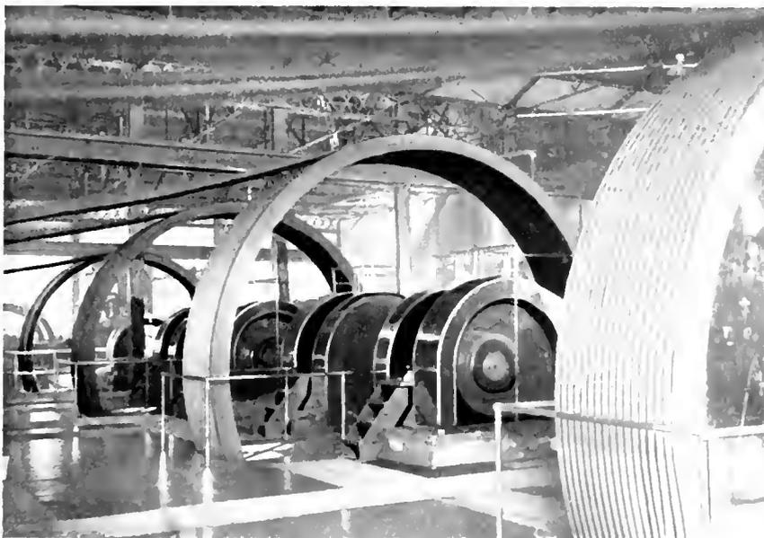
Fig. 22. Leonard Compressor Plant, showing 2300 H P in Compressors
