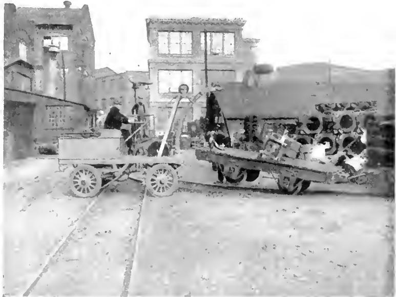
Placing Derailed Flat Car on Track
