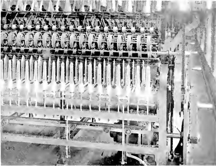
Fig. 4. 7 1/2 H.P. Induction Motor Arranged for Individual Drive of Spinning Frames
