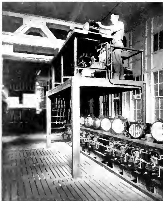
Fig. 8. Testing Arc Headlights
