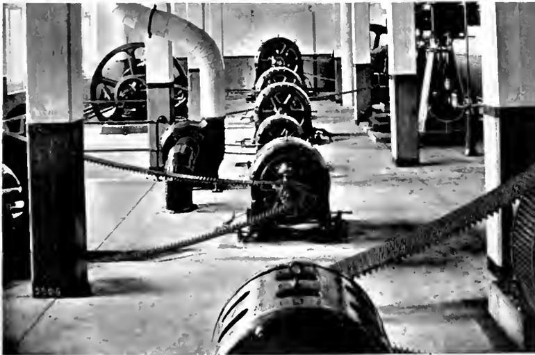
Fig. 2. Motors Driving Compressors and Pumps in Solvent Plant by Chain Belts
