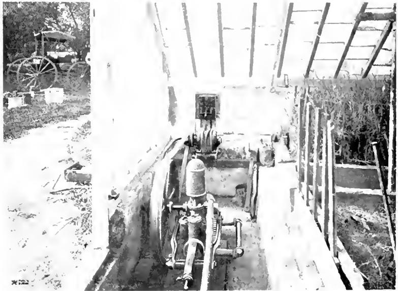
Fig. 17. Induction Motor Belt-Connected to Pump Located in Green House
