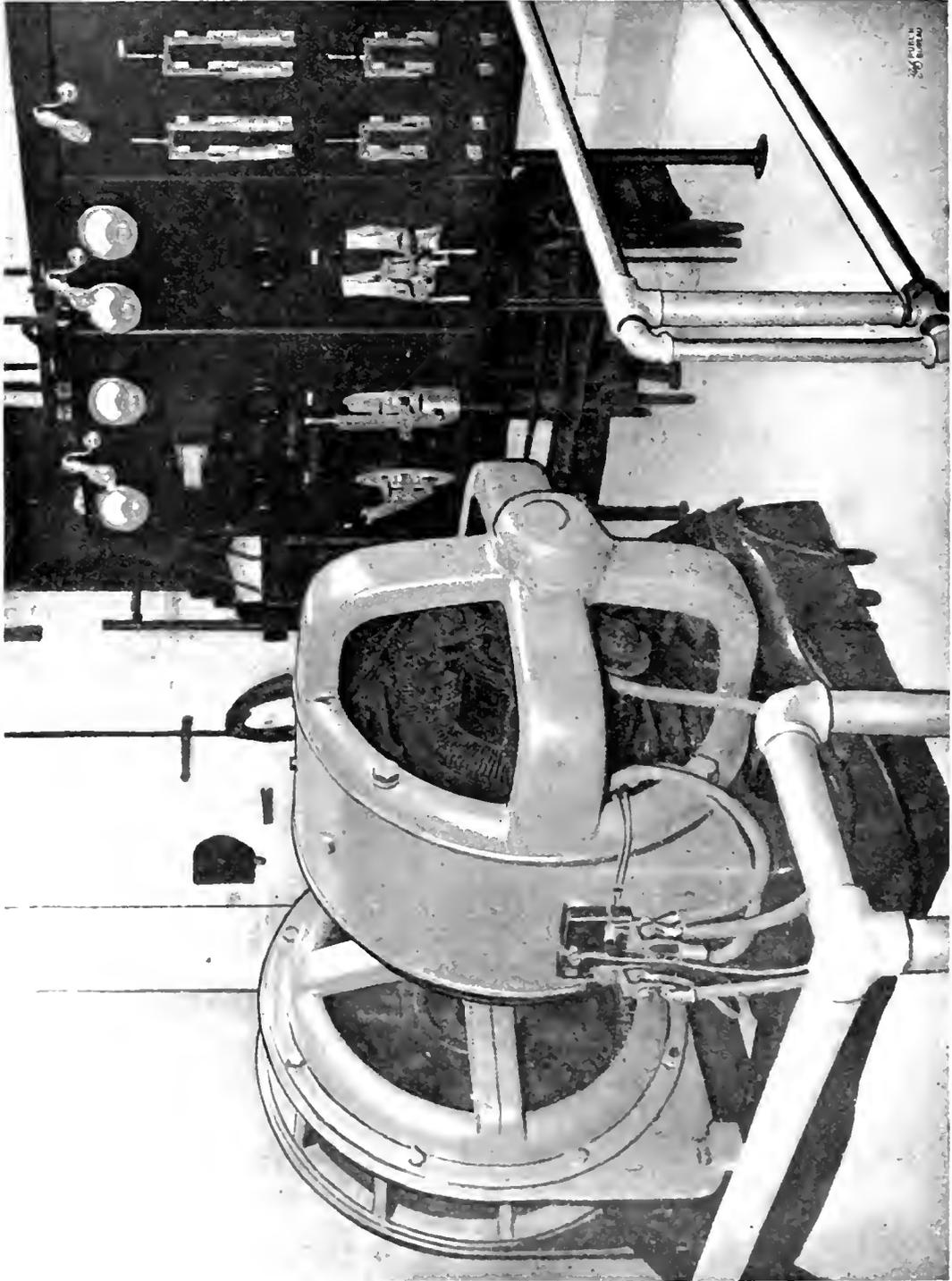
170 Kv-a. Synchronous Condenser Generator Set
