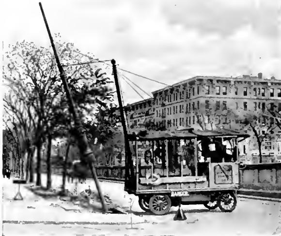
Fig. 5. Winch Equipped Truck
