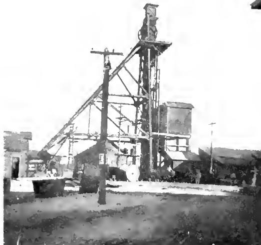
Fig. 23. Mountain View Hoist, operated by Compressed Air
