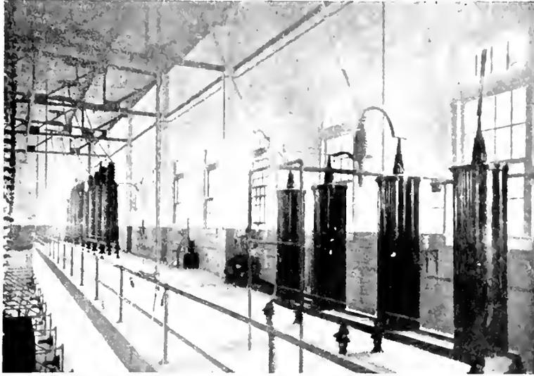
Fig. 18. Butte Substation, showing Electrolytic Lightning Arresters
