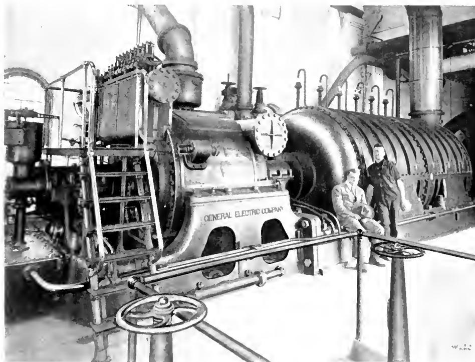
Fig. 1. Air Compressor Direct-Connected to Curtis Steam Turbine, 1500 R P M.
