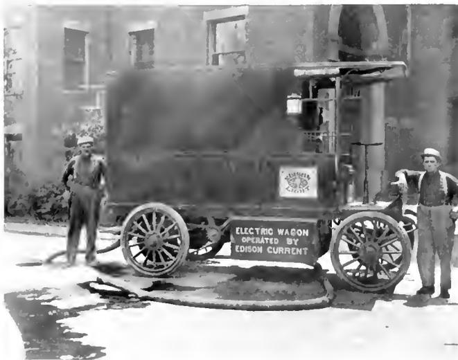
Fig. 1. Electrically Propelled Vehicle, Containing a Motor Driven Centrifugal Pump
