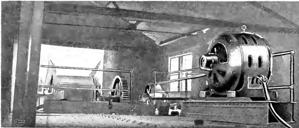
75 H.P. Induction Motor Driving Bucket Conveyor at No. 2 Tipple,
