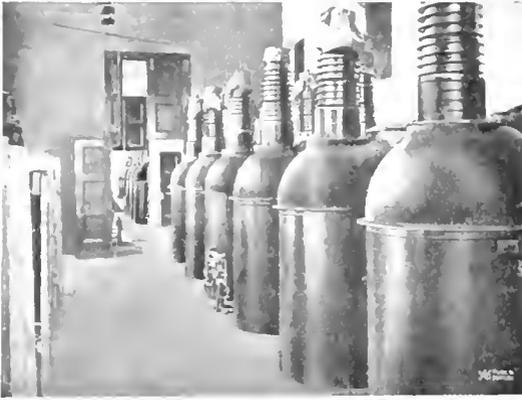
High Tension Oil Switches in Substation of Stanislaus Power Company
