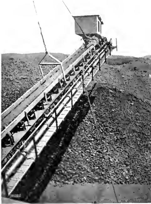
View of Stacker Showing Shed for Motor Driving Conveyor
