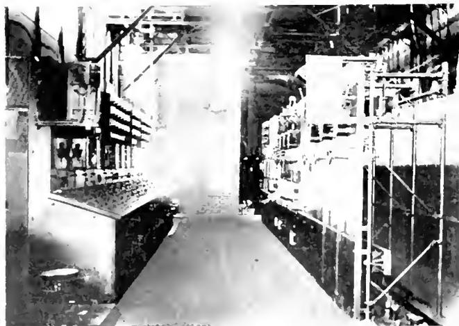
Fig. 4. Control Benchboard and Switchboard
