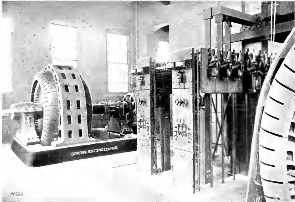
Fig. 3. Two 1650 kv-a., 440 volt, 500 r.p.m. Synchronous Condensers and Control Panels Substation, Universal Portland Cement Company, Buffington, Ind.
