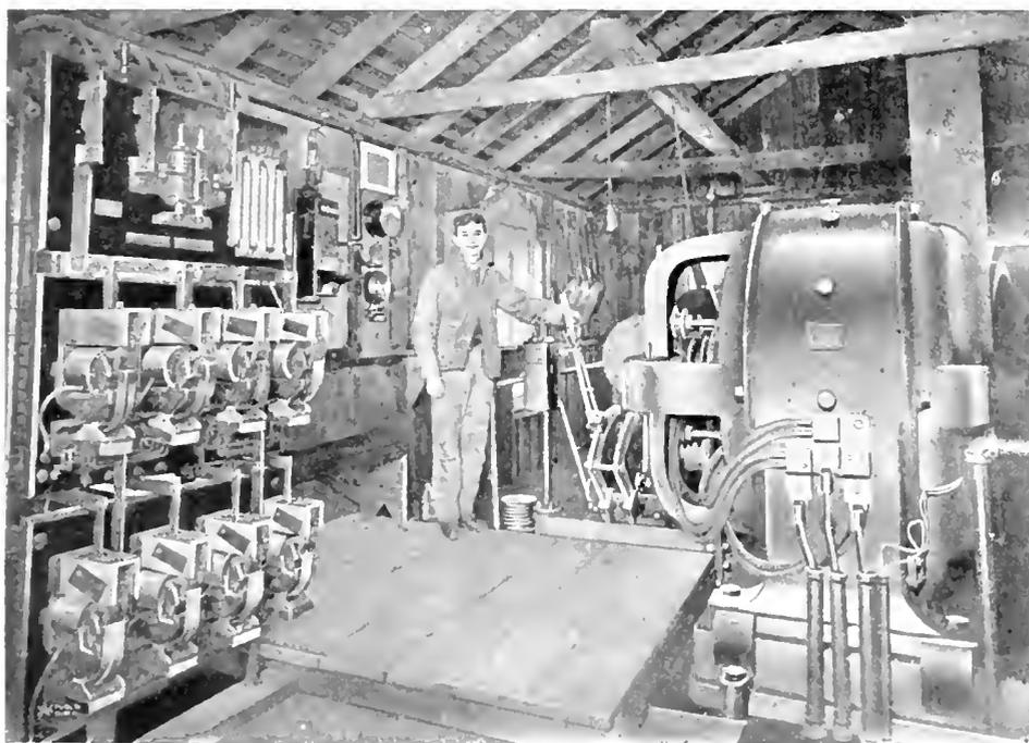
170 H.P. 220 Volt 385 R.P.M. Compound Wound Motor Driving "Trial" Slope Hoist. Contactor and Relay Panel Shown on the Left. Lincoln (Pa.) Colliery, Philadelphia and Reading Coal and Iron Company
