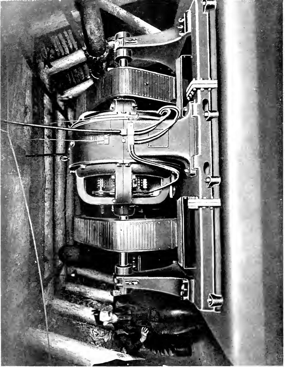
170 H.P. 300 450 R.P.M. Motor Driving 10 In Quintuplex Pump Through Gears; Operating Head 400 Ft.
