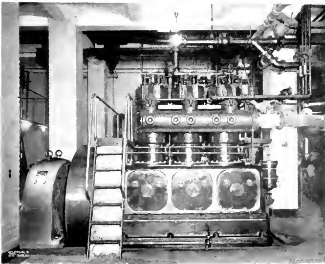
Fig. 2 150 Kw. Gas Engine and Generator Set
