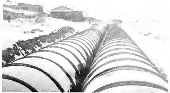
Fig. 7. Steel Pipes, 15 Ft. 6 In. in Diameter
