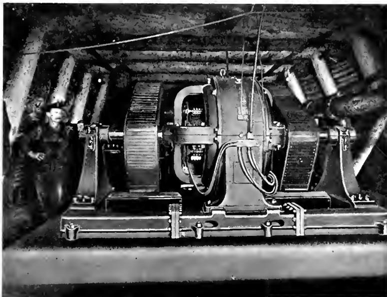
170 H.P. 220 Volt 300-450 R.P.M. Direct Current Motor Driving 10 Inch Quintuplex Pump Through Gears Operating Head 400 Feet. Kohinoor Colliery near Shenandoah, Pa. Philadelphia & Reading Coal & Iron Co.
