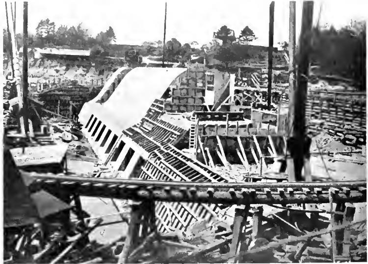
Fig. 2. Spillway of Dam in Course of Construction Showing Location of the 10 Floodgates
