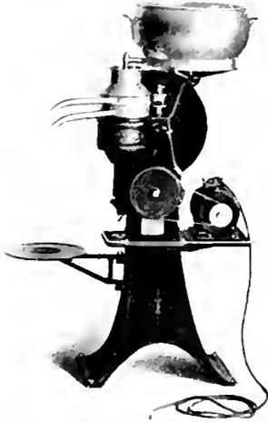
Fig. 7. Motor-Operated DeLaval No. 15 Separator
