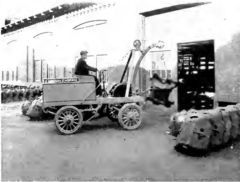
Carrying Railway Motor Castings into Machine Shop
