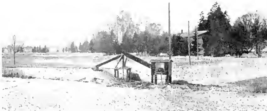
Fig. 16. Motor Driving Pump for Farm Irrigation
