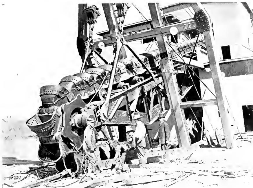
Motor-Operated Bucket Line, Close Connected Type
