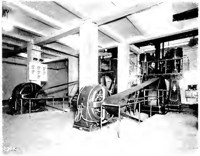
Fig. 3. One 90 H.P. and One 125 H.P. Motor Driving Ammonia Compressors
