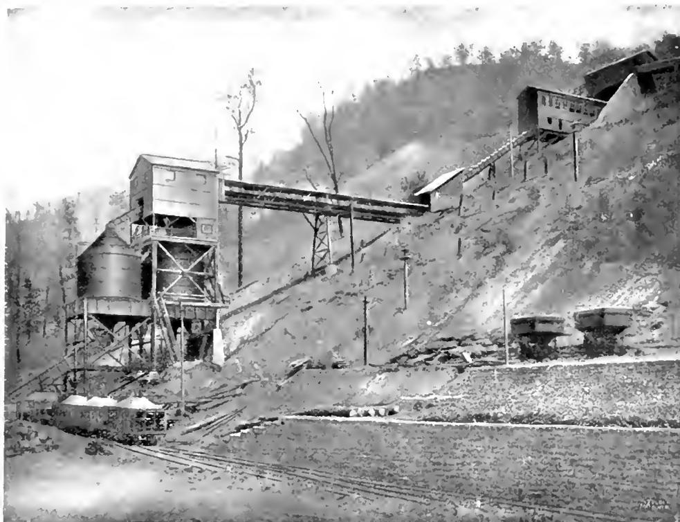
No. 4. Tipple of the United States Coal & Coke Co., Gary, W. Va., showing Arrangement of Motor Driven Steel Belt Conveyors
