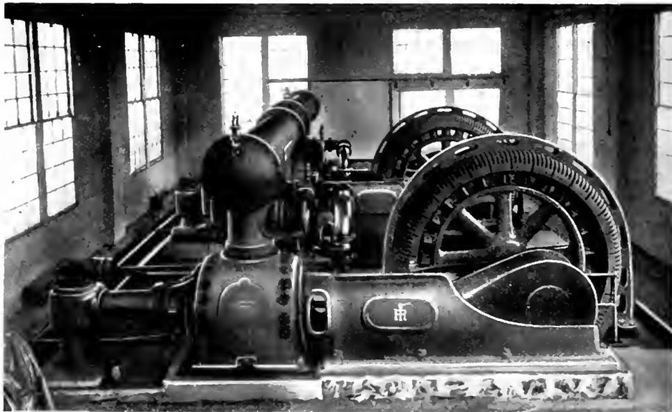
Air Compressors—Capacity 2650 cu. ft. at 100 lb. in Lucerne Substation No. 2, each Direct Driven by an AT1 450 Kw-a. 6000 Volt 125 R.P.M. Synchronous Motor.
