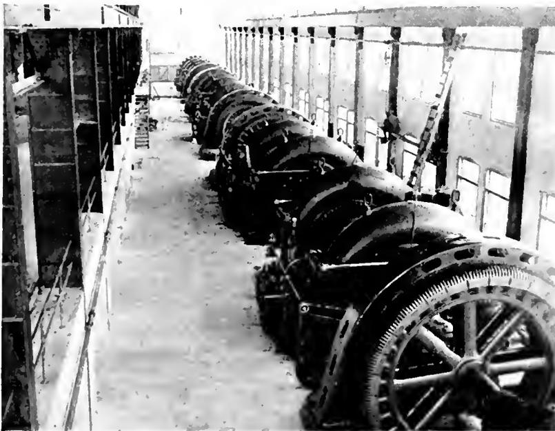
Fig. 12. Generator Room in Rainbow Station, Showing Six 6000 H.P. Generating Units
