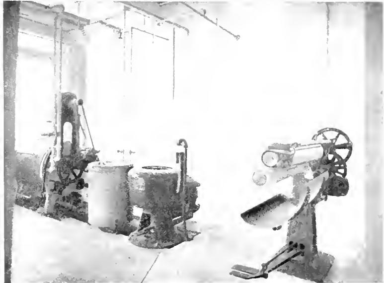
Fig. 4. Laundry From Left to Right. Washer Driven by 2 H.P., 220 Volt Induction Motor; Centrifugal Dryer Driven by  $\frac{1}{2}$  H.P., 220 Volt Induction Motor; Mangle Driven by  $\frac{1}{2}$  H.P., 220 Volt Induction Motor
