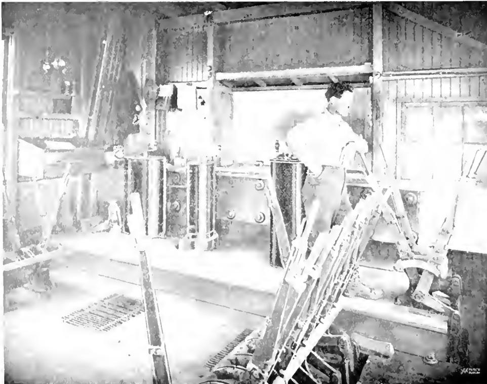
Winch Room of Natoma Gold Dredge Showing Controllers for Operating Bucket Line, Screen and Winch Motors
