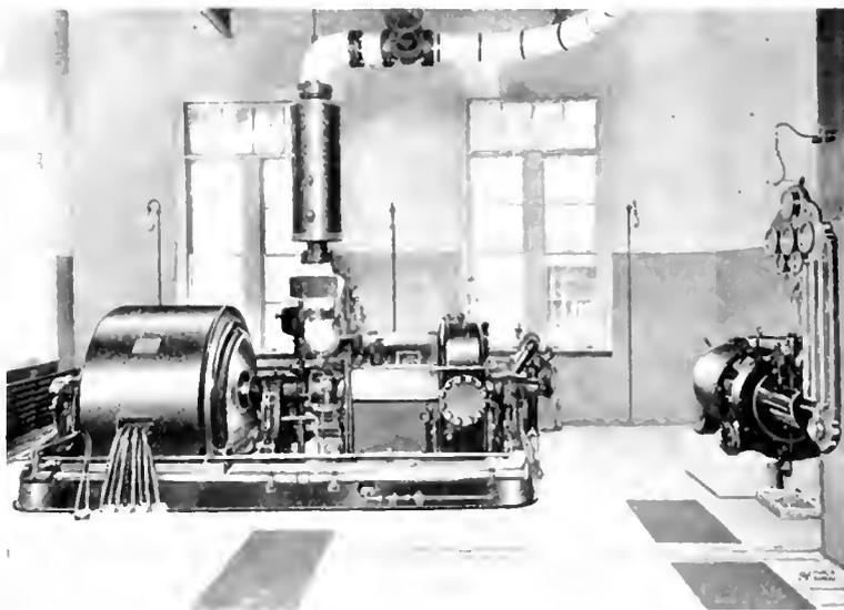
Fig. 1. 500 Kw. Curtis Turbine-Generator Set and Exciter
