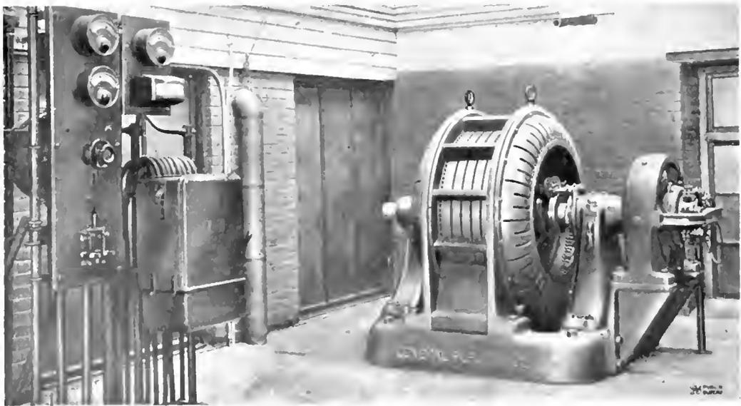
Fig. 6. 300 kv-a. 600 volt, 720 r.p.m. Synchronous Condenser - Saxony Worsted Mills, Bemis, Mass.
