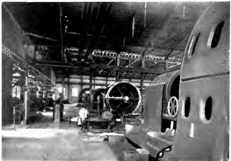
Fig. 21. Leonard Compressor Plant, showing 2300 H.P. in Motors
