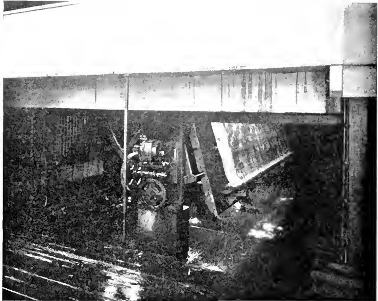
Fig. 3. Tilting Table for Lowering Ice Cakes into Horizontal Position
