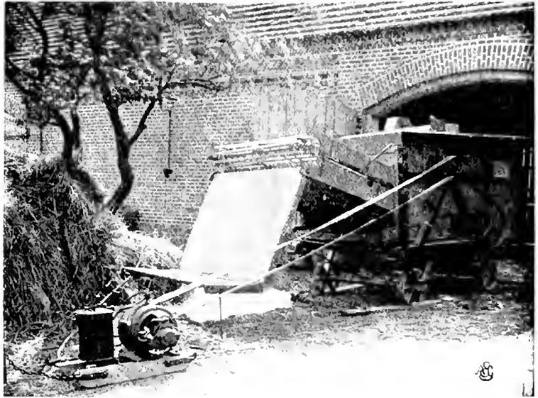
Fig. 1. Portable Motor Outfit Used for Driving Auxiliary Farm Machinery
