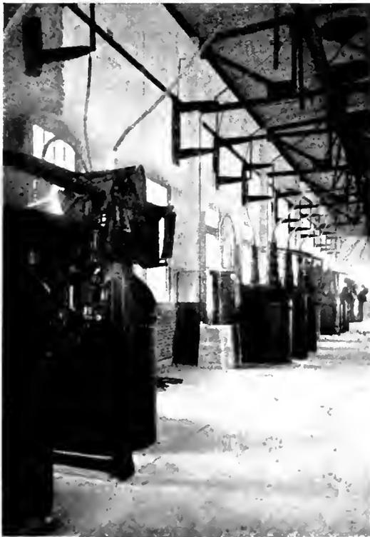
Fig. 19. Interior, Butte Substation, showing 100,000 Volt Line Switches
