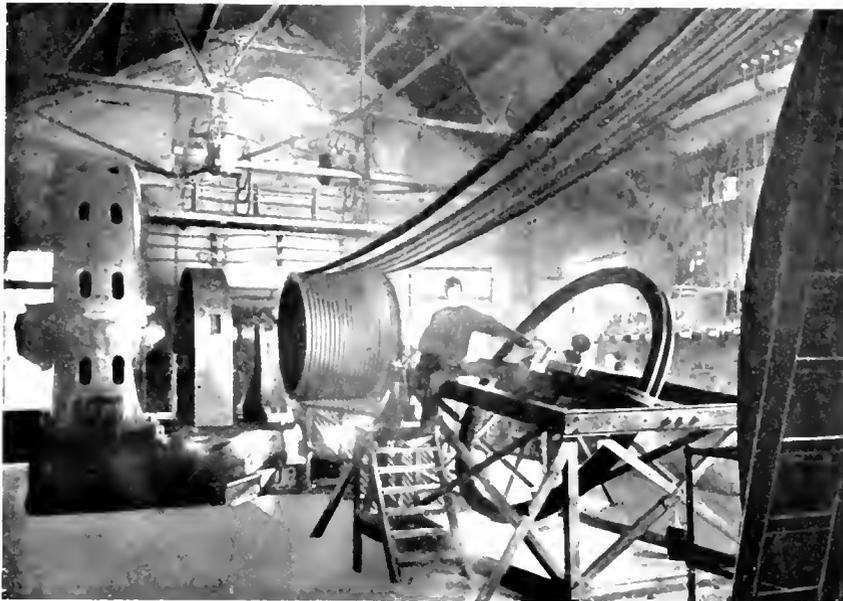
Fig. 26. Never Sweat Compressor Room, showing 900 H.P. Motor Driving Air Compressors
