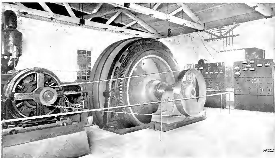
400 Kw. 2300 Volt Three-Phase 60 Cycle Engine-Driven Alternator with Belted Exciter and Switchboard in Power House. Bear Valley Colliery, Shamokin, Pa., Philadelphia and Reading Coal and Iron Company
