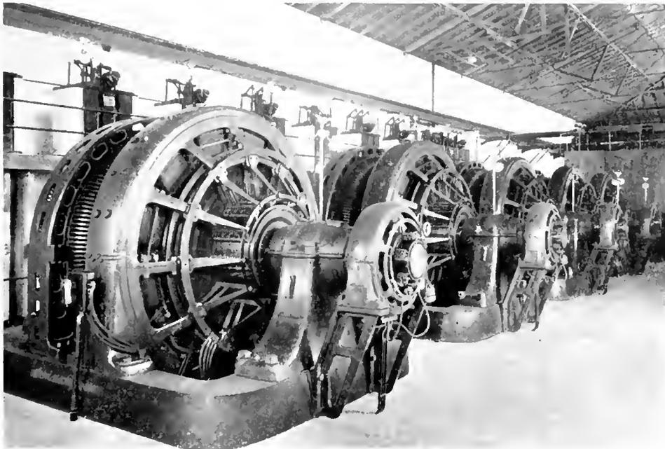
Substation Containing 1500 Kw. Synchronous Motor-Generator Sets
