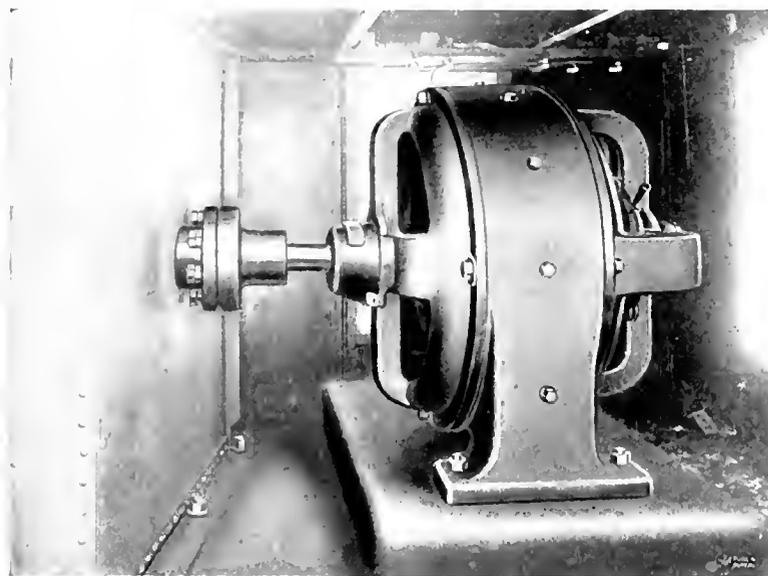
50 H.P. 230 Volt 200-400 R.P.M. Shunt Wound Motor Direct Coupled to
