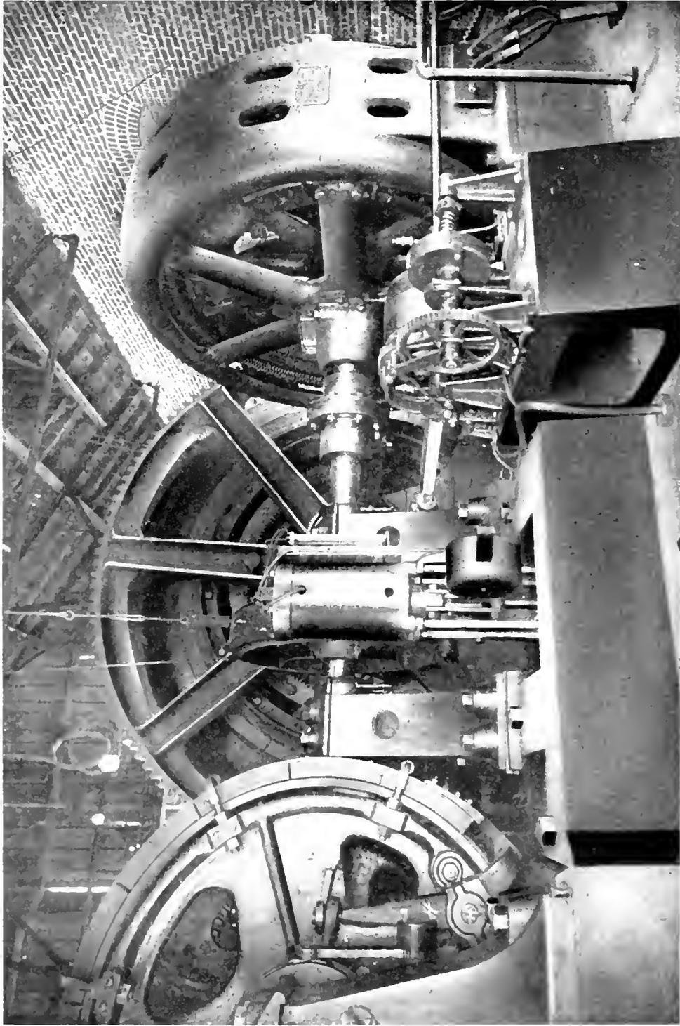
800 H.P., 2200 Volt, Squirrel Cage Induction Motor Geared to Water Hoist
