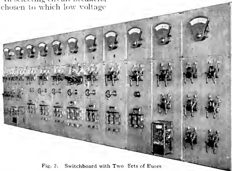
Fig. 2. Switchboard with Two Sets of Buses
