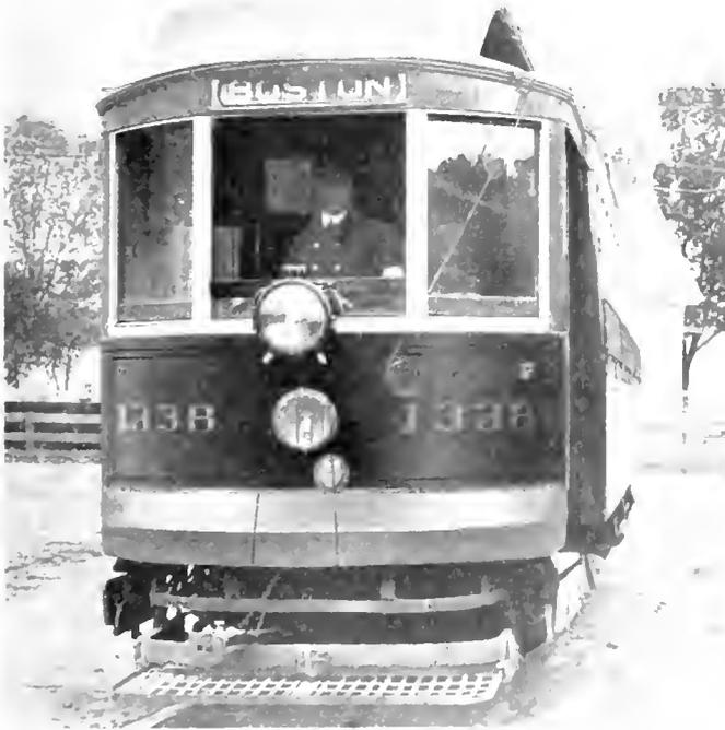
Fig. 3. Four-Ampere Luminous Arc Headlight Installed on Interurban Car
