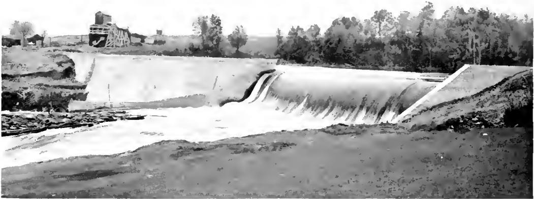
Fig. 3. View From Down Stream Showing Spillway and Impounding Section of Dam
