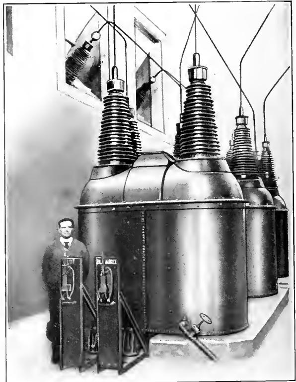
Fig. 7. 140,000 Volt Oil Switches in Zilwaukee Substation of Eastern Michigan Power Company
