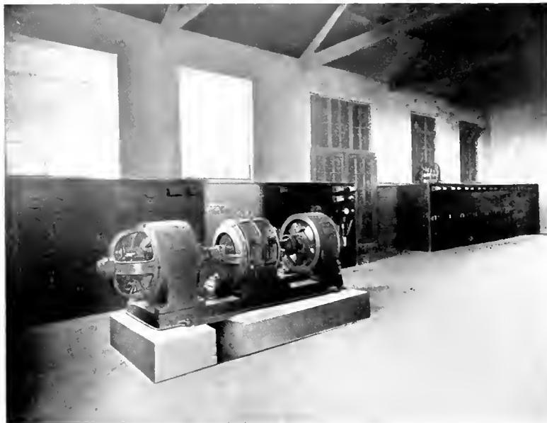
Fig. 3. 3-Unit Set for Excitation of Cogging Mill Motor and its Special Generator.
