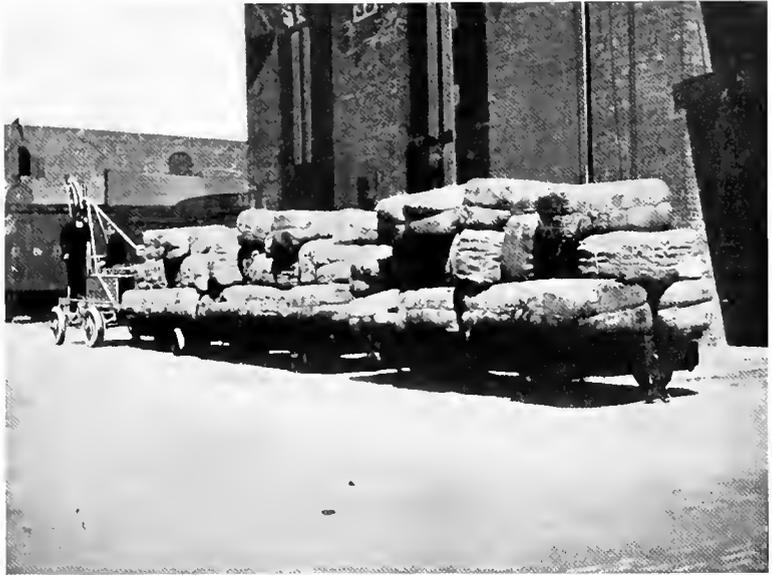
Fig. 8. Battery Truck Crane and Trailers Trafficking Between Piers, Bulkhead and Warehouses
