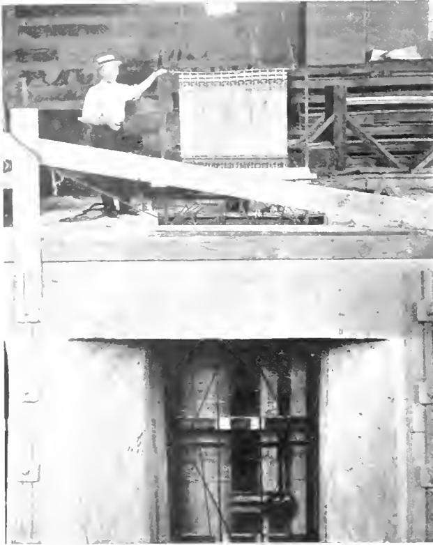
Fig. 5. Upper Portion of Moveable Framework, with Glass Reading Tubes Backed by Graduated Board
