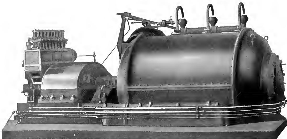
Fig. 15. Blast Furnace Turbine Compressor, Inroquois Iron Company, South Chicago
