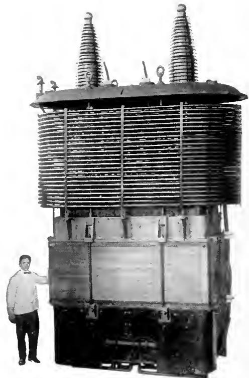
Fig. 3. 3000 Kv-a. 140,000 Volt Water-Cooled Transformer Without Case
