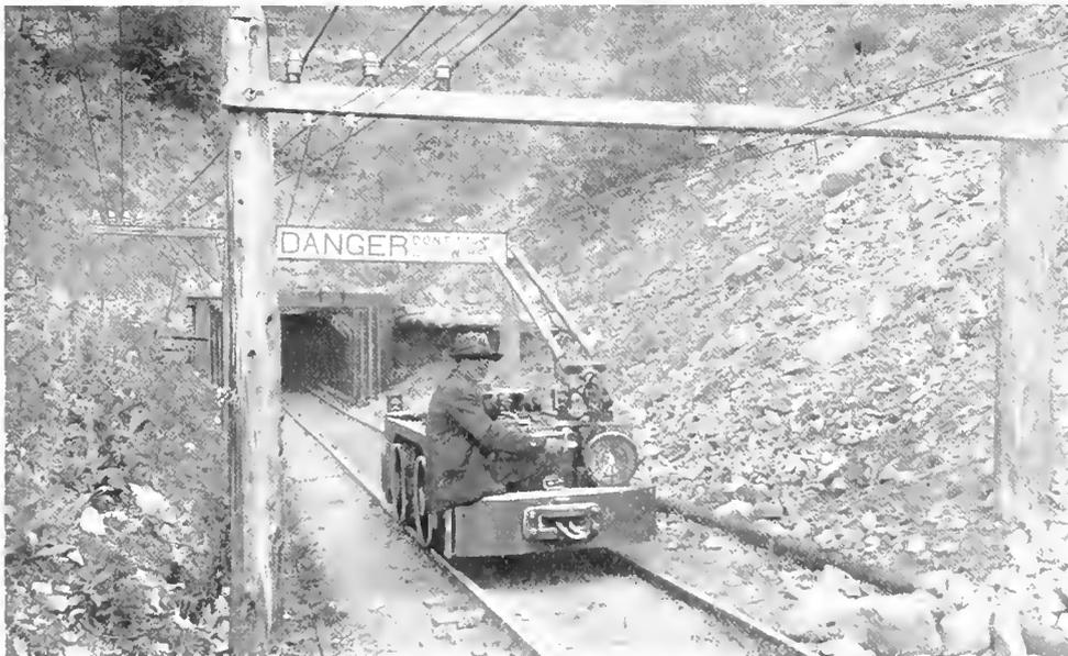
Fig. 8. Five Ton, 220 Volt Double Trolley Direct Current Locomotive at Barton Hill Tunnel
