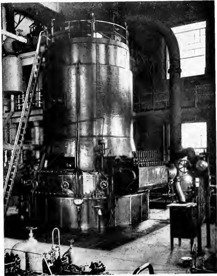
Fig. 2. 9722 Kv-a. Mixed-Pressure Curtis Turbine
