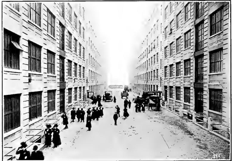
Fig. 1. The Railroads and Freight Elevators are in Alternate Streets Between the Bush Factories
