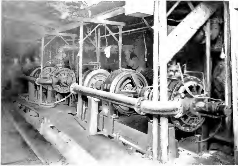
Fig. 3. Induction Motor-Driven Pumps
