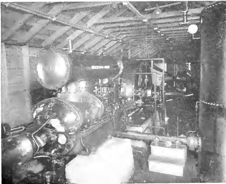
Fig. 3. 200 H.P., 2200 Volt Induction Motor Belted to Ingersoll-Rand 20 $\frac{1}{4}$ x13 $\frac{1}{4}$ x18 In. Air Compressor. Frazer Brace & Co., Shelburne Falls, Mass.
