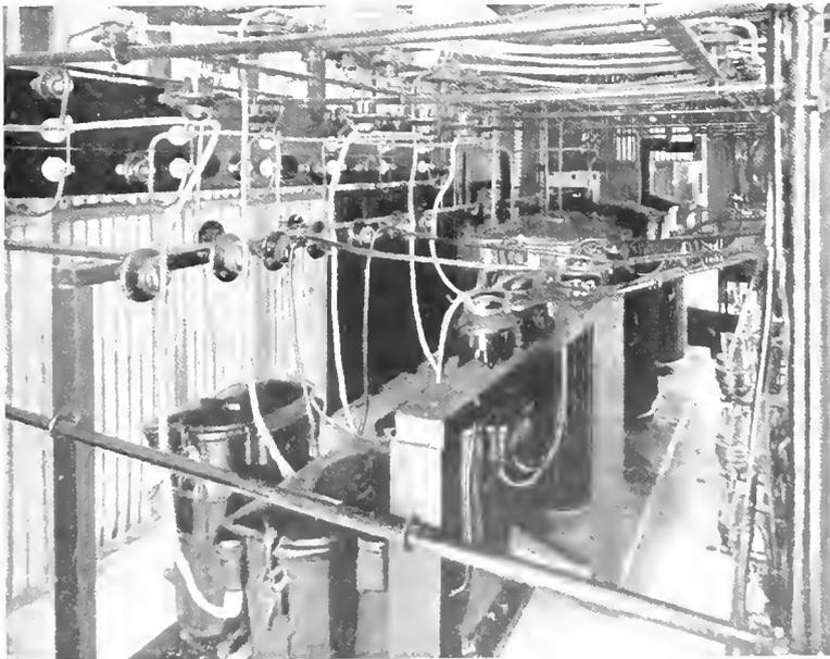
Fig. 12. Three 50 Kv-a., 6600/460 Volt Transformers for Power;
