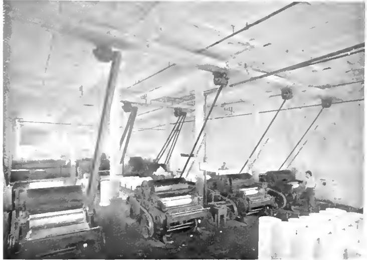
Fig. 5. Pickers Driven by Individual Motors
