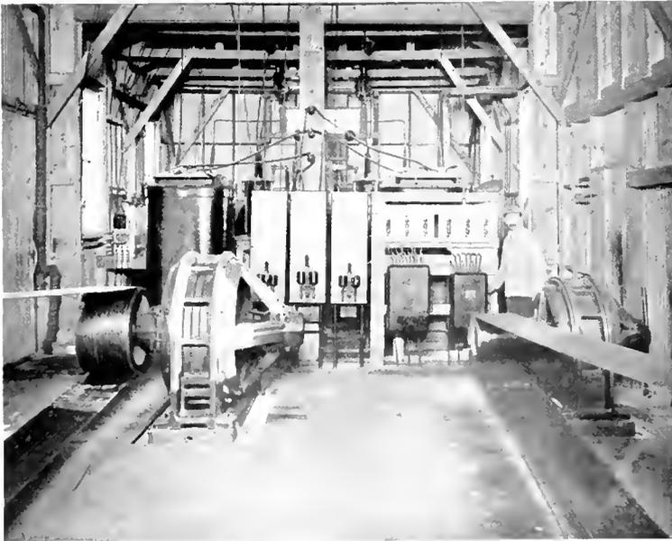
Fig. 7. Induction Motors Belted to Air Compressors
