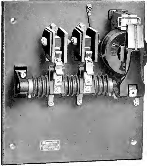
Fig. 4. Double Pole Alternating Current Contactor
