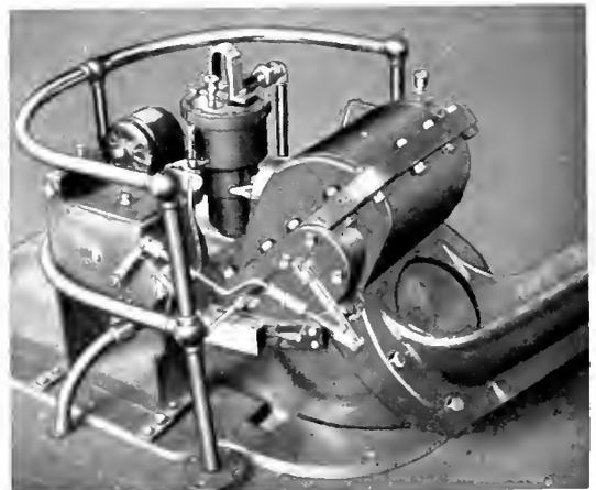
Fig. 2. Transmitter Used in Philadelphia Pneumatic Tube Mail Delivery System
