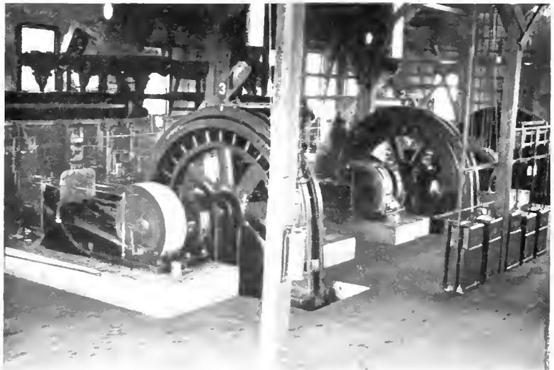
Fig. 2. 500 H.P., 2200 Volt Synchronous Motor Direct Connected to 32x20x30 In. Air Compressors. The United Engineering & Contracting Company, Barge Canal Contract 40, Lockport, N. Y.
