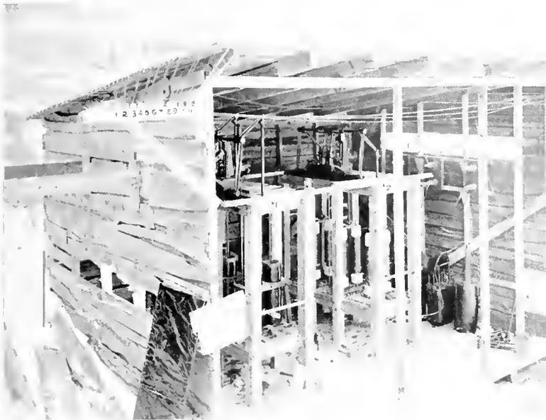
Fig. 4. Oil-break Switches Under Test Conditions Made to Represent Actual Operation
