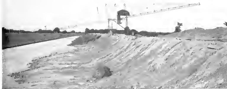
Fig. 7. Cantilever Crane Operating Drag Bucket made by Erown Hoisting Machinery Co. 225 H.P., 400 Volt Induction Motor. The United Engineering & Contracting Company, Barge Canal Contract No. 40, Lockport, N. Y.
