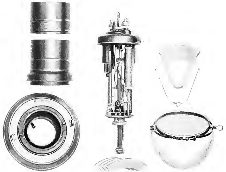
Fig. 2. Parts of Enclosed Flame Arc Lamp
