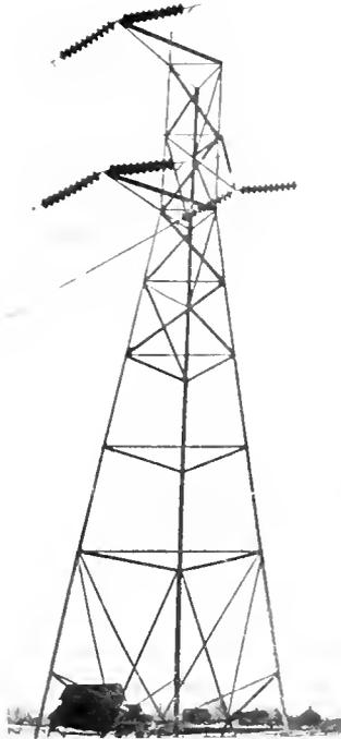
Fig. 2. 140,000 Volt Single-Circuit Strain Tower of the Eastern Michigan Power Company
