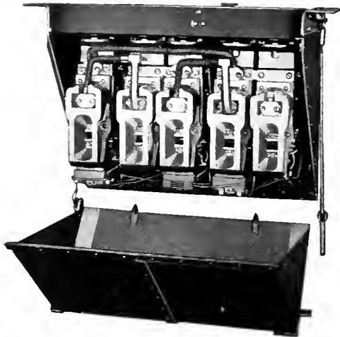
Fig. 4. Contactor Box for Ammunition Hoist Motor
