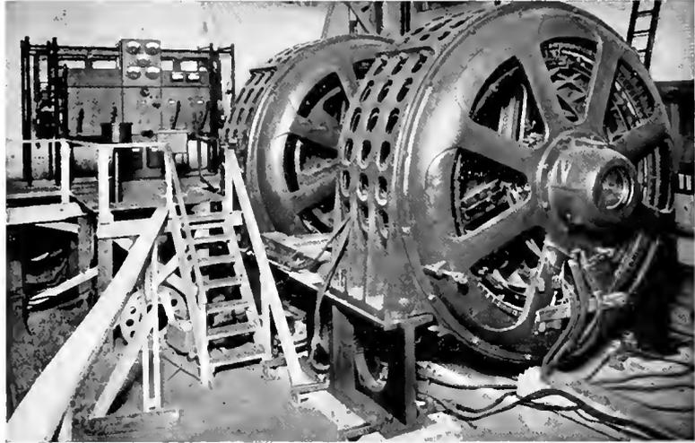
Fig. 4. Induction Motors in Testing Department of Manufacturer
