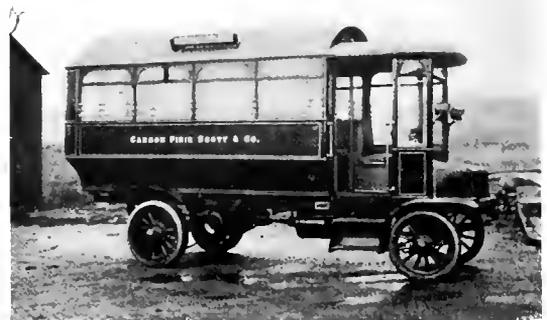
Fig. 9. Passenger Omnibus Fitted on Chassis of Fig. 8
