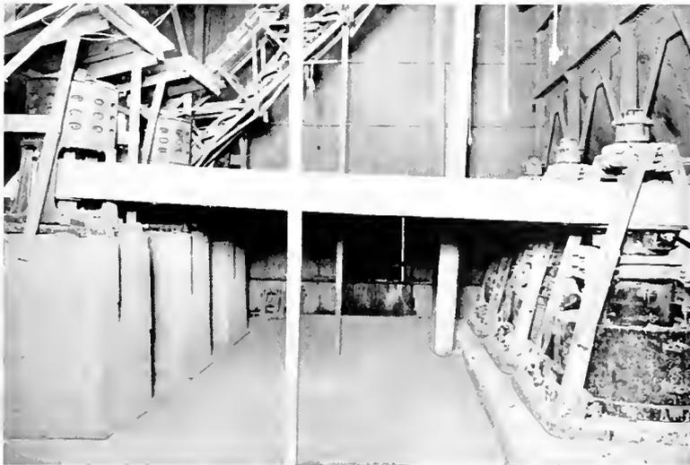
75 H.P., 400 R.P.M., 60 Cycle, Vertical Induction Motors Driving Giant Griffin Mills Knickerbocker Portland Cement Company, Hudson, N. Y.
