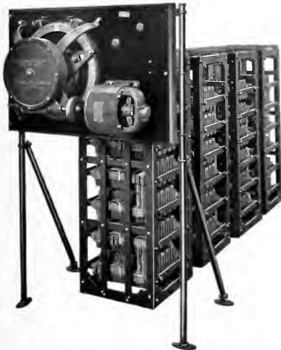
Fig. 8. Motor-operated Field Rheostat for 14,000 Kw. Turbo-alternator
