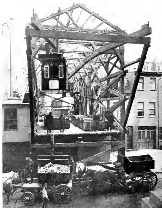
Fig. 8. Monorail Hoists Operated by One 75 H.P. and One 15 H.P. Motor. The United Engineering & Contracting Co., New York City
