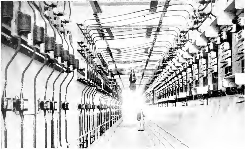
Fig. 8. Interior of Substation showing Lightning Arresters
