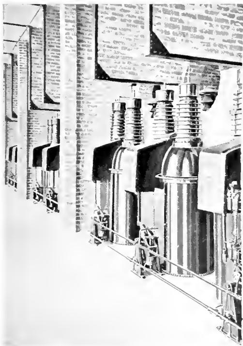
Fig. 9. Arrangement of 70,000-Volt 150 Ampere Oil-Switches
