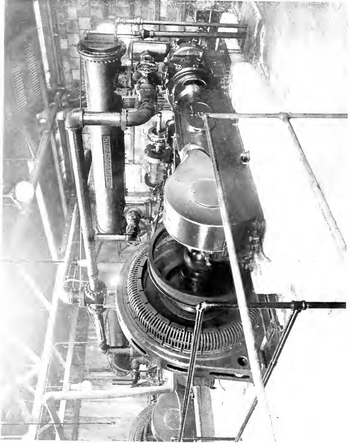
Two 137 Kv-a. Synchronous Motors Direct Connected to Two-Stage Air Compressors. Temporary Installation for Construction Work on Catskill Aqueduct, New York City
