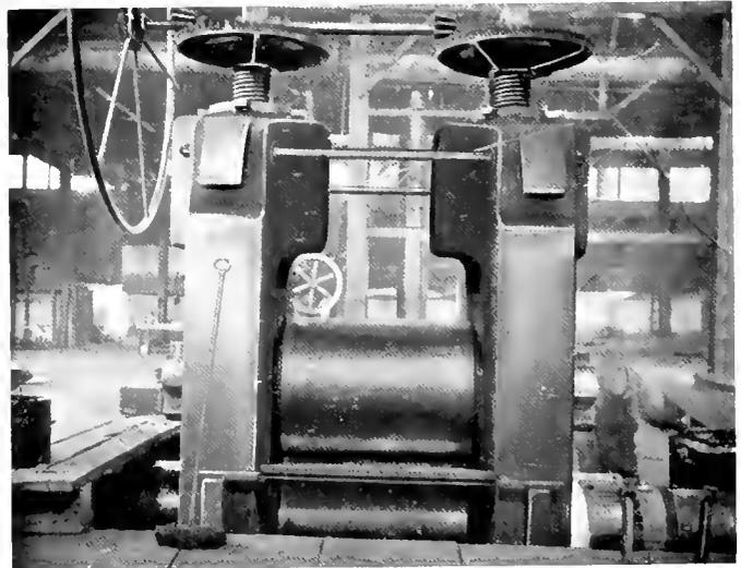
Fig. 14. One Stand of Rolls, 30 in. Sheet Mill
