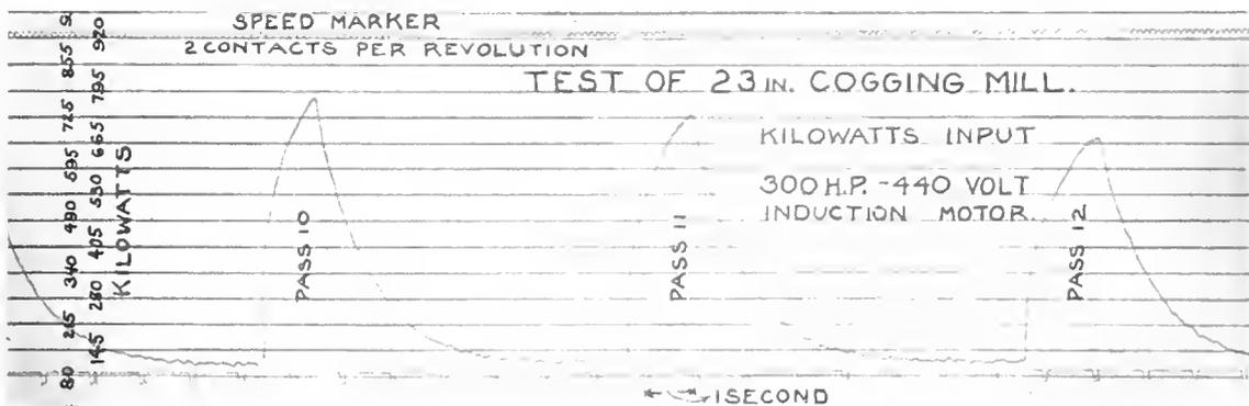
Fig. 16. Example of Insufficient Flywheel Effect
