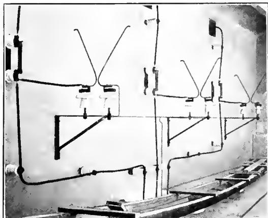
Fig. 1. Main Horn Gaps and Fuses of a European Type Lightning Arrester Installation Located in Mexico
