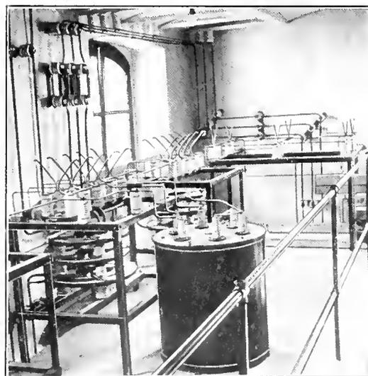
Fig. 2. Main Floor Arrester Equipment of the Mexican Plant. Multiple horn gaps and choke coils at the left, delta connected horn gaps at the right, and oil tank containing resistance in the foreground
