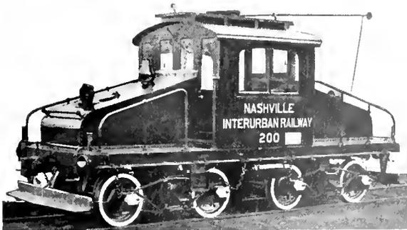
Fig. 1. 25-Ton Electric Locomotive, Nashville Interurban Railway
