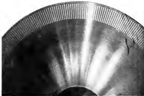
Fig. 4. Rotor of Standard 100,000 Cycle Alternator
