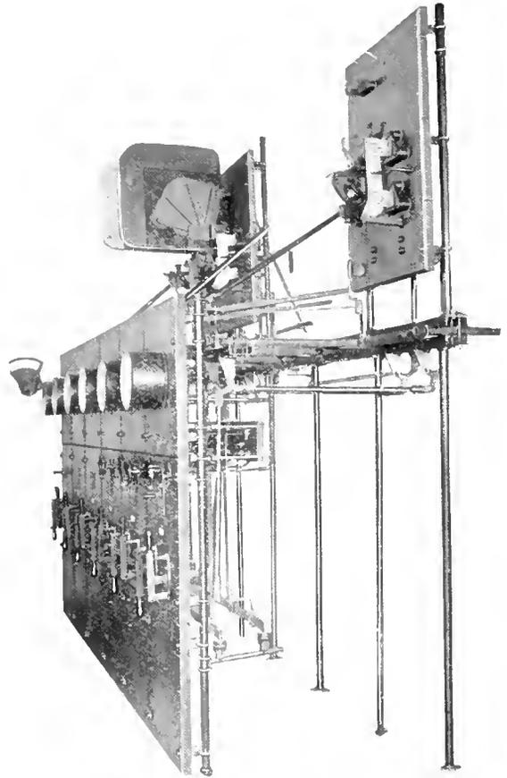
Fig. 4. Switchboard for 2400 Volt D.C. Substation
