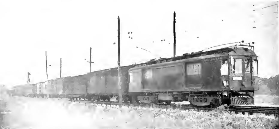
Box Car 1 Locomotive Hauling Train of Freight Cars on Washington, Baltimore & Annapolis Electric Railway. Locomotive with Four 125 H.P. 600 1200 Volt Motors (GE-207) and Sprague G-E Type M Control
