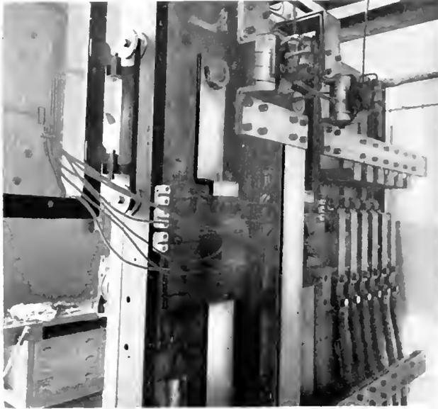
Fig. 9. Back View of the Switchboard Shown in Fig. 8. Main Reverse Current Relay in the Upper Right Hand Corner
