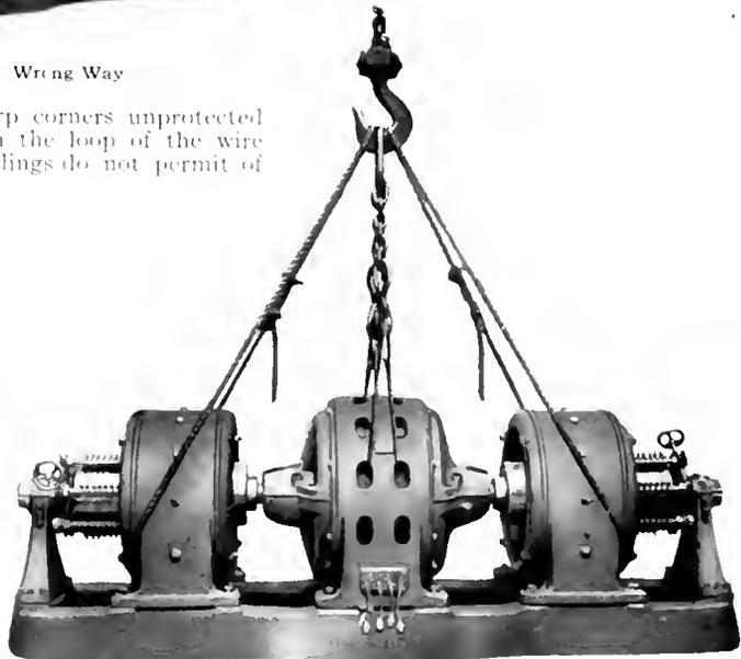
Fig. 33. Lifting Motor-Generator Sets Right Way.
