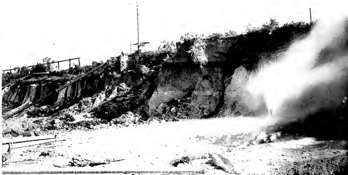
Fig. 1 Removing the Overburden. Placed under a pressure of 100 to 150 lbs. by reciprocating pumps, a stream of water is directed at the face of the quarry by nozzles or guns. These nozzles are from 1 to 1½ inches in diameter
