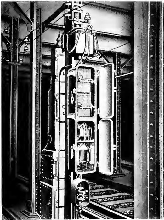
Fig. 7. Typical Instrument Case, New York City Subway
