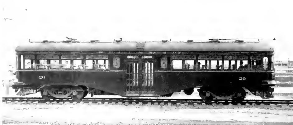
Center Entrance Interurban Car, Kansas City, Clay County & St. Joseph, Equipped with Four 100 H.P. 600 1200 Volt Ventilated Motors (GE-225) and Sprague G-E Type M Control
