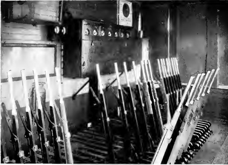
Fig. 2. Mechanical Interlocking Signal Plant
