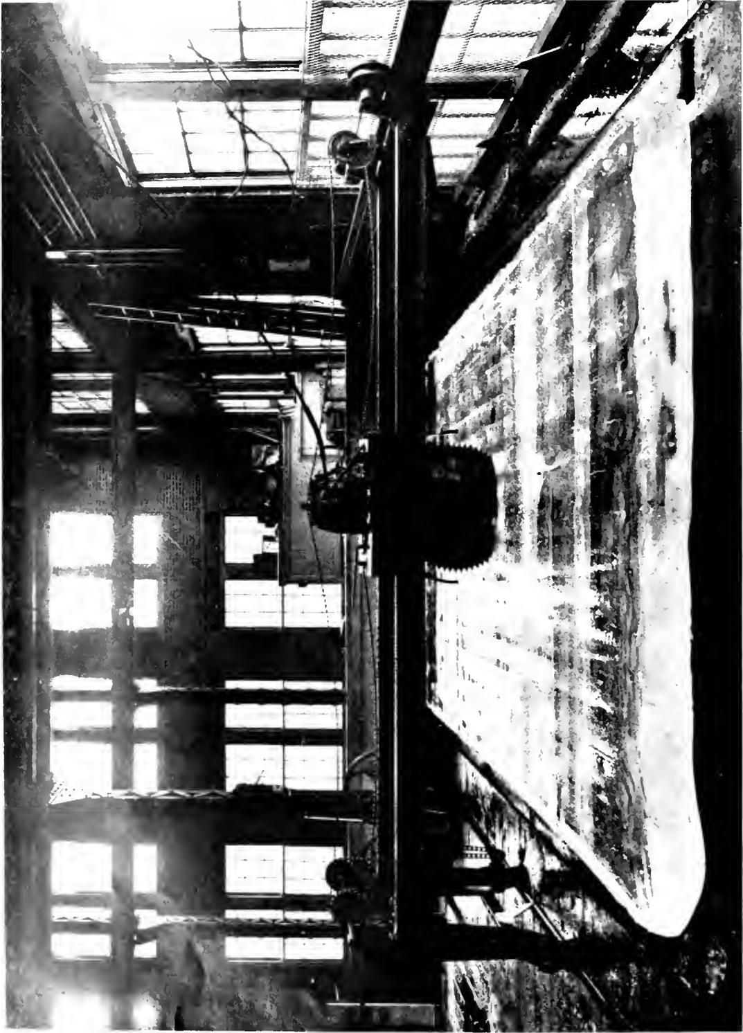
CUTTING A FOUR-TON CAKE OF ARTIFICIAL ICE BY MOTOR-DRIVEN SAW
