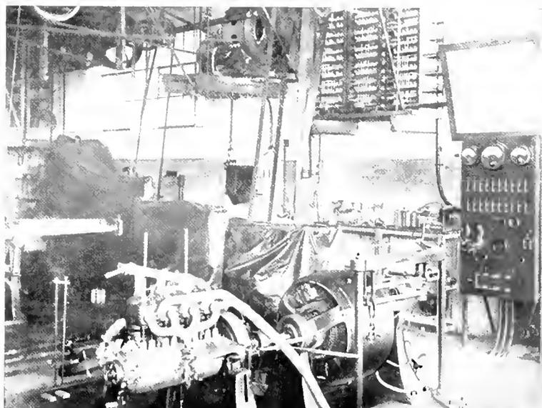
Fig. 3. Testing Laboratory of Large Automobile Factory Equipped with Electric Dynamometer. Willys-Overland Co., Toledo
