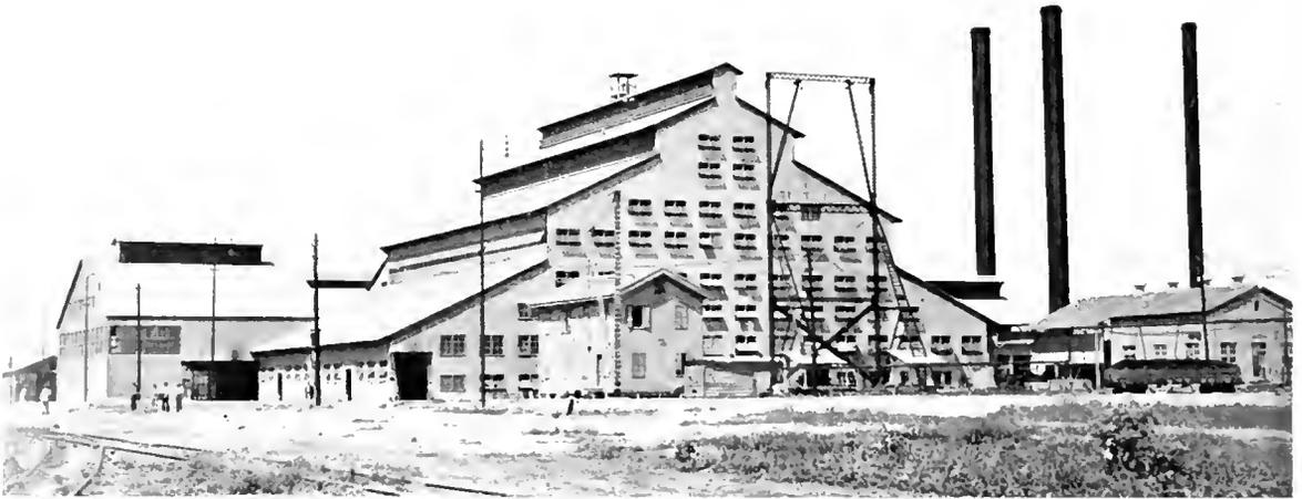
This is a view of the sugar mill and power house of the San Manuel Sugar Company, Las Delicias, Cuba. The raw cane is delivered direct into the "central" by the railroad, and is there subjected to a succession of processes of extraction and refining, in all of which electricity is very profitably employed. The power house is shown on the right of the picture, and derives the bulk of its fuel supply from the "bagasse" or cane from which the juice has been extracted
