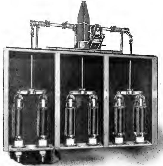
Fig. 4. Motor-Operated Oil Switch with Oil Vessels in Tandem
