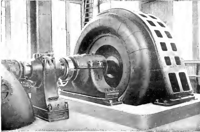
Fig. 3. A 8750 Kw., 6900 Volt Generator, Ventilated Entirely by Air Drawn in Around the Shaft and Expelled Into the Room Again, Through Holes in the Frame Above Base Line. No Openings to the Pit
