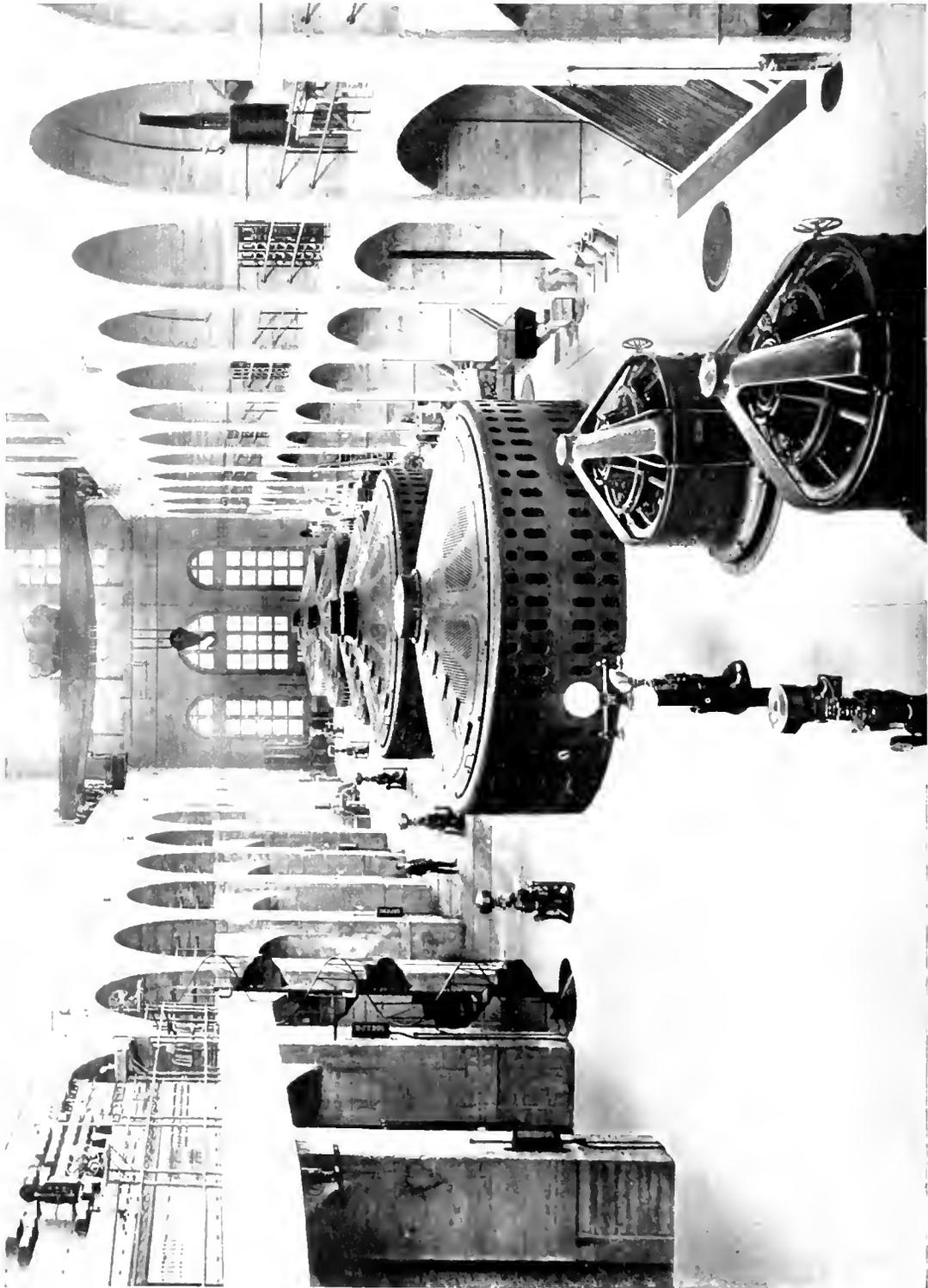
Interior of Holtwood Station of the Pennsylvania Water & Power Company, showing two 400 kw. vertical exciters and three 7500 kv.-a. and two 10,000 kv.-a. vertical waterwheel generators. The generators operate at 94 r.p.m. and deliver three-phase current at 25 cycles, 11,000 volts. Initial capacity of station 42,500 kv.-a.
