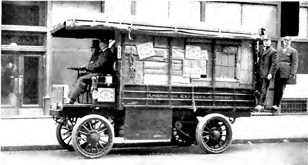
Fig. 2. The Electric Truck is Widely Employed by Express Companies on Account of Its High Economy on Frequent-stop Runs
