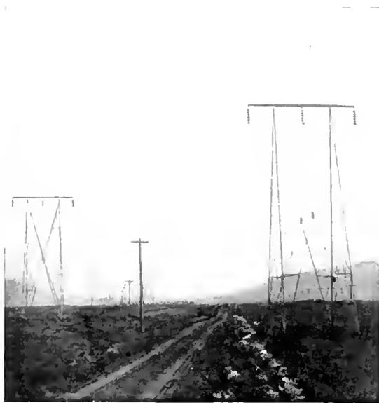
Fig. 6. Double-Circuit Double-Tower Line, Great Falls Power Company
