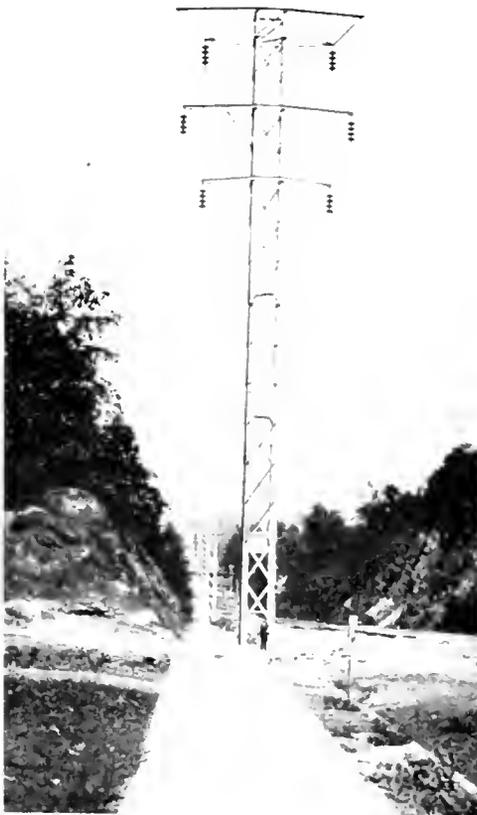
Fig. 2. Latticed Steel Pole on Lines of the Central Georgia Power Co. Note the Staggered Arrangement of Conductors on Each Circuit
