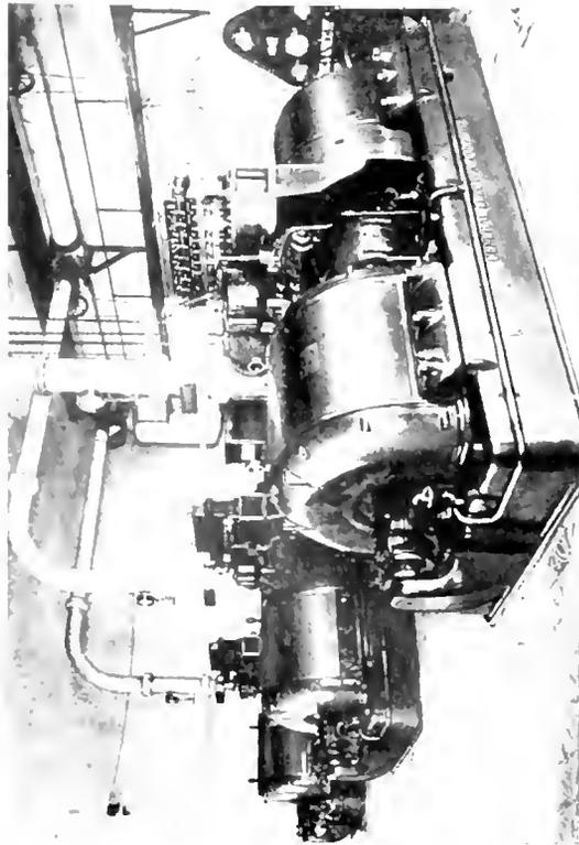
Installation of three 1000 kw. Curtis turbo generators running at 3600 r.p.m. and delivering current at 440 volts, 60 cycles for power and lighting loads in the San Manuel Company's plant. The San Manuel installation was designed for electrical operation, and is now completing its second successful grinding season.
