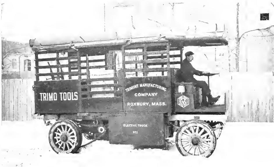
Fig. 1. Storage Battery Truck Used in the Service of a Tool Manufacturer. Power propelled vehicles are able to easily overcome bad road conditions, such as snow, etc.
