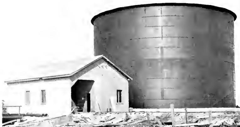
An adjunct to the sugar central. Molasses or "miel" tank and pumping station at the plant of the San Manuel Sugar Company, Las Delicias, Cuba
