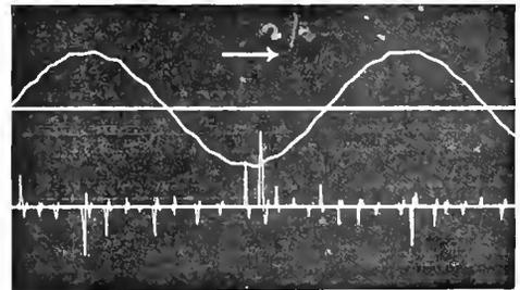
Fig. 32. Charging current of an aluminum arrester when there was a small gap in series (lower record). A current transformer was used, a single impulse giving a complete cycle of oscillations in the oscillogram. Delta potential, 13,200 volts, is shown in the upper record
