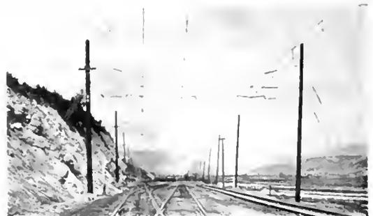
Fig. 6. Catenary Suspension, 2400 Volt Trolley
