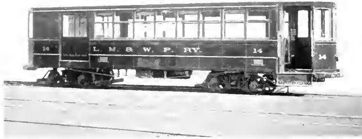
Fig. 4. Storage Battery Car on Lewisburg, Milton & Watsontown Passenger Railway
