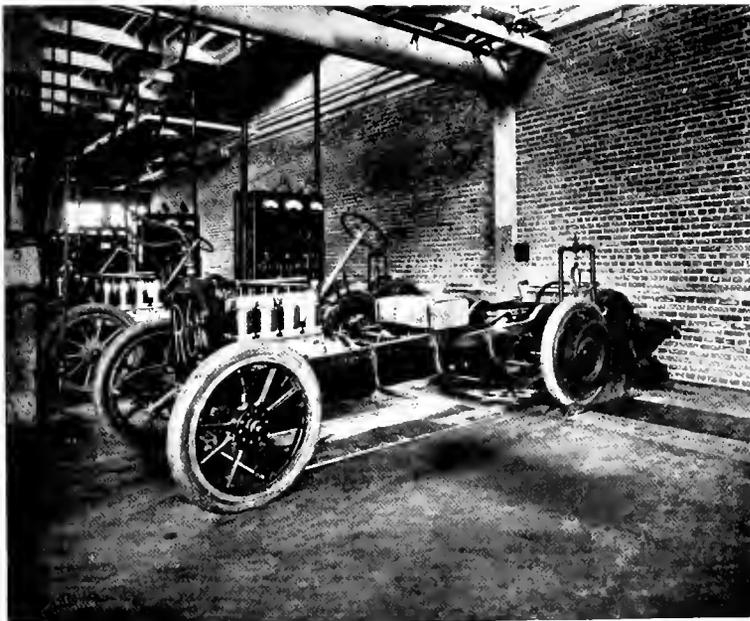
Fig. 7. Chassis-testing Dynamometers in the Plant of the Cadillac Motor Car Company, Detroit
