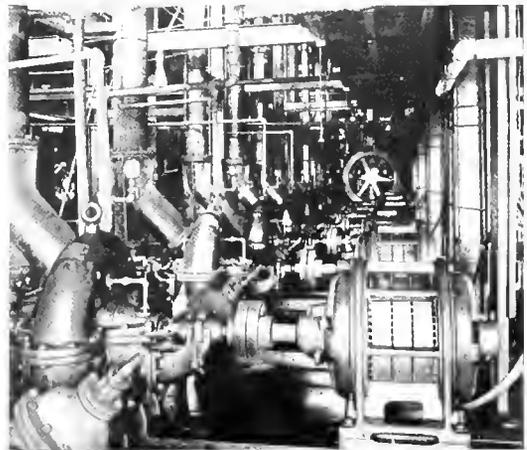
There are frequent applications of the centrifugal pump in the modern sugar central. All the above motors are three-phase induction machines running at 1800 r.p.m. five of them being rated at 50 h.p. and two at 35 h.p. Each is direct-connected to a centrifugal pump, there being a separate one for each vacuum pan and quadruple effect. Capacity 1400 gallons, 1800 gallons and 2000 gallons per minute
