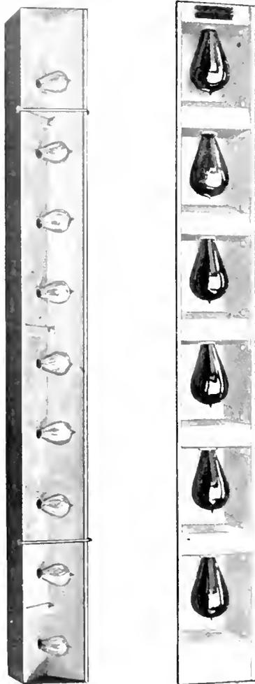
Fig. 1. Lamps and Reflectors Which are Placed Along the Sides of the Proscenium Arch
