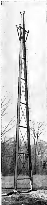
Fig. 8. Flexible Steel Tower on Lines of Rochester and Sodus Bay Power Co.
