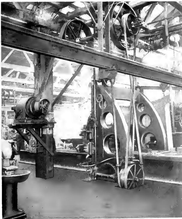
Fig. 9. Planer, 72 in. by 22 ft., belt driven, by a 40 h.p. 1060 r.p.m. Compound Wound Motor
