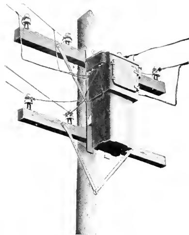
Fig. 15. Automatic Feeder Voltage Regulator on Pole
