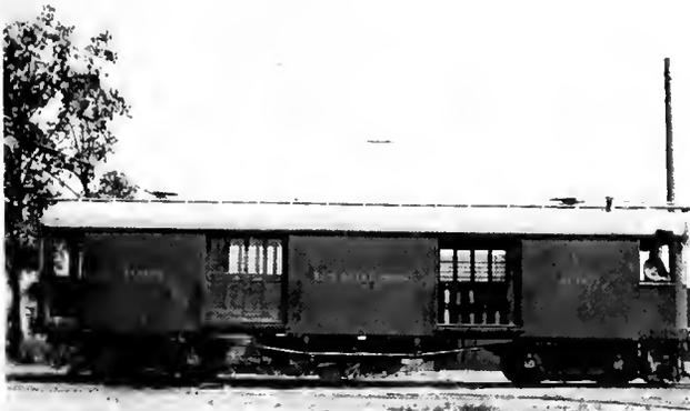
Express Car, Gary & Interurban Railway Company, Equipped with Four 100 H.P. Motors and Sprague G-E Type M Control
