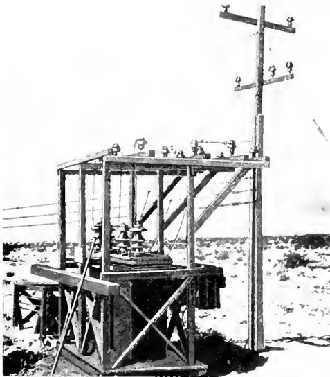
Fig. 23. Three 20 Kv-a. Outdoor Transformers in Irrigation Service
