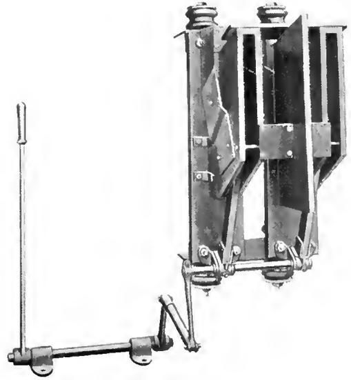
Fig. 5. Hand-Operated Main Switch, 2400 Volts
