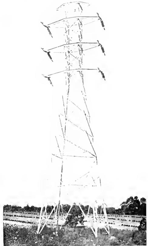
Fig. 9. Intermediate Strain Tower, Pennsylvania Water and Power Company
