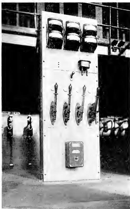
Fig. 3. Front View of the Switchboard Located in the Controlling Substation Showing the Starting and Running Switches for the Converter of the Distant Automatic Substation
