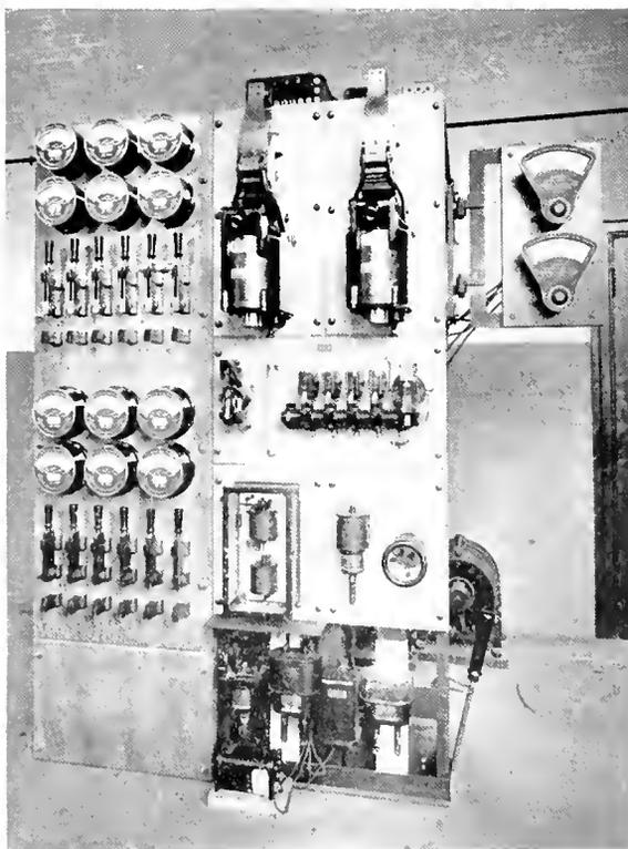
Fig. 8. Front View of the Switchboard in the Rowena Street Substation Showing the Automatic Control Device at the Right and Feeder Panel at the Left
