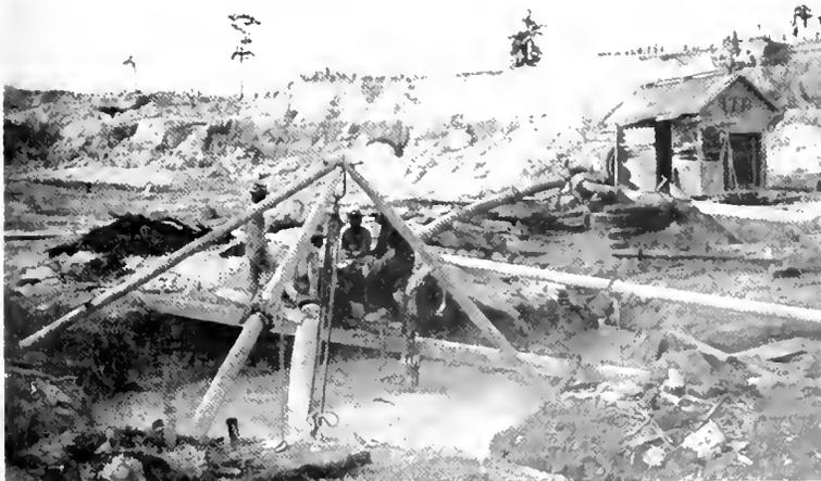
Fig. 2. At some place near the center of the field is located the sump-hole, about 8 feet square, around which the guns work, washing the material to the bottom of the pit
