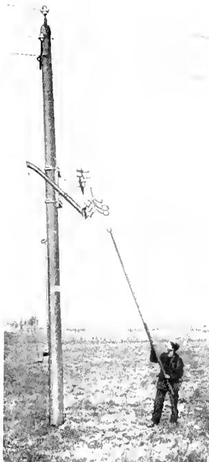
Fig. 27. Pole Line Disconnecting Switch and Temporary Connections for Supplying Power to Transmission Wagon Shown in Fig. 26 for Power Supply on Farm
