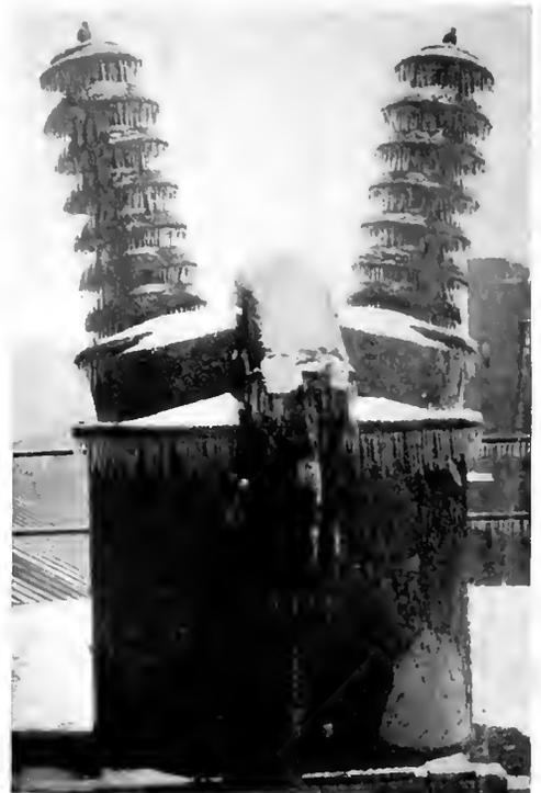
Fig. 12. Single-Pole Oil-Switch on 110,000-Volt Circuit After a Sleet Storm
