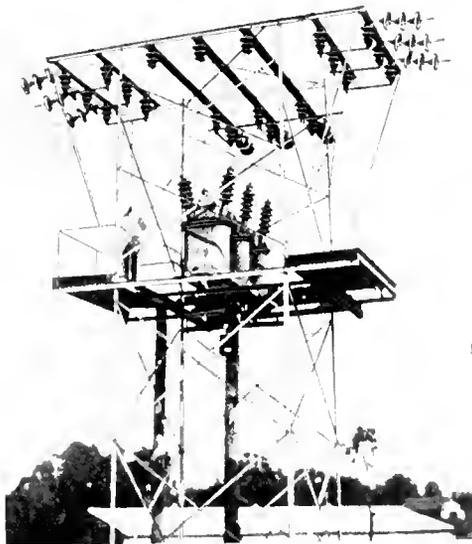
Fig. 20. 44,000-Volt Switching Tower at Mooresville, N. C.
