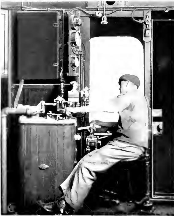
Fig. 8. View Showing Position of Operator and Controlling Apparatus on Self Propelled Car with Electric Drive
