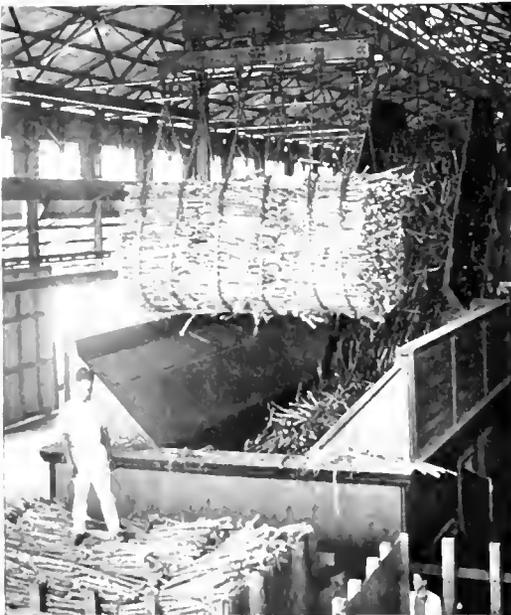
Handling the cane at the central. The hoist shown here (San Manuel Company) is operated by a 30 h.p. induction motor
