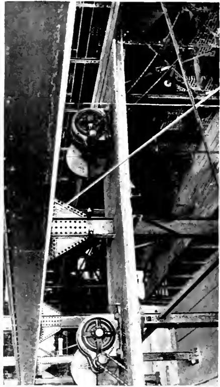
Raising steam from the refuse of production. The "bagasse" is used as fuel in the steam electric plant, and the above picture shows two 15 h.p., 900 r.p.m. motors driving, through back gearing and chains, the "bagasse" feeders corresponding to the boilers on each side.
