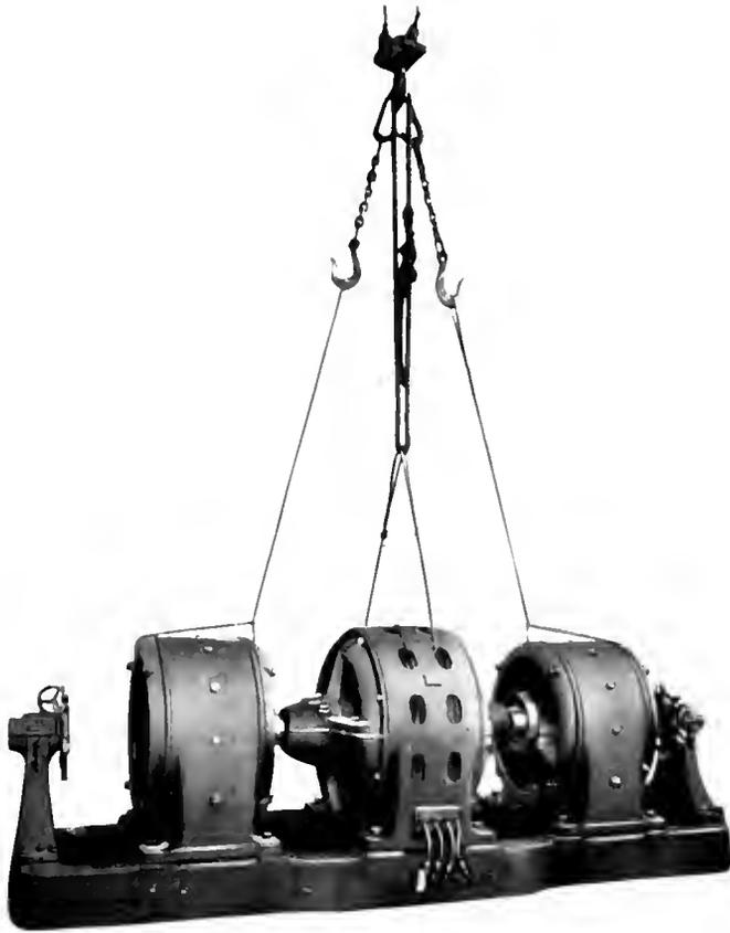
Fig. 32. Lifting Motor-Generator Sets Wrong Way
