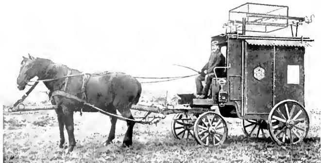
Fig. 26. Transformer and Switching Wagon Mounted on Horse Drawn Vehicle
