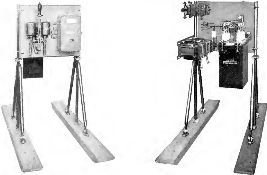
Figs. 16 and 17. Front and Rear Views of Switchboard Cabinet Panel for 2300-Volt Distribution to Rural Consumers. The panel is provided with oil-switch and watt-hour meter for controlling and metering the distribution of 25 kv-a. of three-phase load. These panels are installed in a housing of wood or steel, as desired, and are then mounted on pole or tower as indicated in outline sketches shown in the early part of article
