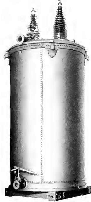
Fig. 1. A 3333 Kw., 110000 11000-Volt Water-Cooled Transformer For Outdoor Use
