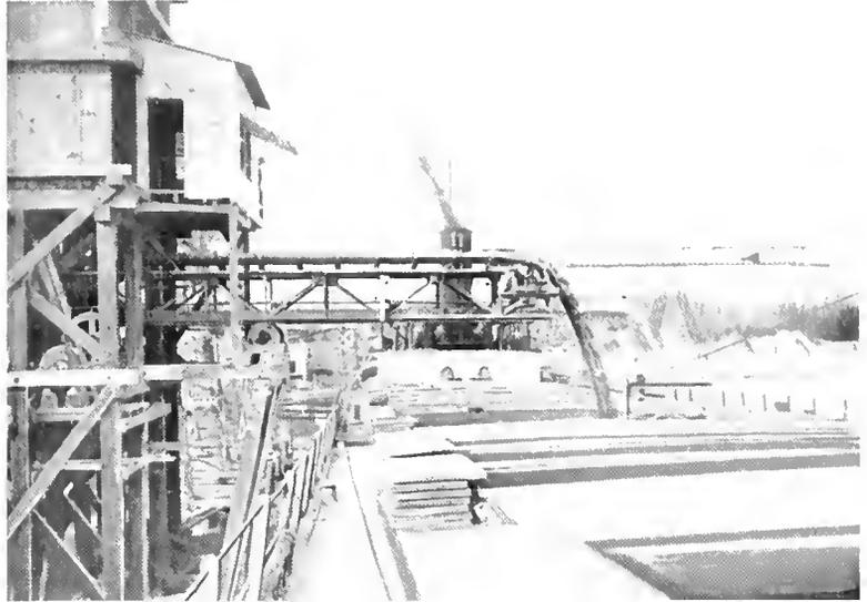
Shuttle Conveyor, Driven and Adjusted by Two 20 H P., 220 Volt Induction Motors, Delivering Flux Stone to Ship
