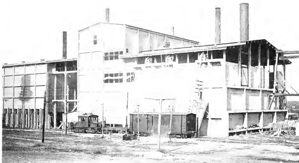
Fig. 5. Drying equipment at the quarry of the Prairie Pebble Phosphate Company. One drying plant will usually take care of all the material from several different washers, and both electric and steam locomotives are used for transporting the rock
