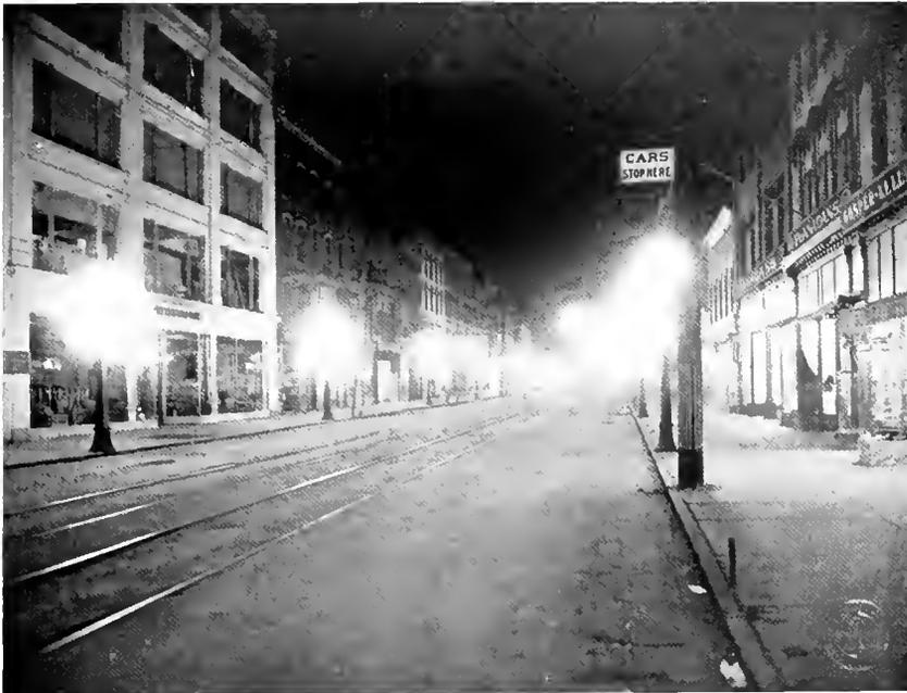
Fig. 3. Night View Taken on Water Street, Elmira, N. Y., Showing Well Distributed and Even Illumination. The Uniformity of Illumination and the Absence of Any Deep Shadows on Either the Road or Side Walk is Very Noticeable. The Lighting in this Instance is Effected by Series Tungsten Filament (Mazda) Lamps. There are Three 80 Candle-Power Series Lamps on Each Standard Taking 6.6 Amperes. The Lamps are Spaced 60 Ft. Apart
