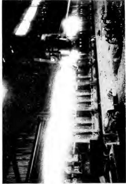
Fig. 5 Pouring side of Open Hearth, showing 125-ton Ladle Crane Filling Ingot Mold
