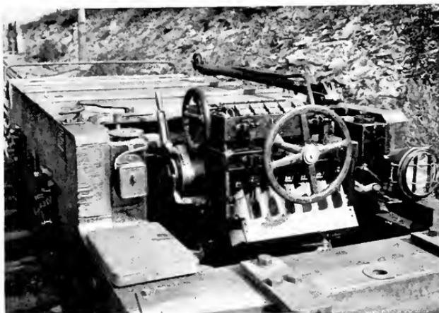
Fig. 16. Locomotive Equipped with HC Control with Covers Removed to Show Arrangement of Contactors
