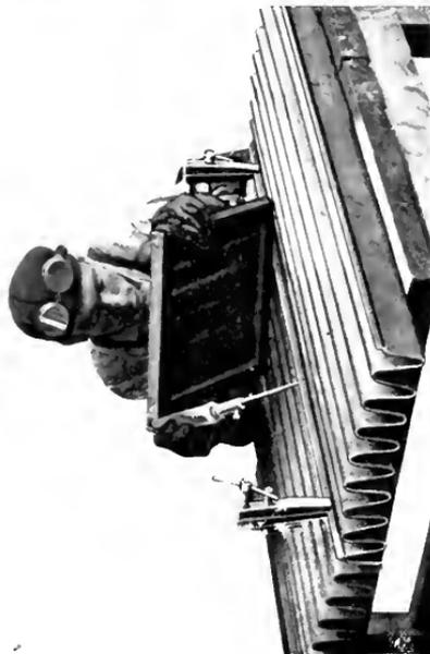
Fig. 15. Seam Prepared for Hand Welding with Carbon Electrode and Operator in the Position for Welding
