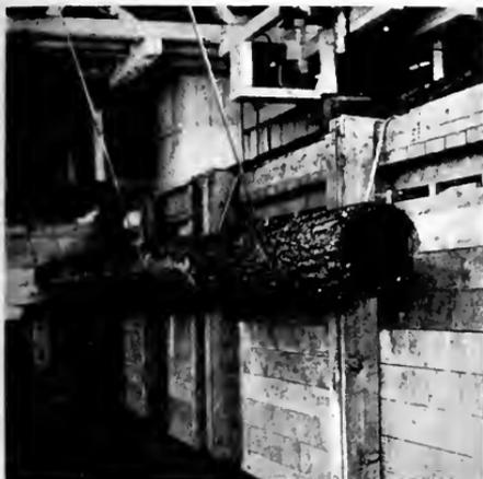
Log Hoist Driven by a 52-h.p., 600-r.p.m., 440-volt Varying Speed Motor. Booth-Kelly Lumber Company.
