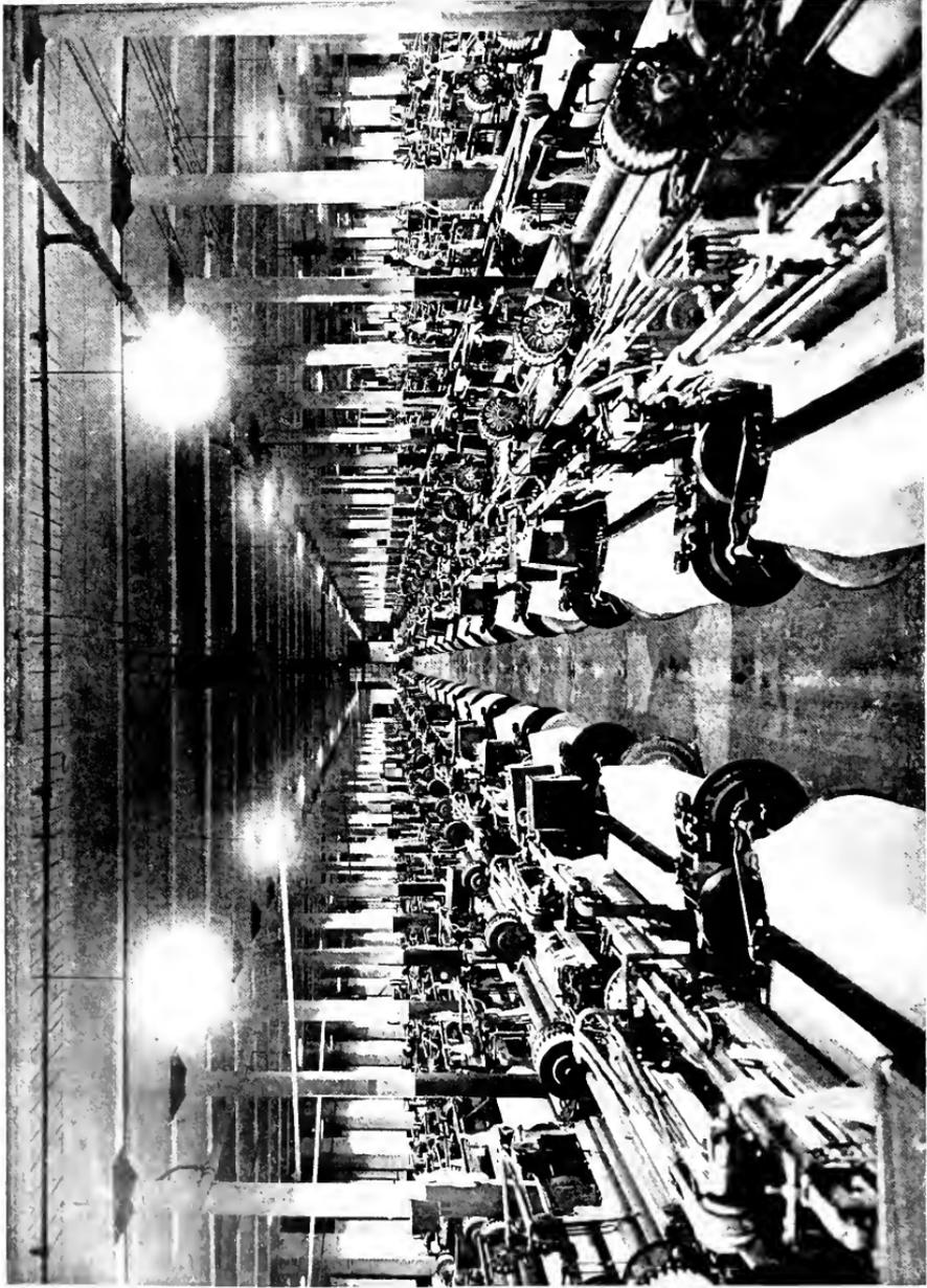
A Few Years ago Looms Were Usually Lighted by Small Incandescent Lamps in Deep Bowl Reflectors, Hung Close to the Weavers. These are hung high, well out of the ordinary angle of view, and provide evenly distributed general illumination. This system makes the room feel more cheerful and all parts of the machines are rendered clearly visible. This weave shed is lighted by 100-watt Mazda C lamps in enamel dome reflectors, hung 12 feet high on casters 12 by 22 ft. (See articles pages 674 and 681.)
