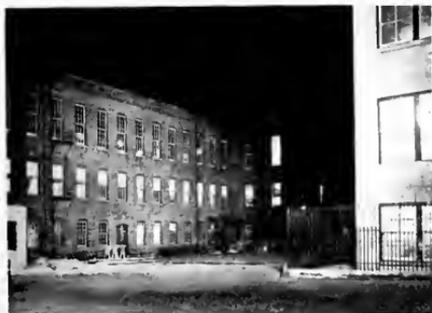
Fig. 93. Factory Yard Flood Lighted for Night Protection by One G-E Floodlighting Projector Equipped with 400-watt Edison Mazda "C" Floodlighting Lamp
