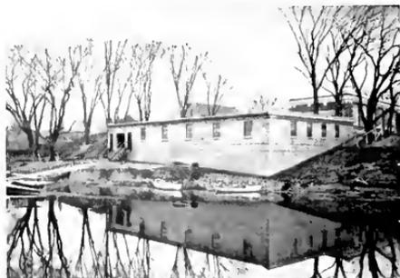
Fig. 5. The Concrete Boathouse on the Banks of the Mohawk River in the Rear of Edison Club and Hall. A double track is provided for running the 200 canoes in and out of the fireproof boathouse
