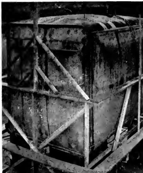
Fig. 23. Electrically Welded Box Constructed for Experimental Purposes for the Electric Welding Committee of the Emergency Fleet Corporation. Box Under a Hydrostatic Pressure Test of 40 lb. Per Square Inch. Note bulging of plates
