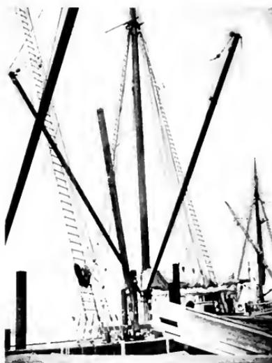
Fig. 9. Long Timber Suspended in Position Preparatory to Lowering
