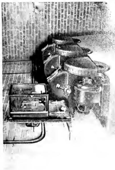
1 h p. G. E. Motor Driving Electrically Winkles, Roller and Lower Furnace
