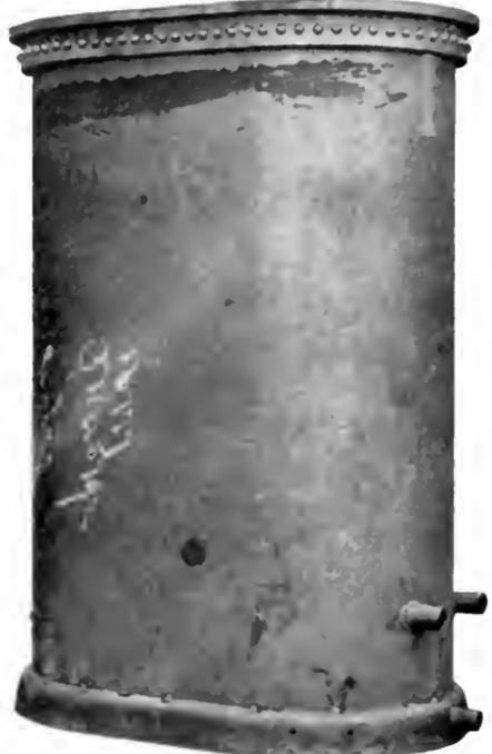
Fig. 10. Shows Base and Shell of Tank Tacked and Welded. Ready for Welding. The shell plate is beveled on one side and the distance between it and the base is 1/2 inch. This arrangement enables the welder to weld through and provides breathing space as the welding progresses. As the welder approaches the tacks they are driven away by the movement of base and free it from unnecessary tacking. When the welding is finished the bottom line of base is irregular. The base is afterward cut square.
