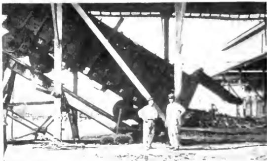
Hydraulic Car Unloader, Central Mercedes. A motor-driven centrifugal pump replaced the steam pump for supplying the water.
