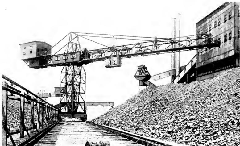
Fig. 27. High Speed A.C. Hammer Head Coal Handling Gantry Cranes
