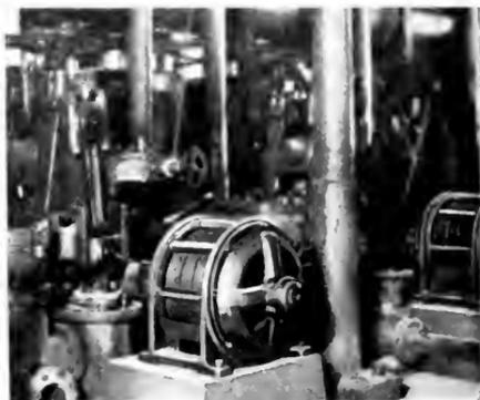
15-h.p., 600-r.p.m. Motors Geared to Triplex Plunger Molasses Pumps. Central Mercedes
