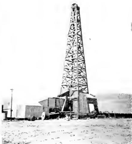
Fig. 2. One of the Heaviest Derricks in the World, in the Coalinga Field, California. Height 106 ft. Depth of well 4200 ft.
