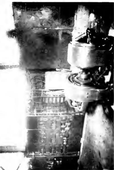
Fig. 12 Motor Rectifier, Slip Regulator, and Control Panel for Starting the Flywheel Motor generator, Fig. 11
