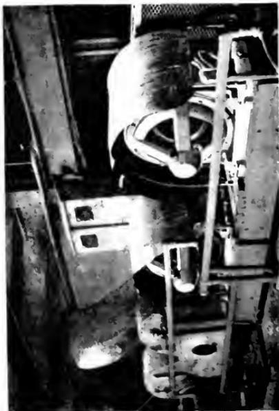
50-h.p. Motors Driving Bluest Pans in Lime Kiln Solvay Process Company, Syracuse, N. Y.
