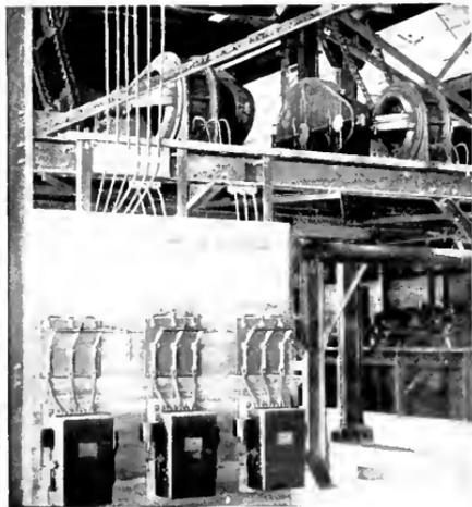
25-h.p. Back-gear Motors Driving Main Bagasse Conveyors, Central Delicias. The motors are mounted directly under the conveyor while the starters are on the operating floor below
