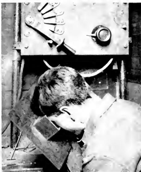
Fig. 9. Improper Distance at which to Hold the Electrode from the Work
