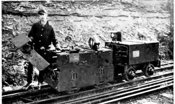
Fig. 18. 2-ton, 20-inch Gauge Storage Battery Locomotive with Battery Carrying Trailer
