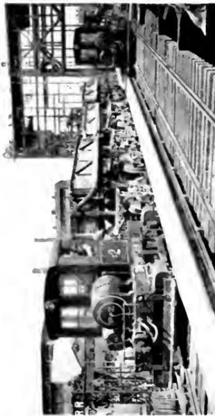
Electric Locomotive Handling Pyrites at Sulphuric Acid Plant of Davidson Chemical Company, Baltimore, Md
