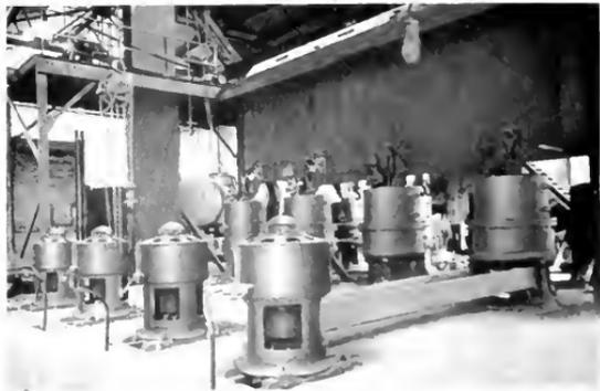
The Pulverizers, which are grinding the rock in this installation, are of a type most commonly used for pulverizing coal.
