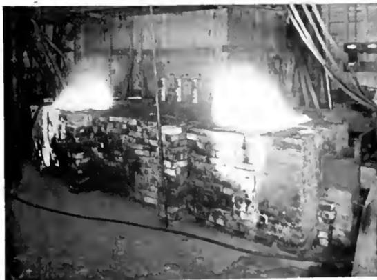
Fig. 3. Resistance Furnace in Operation, Making Special Carburides. The flames show gases burning above contact area between electrodes and charge
