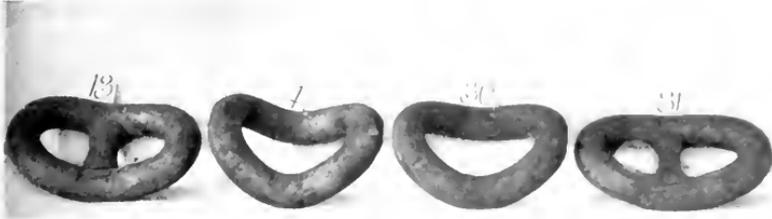
Fig. 6. Wrought-iron and Electric Cast-steel Links which Have Been Subjected to an Impact Test Under a Drop Hammer
