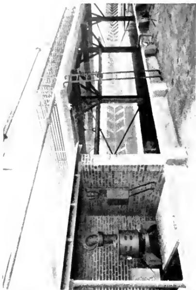
Fig. 14 20-h p., 1000-r.p.m. Vertical Induction Motor driving a Circulating Water Pump Serving the Cooler at the Right. Los Alamitos Sugar Co., Los Alamitos, Cal.
