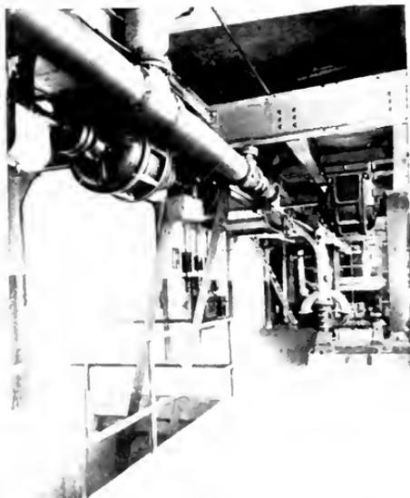
Fig. 8. 30 h.p., 750 r.p.m. Squirrel-cage Motor with Double end Connection Driving Pulp Pumps. A pump is shown to the right driven by a 20 h.p., 1000 r.p.m. squirrel-cage motor also suspended from the ceiling. American Beet Sugar Company, Chino, Cal.
