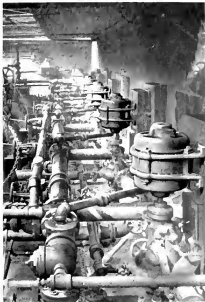
Electric Motor-driven Pumps in By-product Recovery Plant of Sargent & Lundy Co., Detroit, Mich., Which Produces Raw Material for Dye Manufacture.
