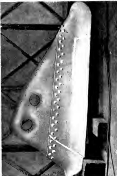
Fig. 8. Steel Plate Riveted to Casting, the Seams Being Closed by Arc Welding.
