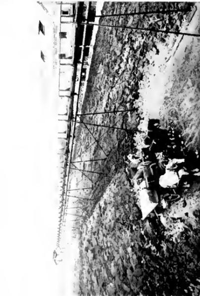
Fig. 15 Pulp Silo showing the Outgoing Pulp Line, the Strainer, Tower and the Return Water Pipe. Los Alamitos Sugar Company, Los Alamitos, Cal.
