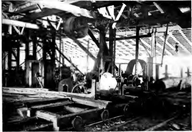
50-h.p. Motor Driving a Rip Saw and a 25-h.p. Motor Driving a Planer and Woodworking Tools in the Carpenter Shop. Central Delicias
