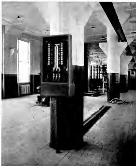
Fig. 24. Standard Lighting Panel Board
