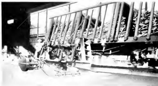
Motor operated Side Tilting Car Platform, Centra, Ulaeas, Cuba. The control is located on the opposite side with the operator.
