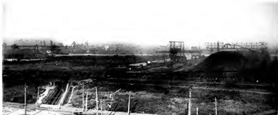
Fig. 5. View of Coal Storage Pile at South Chicago. Both steam and electrically operated unloaders and electrically operated stocking bridge are shown. There is sufficient storage area to care for 300,000 tons of coal
