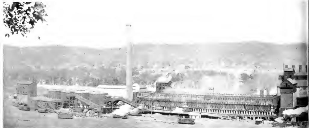
Fig. 4. Panoramic View of a Two-block By-product Coke Oven Plant. Several modern plants
