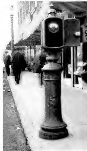
Fig. 7. Control Pedestal for 100-kv-a., 550-volt, 60-cycle, Three-phase Subway Static Condenser. Lynn Gas & Electric Company
