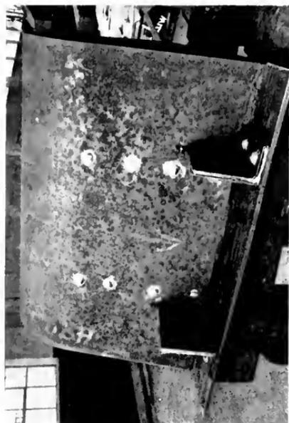
Figs. 10 and 11. Section of Submarine Ballast Tank Prepared for Electric Welding
