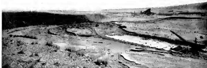
Fig. 2. General View of Tesla Creek Channel, showing Electric Drag-line Excavator in the Foreground, Railway Running to Washing Plant in the Distance and Storage Piles in the Vicinity of Washing Plant. The flat level country of the San Joaquin Valley is seen in the background
