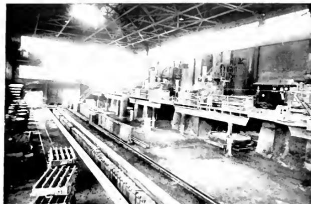
Fig. 6. An Up-to-date Electric Furnace Installation for Producing High-grade Tool Steels. The present equipment consists of four 6-ton furnaces, each taking 1500 kw.
