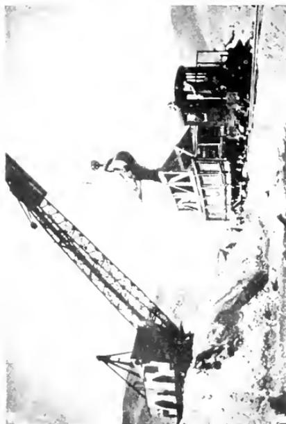
Fig. 3. Electric Drag line Excavator Loading Grizzly Car with Electric Locomotive in Foreground. Two members of the track gang may be seen grading and laying track just ahead of the grizzly car.
