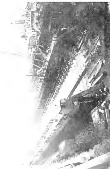
Fig. 1 Floating Dry Dock of the Bethlehem Shipbuilding Corporation, Showing Five 46-h p. Vertical Totally Enclosed Induction Motors and Control House on Each Wing of the Dock
