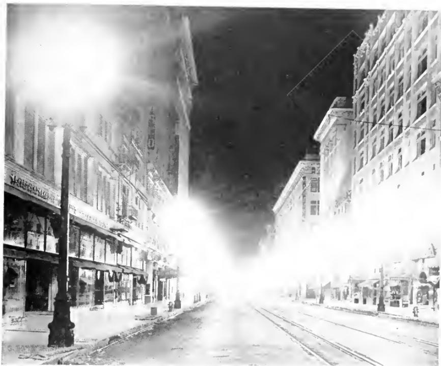
Fig. 1. Broadway, Los Angeles, Cal., Intensively Lighted by 6.6-amp. Luminous Arc Lamps
