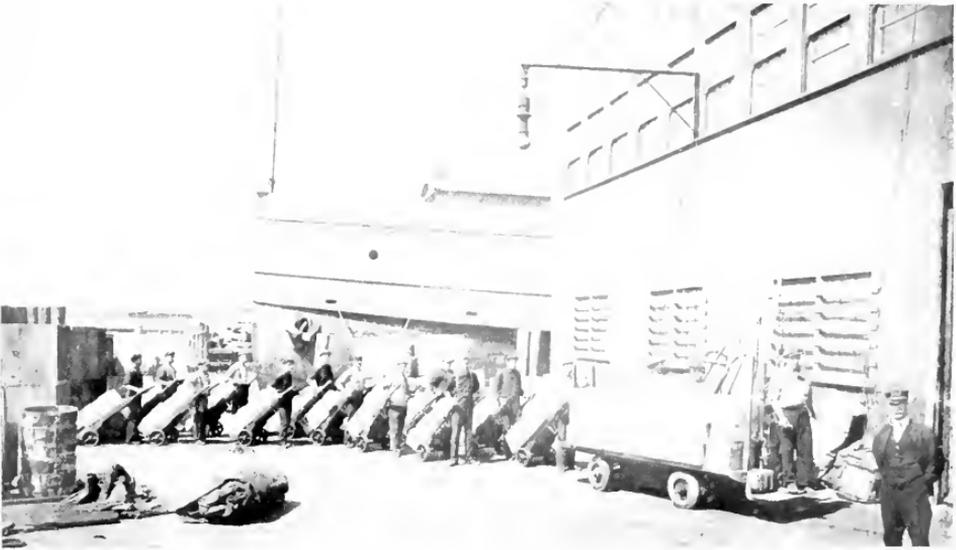
Sprague Electric Freight Truck Carrying 48 Cases of Canned Goods which as shown is Equivalent to 12 Hand Truck Loads
