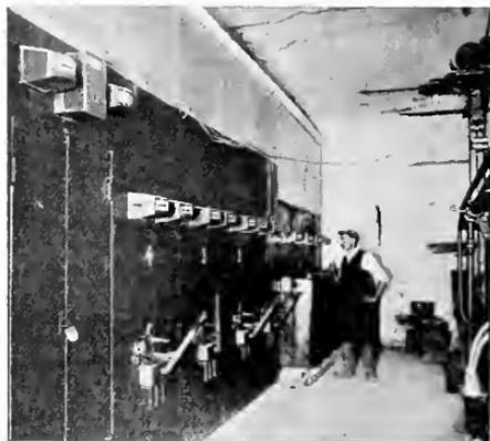
Fig. 3. Switchboard for Controlling the Operation of the Pumping Plant Illustrated in Fig. 1
