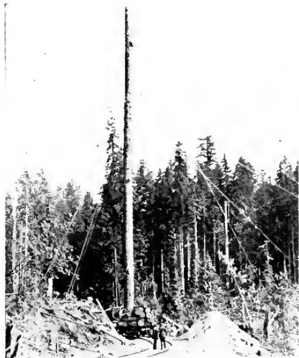
Fig. 34. Use of Tree Trunk for Handling the Yarder and Hoisting Cables for Hauling in Logs and Loading Them on Railroad Cars
