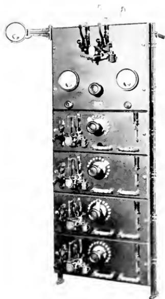
Fig. 3. Charging Panel Consisting of Generator Control Section and Four Charging Sections
