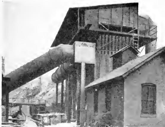
Fig. 5. Completed Installation, Showing Inlet Connections, Concrete Hoppers and Pipes
