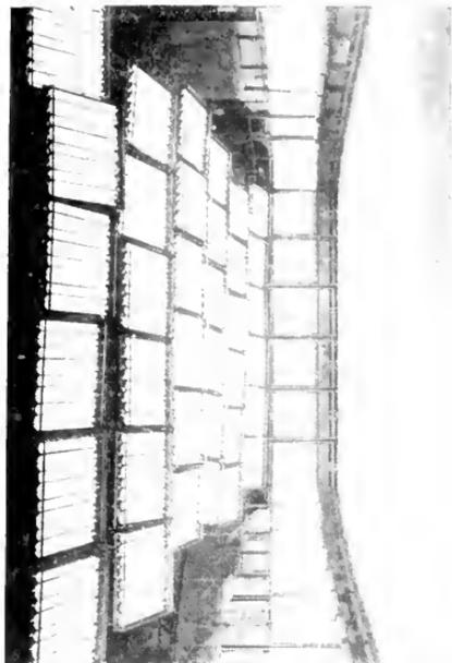
Fig. 2. Banks of Cooper Hewitt Lamps in a Studio. An example of "soft" lighting.
