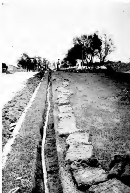
Fig. 8. Band Steel Armored Cable is generally recommended in places where no conduit exists as it can easily be laid in the ground without conduit as shown in this illustration
