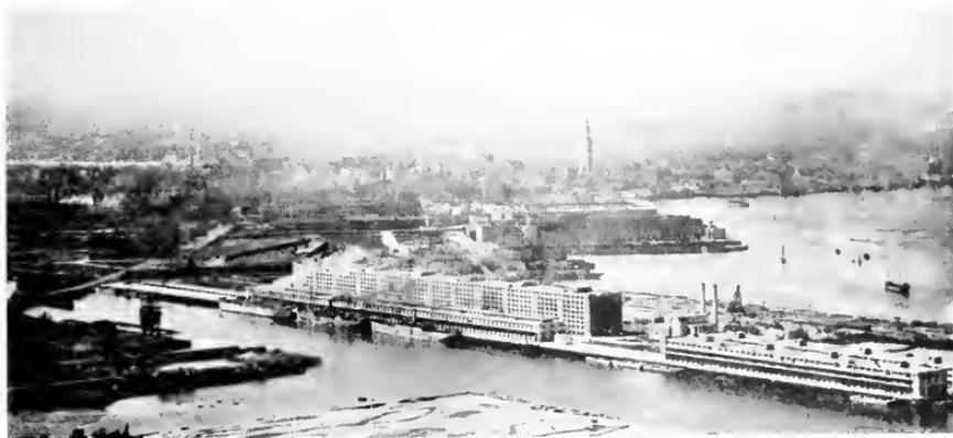
Fig. 1. Airplane View of a Modern Marine Terminal—The Boston Quartermasters' Terminal—showing the two-story pier sheds served by gantry cranes and the eight-story supporting warehouse in the rear. The powerhouse for the terminal is also shown. It provides for heating the buildings and also contains substation equipment for converting the power obtained from the Edison Electric Illuminating Company
