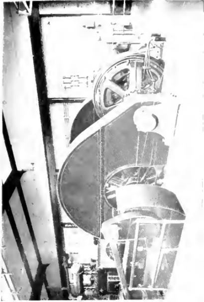
Fig. 2. 800-h.p., 360-r.p.m., 2000-volt Wound-rotor Induction Motor Geared to a Pump; Originally Driven by a Steam Engine.
