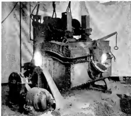
Fig. 6. Two-ton Three-phase Electric Arc Furnace Developed at the Schenectady Plant About 1908. At the time it was the largest capacity electric steel furnace in existence
