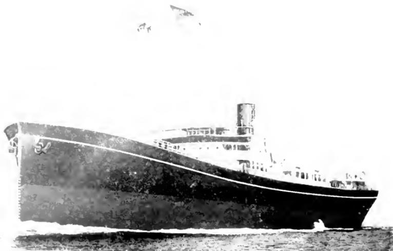
The *Robin Gray* is an Express Freighter Propelled by a 3000-h.p. Turbine Geared Unit of the Two-plane Double-reduction Type. The boat entered the service in the early part of 1920
