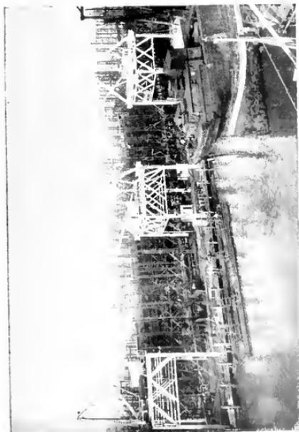
Fig. 3. Stationary Cranes of the Swing-boom or Derrick Type.
