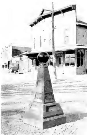
Fig. 9. Special Type of Post Used for "Silent Policeman" at Street Intersection
