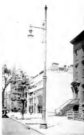
Fig. 10. Combination Ornamental Iron Pole Used for Trolley Span Wire and Street Lamp Suspension
