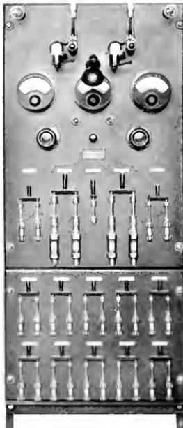
Fig. 3. Typical Auxiliary Distribution Switchboard for Small Capacity Circuits
