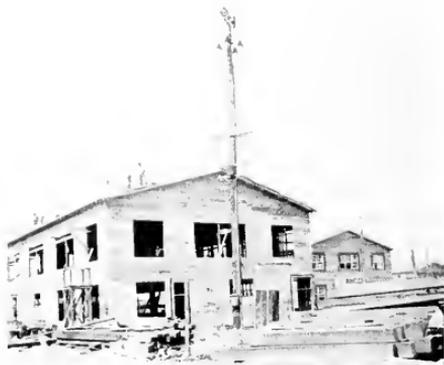
Fig. 10. Novalux Units and Floodlighting Projectors Mounted on 50-ft. Pole. Hog Island Shipyard, Philadelphia, Pa.
