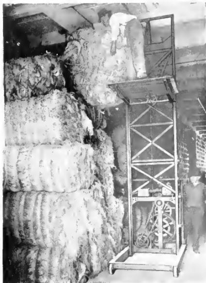
Fig. 5. A Portable Elevator, Electrically Driven, Piling Heavy and Unwieldy Bales of Sisal
