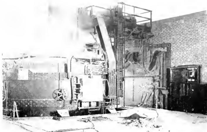
Fig. 3. Another View of 40-ton Furnace, Showing Control Panels on Right and Electrode Motors on Platform Above
