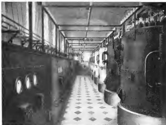
Fig. 3. A Battery of 2000-kw. Steam Boilers in Which the Water Itself Comprises the Heat Generating Resistance
