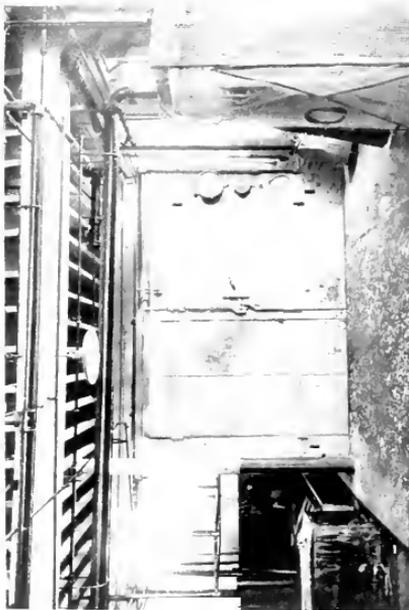
Fig. 3. Japan Baking Box Type Electrically Heated Oven, 8 Ft. High, 12 Ft. Wide, 18 Ft. Deep. 150 kw. connected, Chevrolet Motor Car Company, Tarrytown, N. Y.
