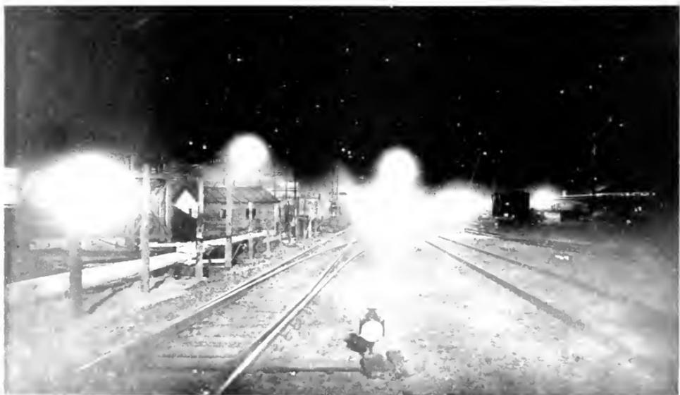
Fig. 12. Freight Yard Illuminated by Novalux Units. Hog Island Shipyard, Philadelphia, Pa.
