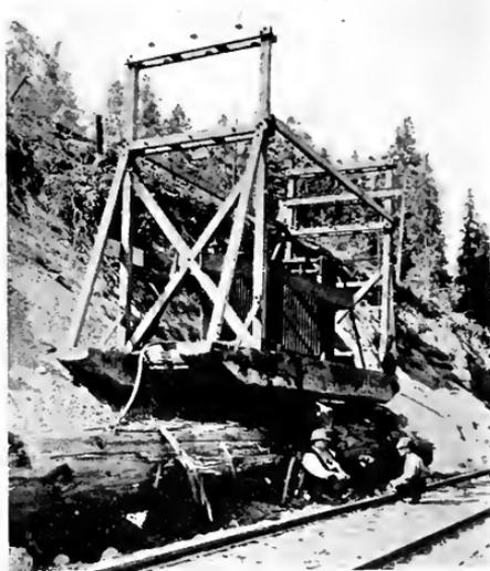
Fig. 35. Arrangement of Outdoor Transformer Equipment, Showing Method of Mounting on Sled and Location Near Railroad Track
