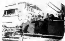
Electric Portable Conveyor speeds unloading with 100 ft. carry from slip to wharf shed.
