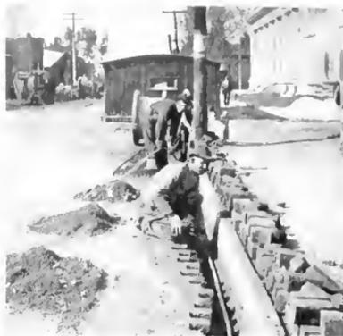
Fig. 3. Installation of Armored Cable in Brick Paved Street
