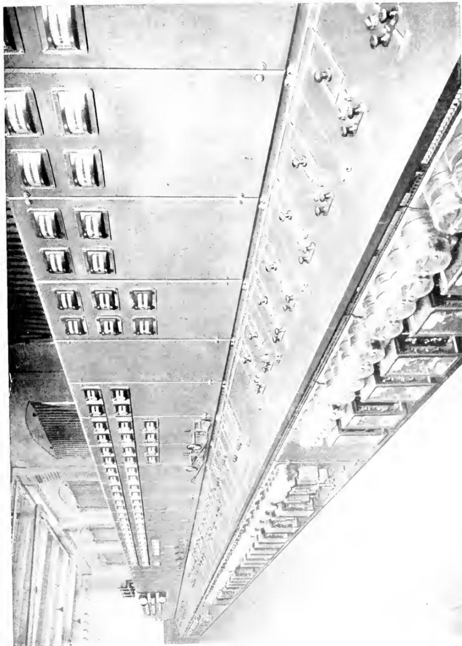
Fig. 2. Instrument and Control Board for Cape Town, Africa. This switchboard is more than 100 ft. long, and while it controls at present only 20,000 k.w., provision is made to handle several times this capacity.
