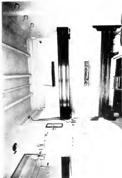
Fig. 5. A Typical Stateroom Lighting Installation. One central ceiling fixture employing a round bulb all-frosted, 34 inch B lamp and an adjustable lamp by the side of the berth. Enclosing glassware or fabric shades would have remarkably improved the installation.
