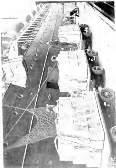
Fig. 3. Industrial Trucks Handling Miscellaneous Freight at Steamship Pier. Each truck contains ten to twelve hand truck loads and no time is lost at the ship's side making up the slings.
