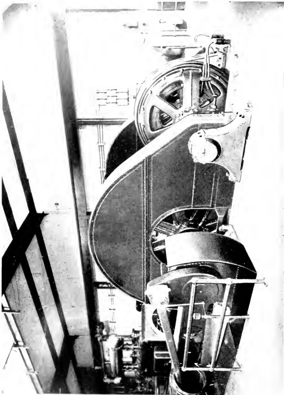
800-h.p. Induction Motor Geared to a Pump Originally Operated by Steam Power. Fig. Hole Pumping Station of the Butte Water Company, Devide, Montana. This installation is a striking example of the preference that is everywhere being shown for electric drive. Aside from the simplicity, cleanliness, convenience, and freedom from trouble of the electric motor, the matter of economy is largely responsible for its popularity.
