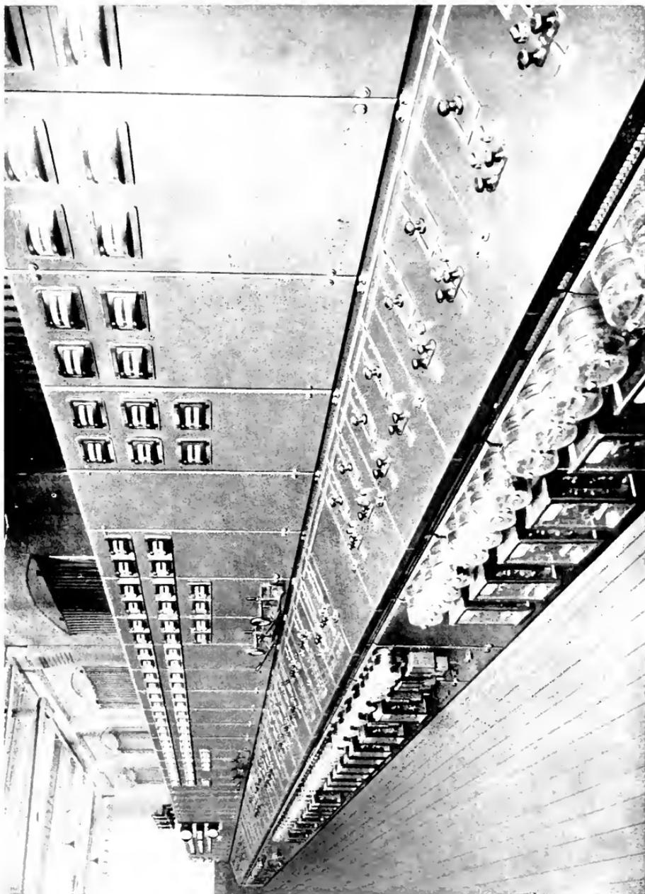
An Elaborate Instrument and Control Board for Cape Town, Africa. This switchboard is more than 100 ft. long, and while its controls at present only 20,000 kw. provision is made to handle several times this capacity. It was completed late in 1920, and will be described in an early issue of the *General Electric Review*.
