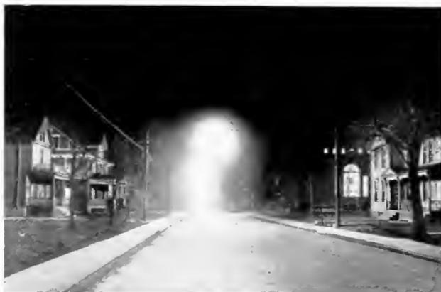
Fig. 8. A Street Intermediate Between a Business District and Highway Lighted by Novalux Mazda Lamp Units Equipped with Reflectors
