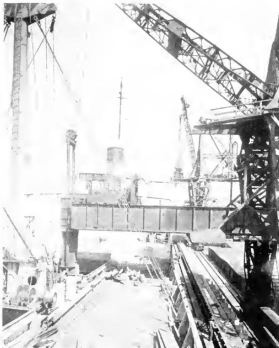
Fig. 1. Conveyor Tower and Ram with Coal Trimmer in Position to Operate
