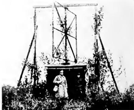
Fig. 4. Direction Finding Radio Station with Camouflage Protection as Employed for Military Purposes in France
