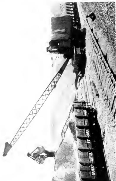
Fig. 4. View of Electrified Steam Locomotive Crane Unloading Cars to Storage Piles
