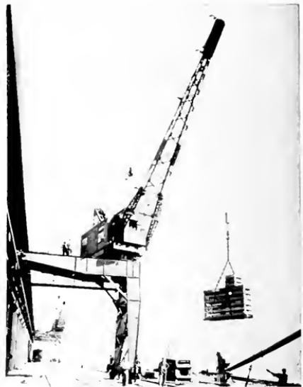
Fig. 2 Half Arch Gantry Revolving Jib Crane on a Quay for Loading and Unloading Ocean Going Ships
