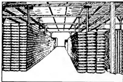
Fig. 3. Shells as Piled at the Closing of the War, Showing Decreased Floor Space Required Due to an Extensive Use of Dunnage
