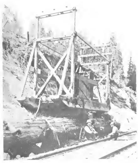
Arrangement of Outdoor Transformer Equipment Showing Method of Mounting on Sled and Location Near Railroad Tracks
