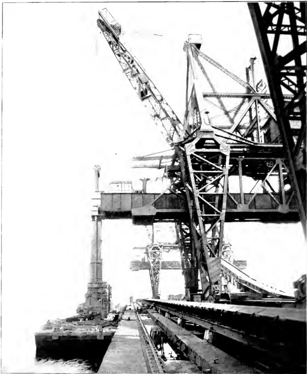
TRIMMING MACHINE LOCATED ON END OF COAL DELIVERING RAM OF
