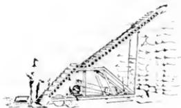
Fig. 7. Portable Conveyor or Motor-driven Tying Machine. The height of the boom is adjustable. Capacity one ton per minute. This device is useful for high piling of bags, bales, boxes, and rolls in a warehouse.
