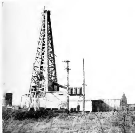
Fig. 4. This Well is being drilled by the Roxana Petroleum Co. with motor-operated cable tools, power being received from Guthrie, Okla., over a 6½-mile, 6600-volt transmission line which the Company built and operates to save the expense of hauling fuel for steam drilling
