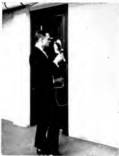
Fig. 20. Measuring Vertical Illumination of Wall Brightness with the Macbeth Photometer
