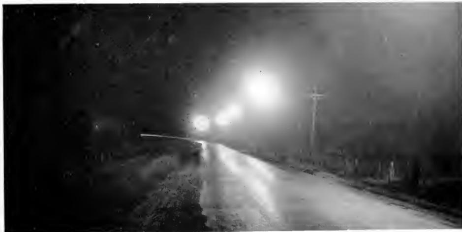
Fig. 3. Paradise Road, Swampscott, Illuminated by Highway Lighting Units Containing 250-c.p., 4-amp. Mazda Lamps
