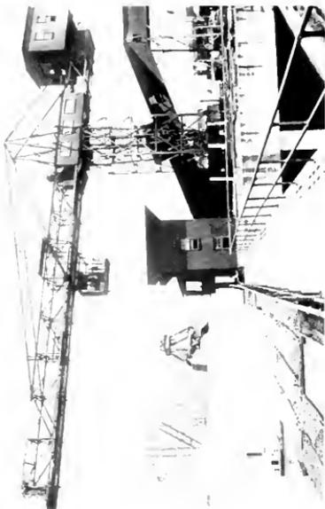
Fig. 6. Hammerhead Tower for Unloading Coal, La Belle Iron Works, Follinsbee, W. Va.
