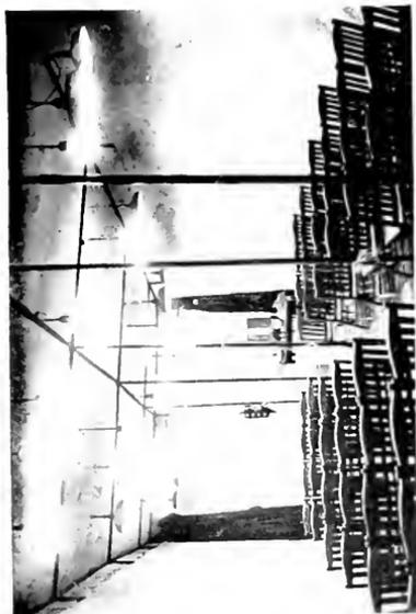
Fig. 87. Portable "Better Industrial Lighting." Demonstration. A canvass covering is supported on a knock-down pipe framework. Black curtains are used to change the character of wall finish. The lighting units are suspended from the framework and controlled from a switchboard at the front of the room. The demonstration apparatus will be noted on the lecturer's table.
