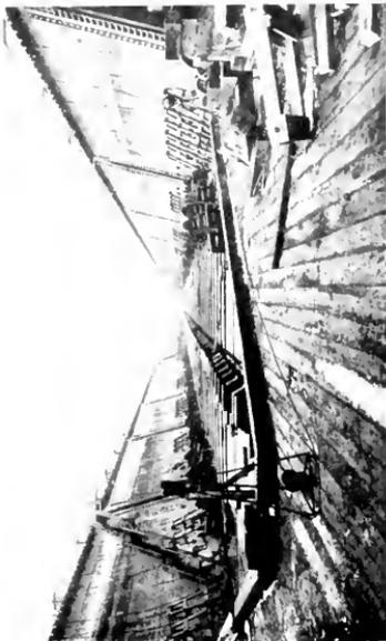
Fig. 2. All Six Sections of the 30,000-ton Floating Dry Dock of the Morse Dry Dock and Repair Company Ready to Submerge and Rise Again Holding the Ships Seen in the Distance
