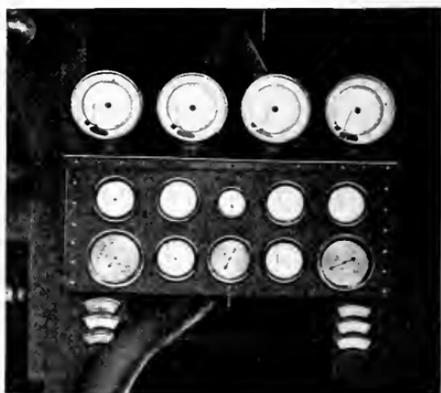
Fig. 3. General Electric Steam Flow Meters Installed in a Large Central Station
