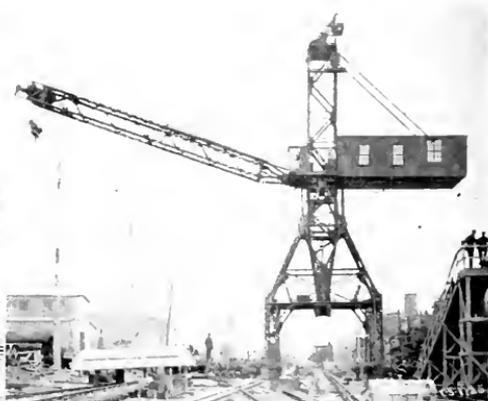
Fig. 2. Revolving Jib Traveling Pillar Crane. Merchant Shipbuilding Corp., Bristol, Pa.
