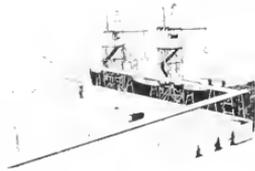
Fig. 42. Coal Tower Hoists unloading coal or bulk material from boats into cableroad which stores it in stock pile. Capacity over 600 tons per hour.
