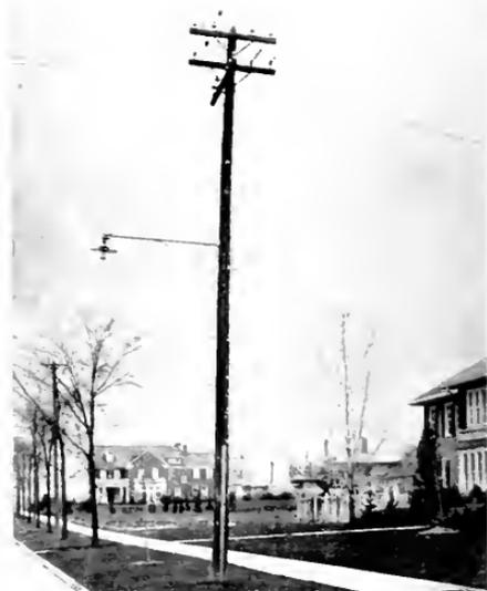
Fig. 1. Aerial Line Construction Showing Series Lamp Bracket Suspension
