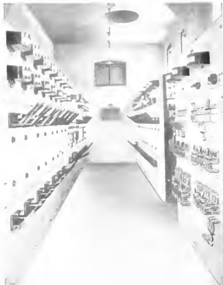
Fig. 3. Panels for Controlling 46 Motors in an Electrified Terminal Elevator
