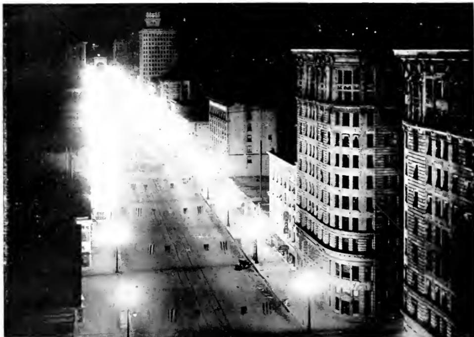
Fig. 7. Main Street, Salt Lake City, Utah, Lighted by Ornamental Luminous Arc Lamps
