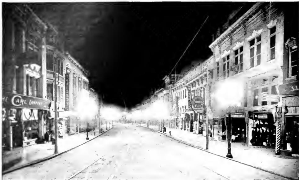
FIG. 3. State Street, Schenectady, N. Y., Illuminated by Ornamental Luminous Arc Lamps
