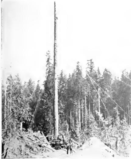
Use of Tree Trunk for Handling the Yarder and Hoisting Cables for Hauling in Logs and Loading Them on Railroad Cars
