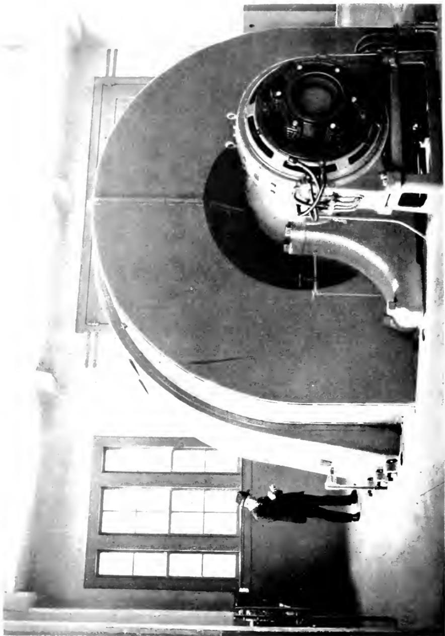
30,000 kv. a., 6000 volt, 3 phase, 50 cycle Synchronous Condenser Located in the Eagle Rock Substation of the Southern California Edison Company. Two articles relative to the future operation of the transmission lines of this company at 220,000 volts appear on pages 197 and 199 of this issue.
