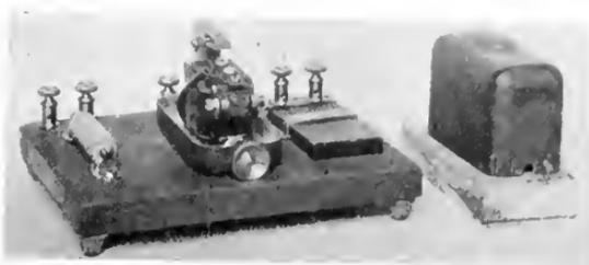
Fig. 4. Stabilizer for the Coolidge Tube - Experimental Model
