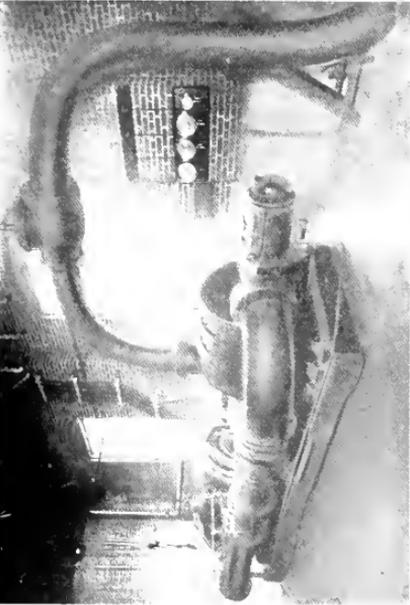
Fig. 1. 1300-h.p., 1200-r.p.m., 2200-volt Wound rotor Induction Motor Direct Connected to Double-suction Impeller Pump of 6,000,000 Gal. Capacity per 24 Hr. Against a Head of 875 Ft.
