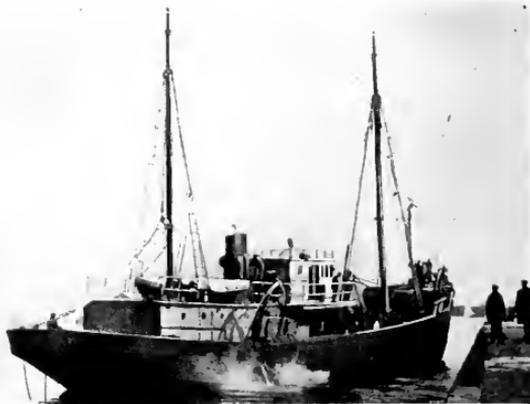
Fig. 8. The Mariner, the First Electrically Propelled Trawler
