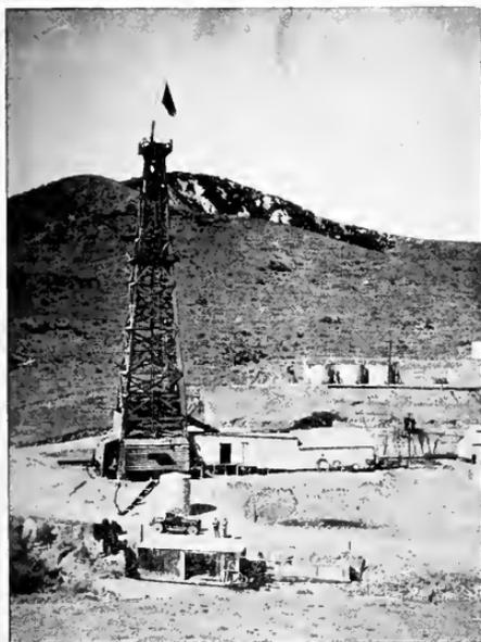
Fig. 28. The "Anita A" Well of the Shell Company of California Drilled by Standard 75-h.p. Oil Well Drilling Motor Equipment
