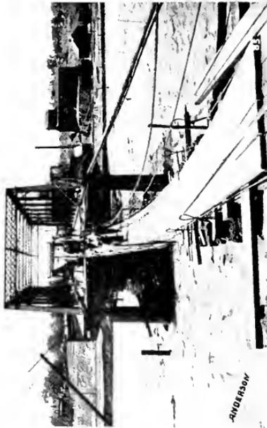
Fig. 1. Fourth Street Bridge for Street Cars and Wagons. Only bridge left out of six. Foot bridge shown made from street car rails and ties
