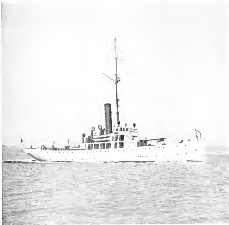
U. S. S. TAMPA, FIRST ELECTRICALLY PROPELLED COAST GUARD CUTTER
