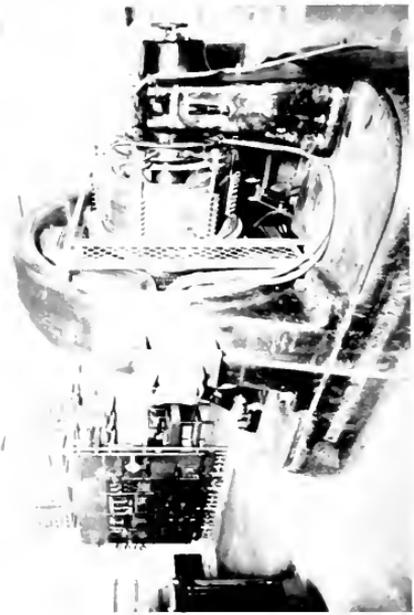
Fig. 10 Interior of the Kenosha Automatic Substation, Showing Control Board and Load-limiting Resistors
