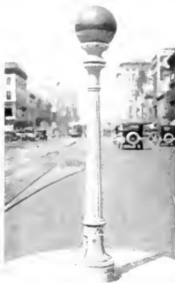
Fig. 8. Traffic Post Installation on Safety Island in Busy Section of City Street
