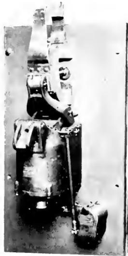
Fig. 78. Self-setting, Under-voltage Device for Solenoid-operated Air Circuit Breakers
