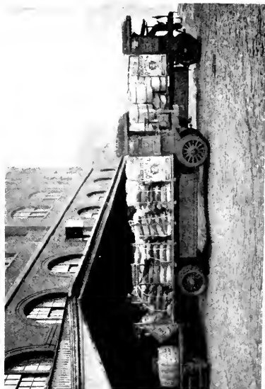
Fig. 4. Five-ton Electric Trucks in Heavy Hauling Service. (Commercial Truck Company)
