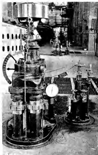
Fig. 8. A Hold-off Sign, Chain, and Lock which prevent the operation of either the governor or the hand controls. The turbine gates are half-way open to prevent the formation of an accumulation of headgate leakage that might move the rotating element
