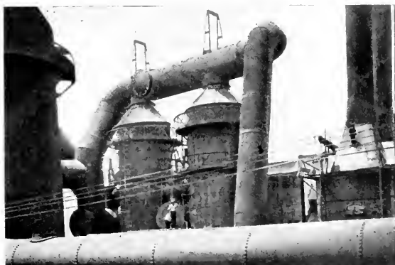
Fig. 7. Two Precipitator Units Handling Blast Furnace Gases
