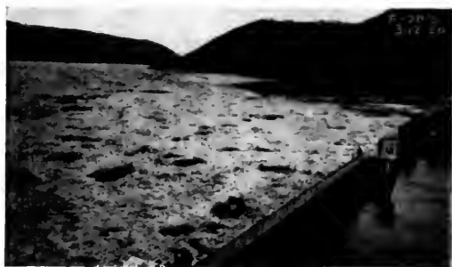
Fig. 4 Cake Ice Does Not Ordinarily Affect Hydro Plant Operation. This illustration shows how an arched wall prevents the ice from getting into the forebay.
