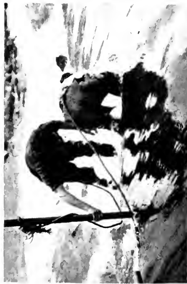
FIG. 3. When men must get out on the crest of a dam, handlines about the waist are necessary.
