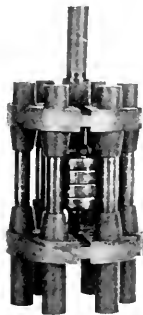
Fig. 35. 110-kv-a., 200-ampere Ratio Adjuster
