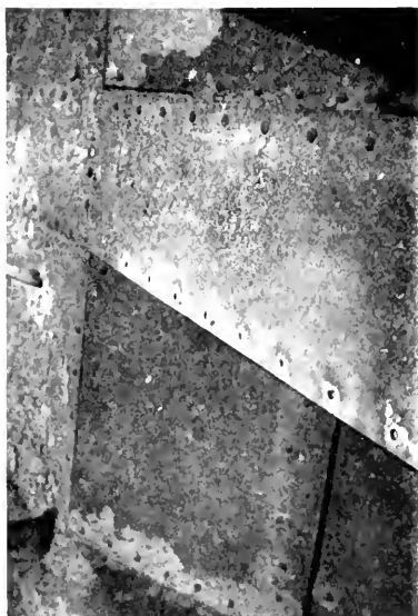
Fig. 3. Sample of Floor Work. These eight rivets were burned at the rate of 400 per hour
