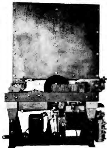
Fig. 11. Locomotive High Speed Circuit Breaker
