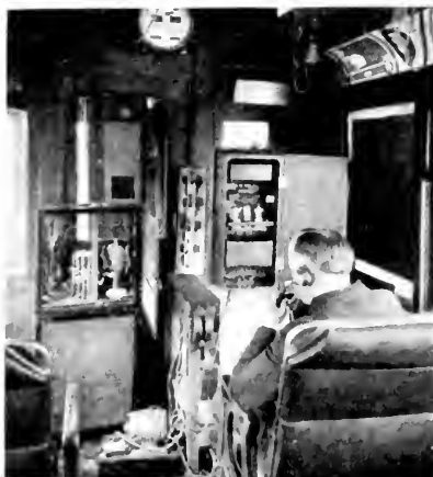
Fig. 39. Operation of Carrier Current Communication on Test Car
