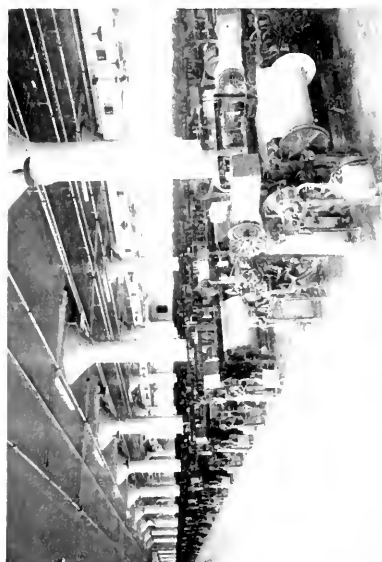
Fig. 2. 1728 Draper Looms Individually Driven by 1\frac{1}{2} -h.p. Loom Motors
