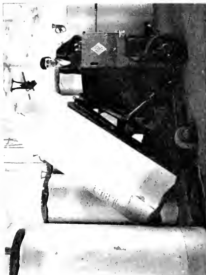
Fig. 2. Special Electric Tiering Truck for Handling Large and Heavy Annealing Pots
