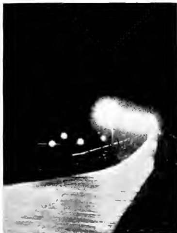
Fig. 6. A Section of the Albany-Schenectady Highway Lighted by Novalux Highway Lighting Units Equipped With 2500-Lumen (250-c.p.) 6.6-amp. Mazda C Series Lamps
