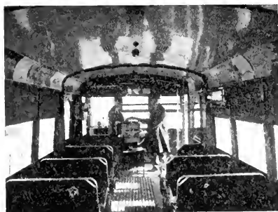
Fig. 7. Interior of Lexington Car, Showing Fare Register Mounted under Table on which Change is Handled
