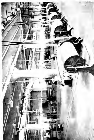
Fig. 7. Ten 56-in. Beacon Frames Group Driven by 30-h.p. Motor
