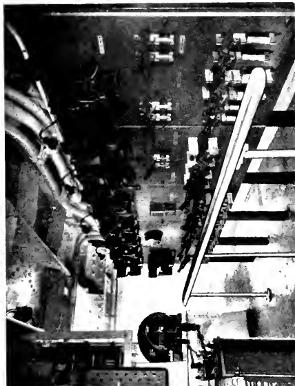
Fig. 5. Pump Control Room Showing Auxiliary Distribution and Control Board for Cargo Oil Pumps. Pump motor controllers, resistance grids, and ventilating motor at the left
