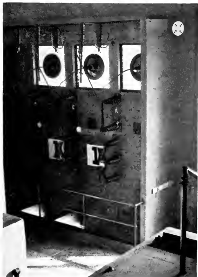
Fig. 3. Sleet Prevention Facilities at Receiving Station. The upper disconnectors serve to short circuit the transmission line when heating current is to be circulated. The disc in the upper right-hand corner carries eight 8-volt lamps in parallel connected to a series transformer in the short circuiting connections and indicates when the heating current is on.
