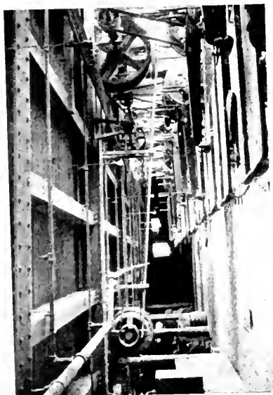
Fig. 3 50-h.p. Induction Motor Driving 31 Staking or Softening Machines
