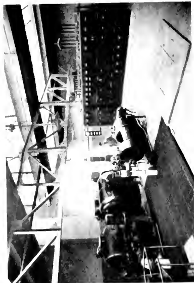
Fig. 4. One 750-kw., 3600 r.p.m., 480-volt Curtis Condensing Steam Turbine Arranged for Automatic Steam Extraction, and one 100-kw., 3600-r.p.m., 480-volt Curtis Steam Turbine at the Plant of John R. Evans Co. (An additional 750-kw. unit will soon be installed.)
