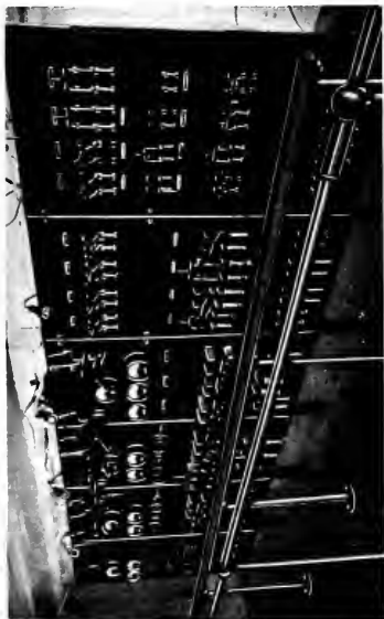
Fig. 2. Main Switchboard for the Control of the Auxiliary Generators and the Distribution of Power
