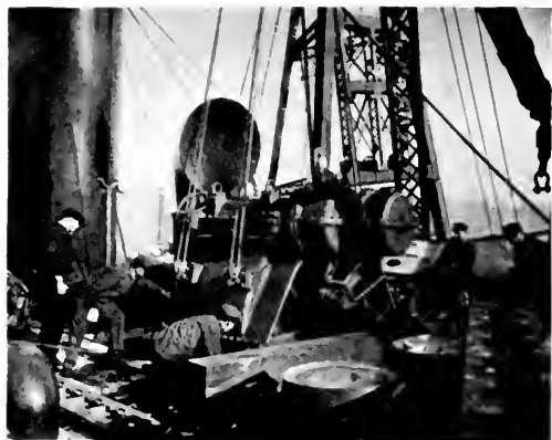
Fig. 9 Replacing a Set of One-plane Reduction Gears by the Two-plane Type in the Record Time of Ten Days
