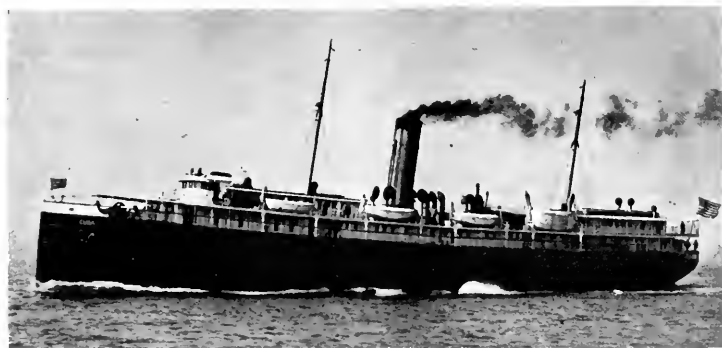
Fig. 1. S. S. Cuba, the First Electrically Driven Passenger and Express Freight Steamer
