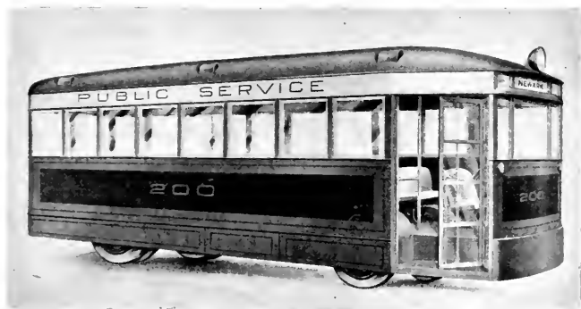
Fig. 2. Twenty-five Passenger Electric Bus (Electrocar Corporation)
