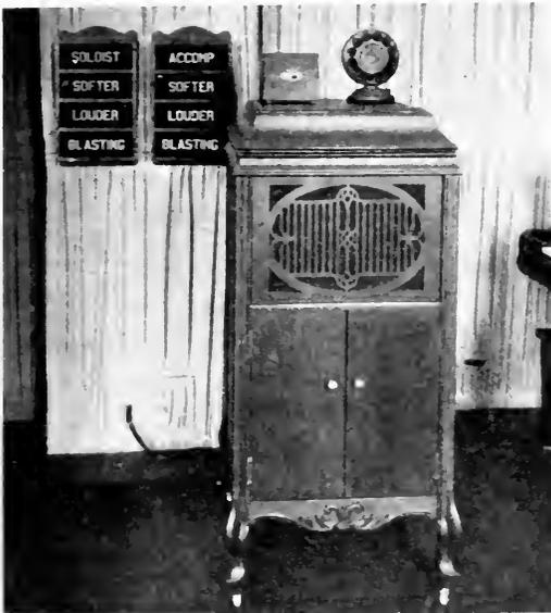
Fig. 14. Announcer's Microphone and Control Box on the Phonograph and the Studio Manager's Indicator on the Wall
