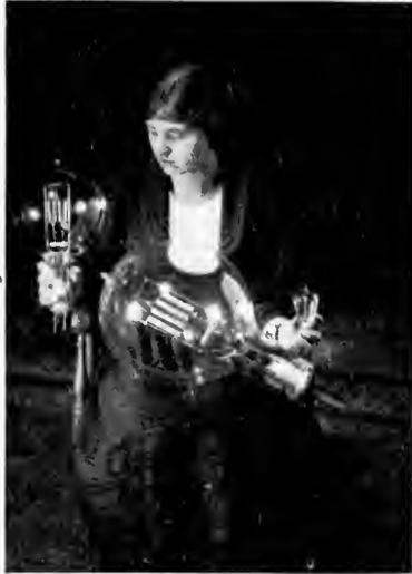
Fig. 74. 10-kw., 30-kw. and 25-watt Incandescent Lamps
