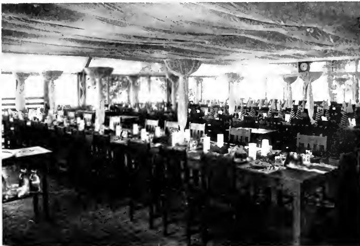
Fig. 80. Lighting pedestals which project slowly moving bands of blended color on the ceiling by means of a motor rheostat device
