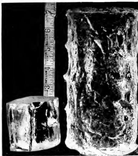
Fig. 5. Two Clear Fused Quartz Slugs made in the Thomson Research Laboratory, General Electric Company, Lynn, Mass., April 27, 1922
