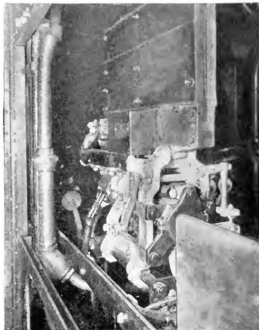
Fig. 13. Apparatus Compartment Showing Location of High-speed Circuit Breaker
