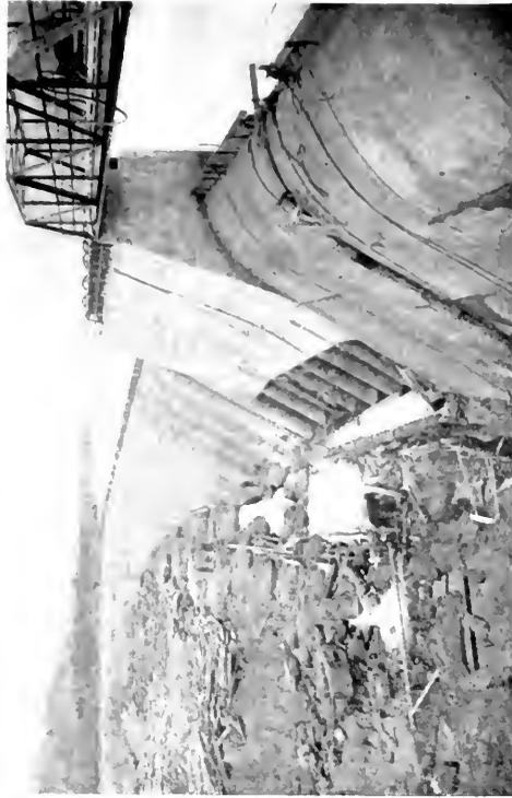
Fig. 3. Spillway from South End of Main Dam. Its great length 864 ft prevents floodwater overtopping the dam
