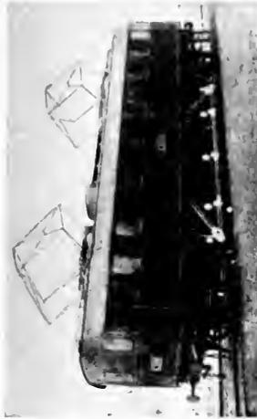
Fig. 9. Midi Railway, France. Direct-connected side-rod drive with two motors, C.F.T.H., Paris, and Swiss Locomotive & Machine Works, Winterthur
