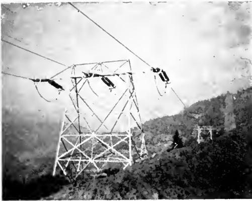
Fig. 9. Anchor Tower on 220,000-volt Big Creek Line of the Southern California Edison Company
