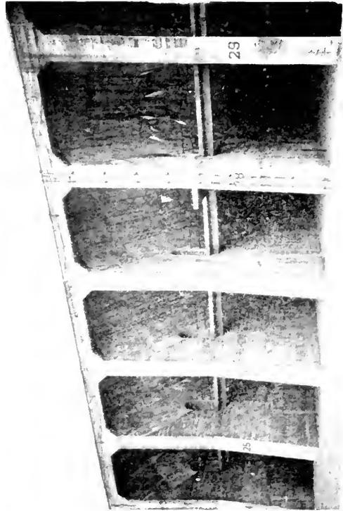
Fig. 4. A Detail of the Main Dam. A depth of 20 ft. of sand on the slab reduces the apparent height very materially
