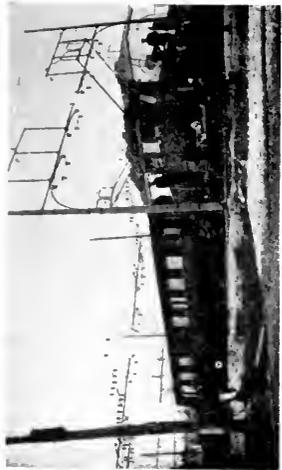
Fig. 7. Italian State Railways. Direct-connected side-rod drive with Scotch yoke. Type originally built by the Italian Westinghouse Vado Ligure Works and later by other Italian manufacturers
