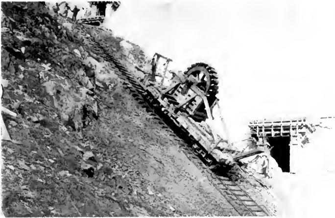
Fig. 3. Lowering 28-ton Generator Rotor to Power House, Jan. 8, 1923
