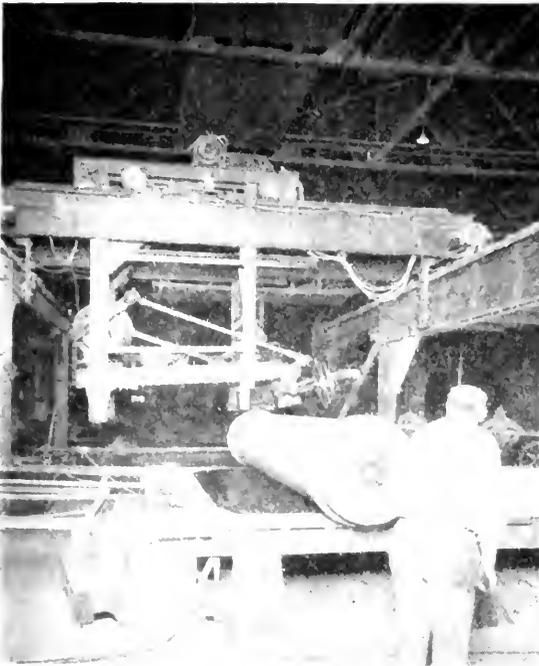
Fig. 4. Teeming Crane, Casting Table and Roller
