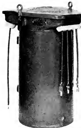
Fig. 41. Plain Welded Steel Tank for Distribution Transformers
