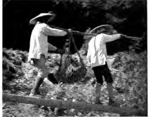
Fig. 5. Method of Excavating by Means of Rope Baskets
