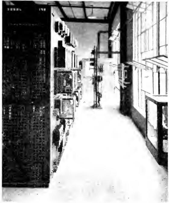
Fig. 12. Back View of Main Control Switchboard
