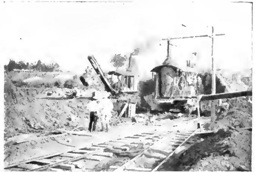
Fig. 6. Modern Method of Excavating by Means of Steam Shovels; Shinetsu Electric Power Company
