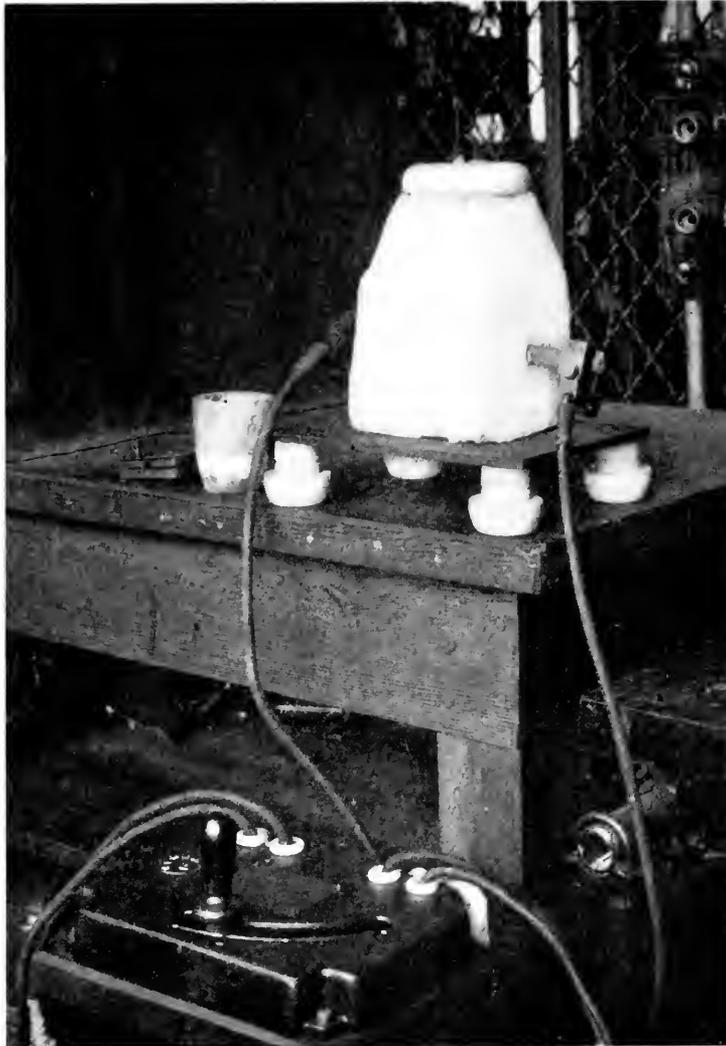
Fig. 1. Electric Arc Furnace Supplied with Energy from the Standard Compensarc in the Foreground. The combination is here employed for melting the alloys in which abrasive diamonds are mounted
