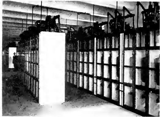
Fig. 7. Switch Gallery of the White Bay Power House. Cell doors are of wood and glass
