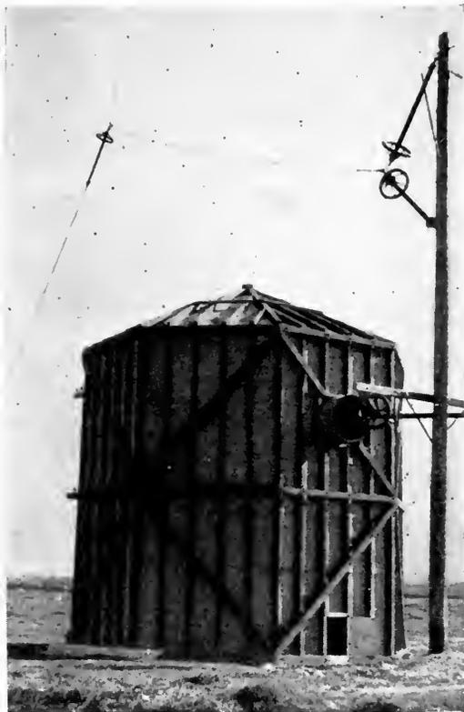
Fig. 4. Coil Similar to That of Fig. 3, but Housed in a Frame Structure Lined with Copper
