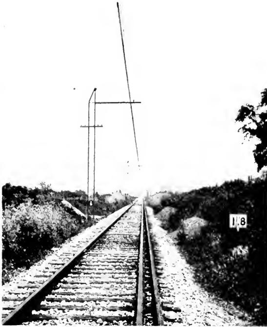
Fig. 4. The Overhead Trolley Suspended from Latticed Side Bracket Poles
