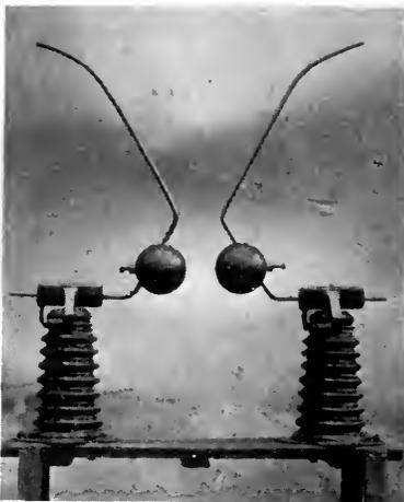
Fig. 4. Original Sphere Horn Arrester Gap
