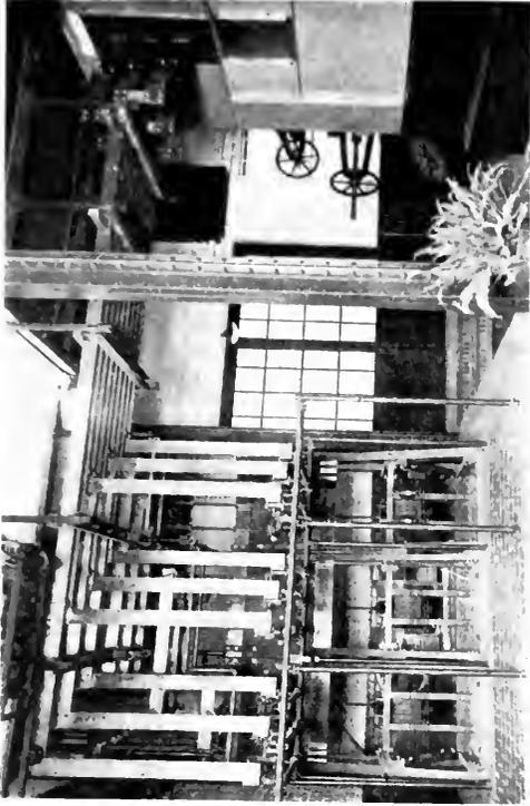
Fig. 3. Arrangement of Main Busbars between Generator and Switchboard
