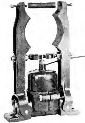
Fig. 44. Magnetic Brake for Induction Regulator
