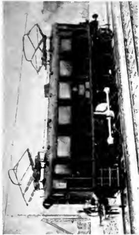
Fig. 8. Prussian State Railways. Direct-connected side-rod drive with one motor through a vertical rod, A.E.G., Berlin
