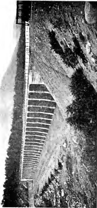
Fig. 2. Main Dam from Bank of Power Canal. The dam is 551 ft. long and 170 ft. high, and is built on gravel and boulders
