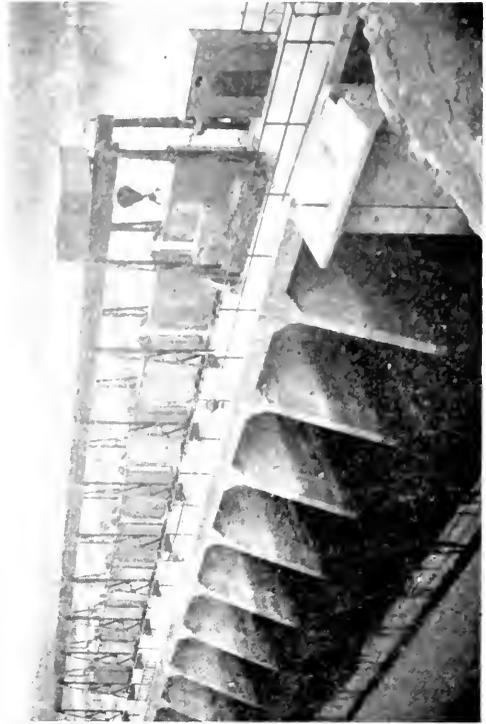
Fig. 5. Headgates and Gate Hoist Overlooking the Pond. A portion of the dam and spillway may be seen through the hoist runway
