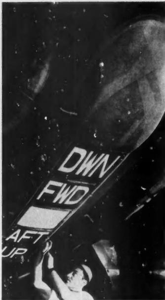
**TRAFFIC LIGHTS** on tanker directs receiver pilots during in-flight refueling
