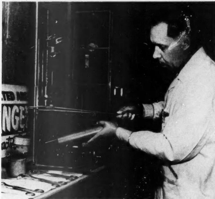
RADIOACTIVE sources are readily checked with this portable radiation probe
