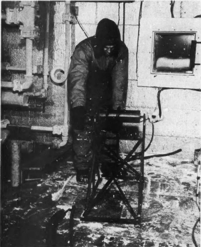
**RADAR CABLE** for outdoor portable equipment is tested in special rooms at  $-65$  F. At the other extreme, this same cable is able to withstand temperatures of  $+135$  F
