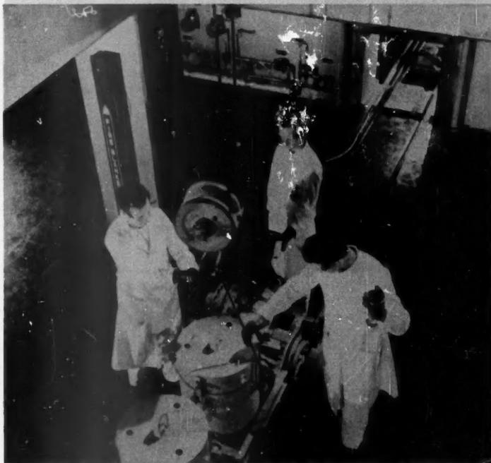
FISSION PRODUCTS after separation from unburned fuel are contained in shielded casks rolled out through the rear wall in an early step in disposal
