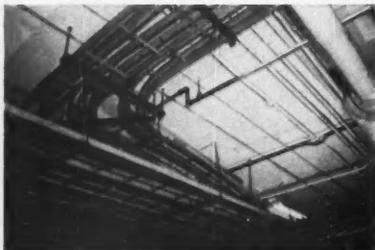
**MAIN FEEDERS** and all other distribution were handled exclusively by G-E interlocked armor cable. This cable, pre-installed in its own raceway, offered many installation advantages not possible with other cable systems.
