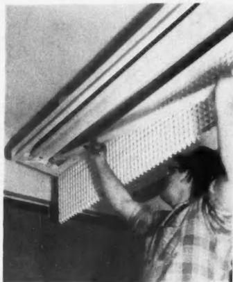
Fig. 7. RELAMPING is easy with the slimline base and socket combination
