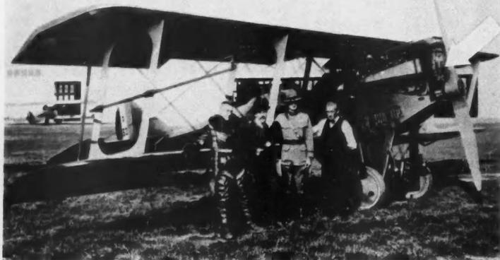
**1** Turbosuperchargers aided development of the jet engine by giving engineers background on the behavior of metals at high temperatures. G-E unit (arrow) helped get this biplane to 40,800 feet in 1921. During World War II . . .
