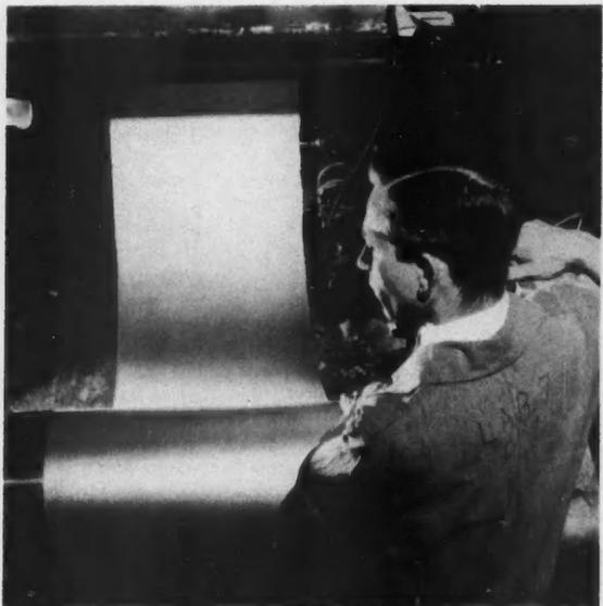
**1** Making mica mat is somewhat similar to making paper. The continuous rolls that come off the machine can be made into ...
