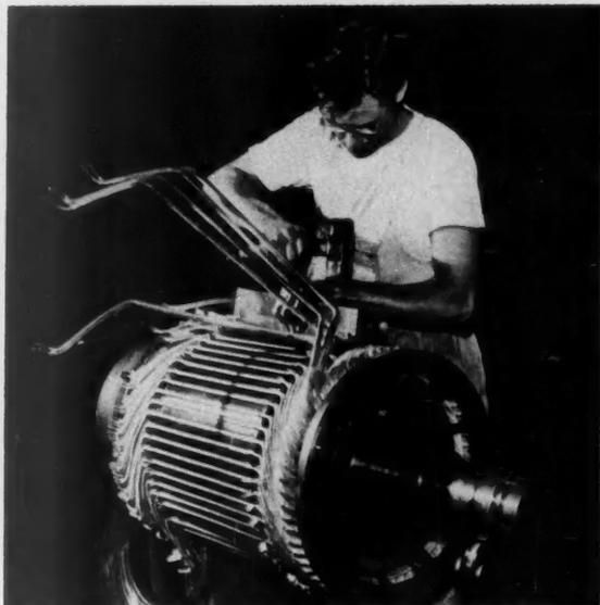
**4** Armature coils wound with mica mat tape in a transportation-type motor for withstanding high operating temperatures
