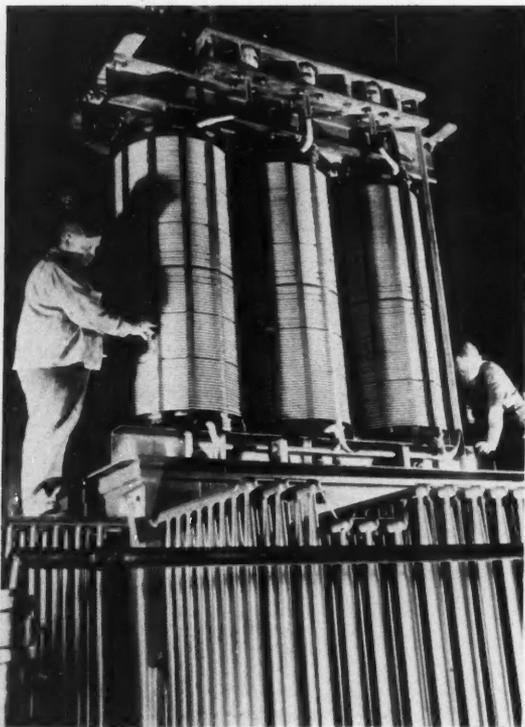
POWER TRANSFORMERS, such as this unit on the assembly floor, have joints sealed by nitrile gaskets for greater reliability
