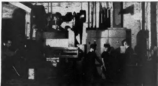
"We get power where it's needed, when it's needed, at presses and machine tools located at many different points," explains Schaefer, "by this method: LVD (Low Voltage Drop) FLEX-A-POWER feeds this packaged Trumbull Centr-A-Power switch-board from an outside transformer, then a network of FVK FLEX-A-POWER, the secondary or plug-in distribution system, takes off from there and criss-crosses the whole plant. There's an FVK outlet every foot of the way.
