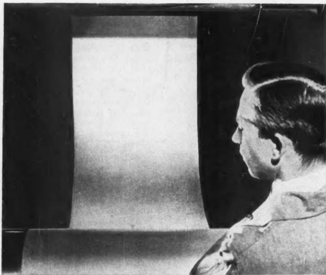
Continuous G-E mica mat sheet emerges from machine which forms minute mica flakes into flexible rolls of highly uniform mica insulation.
