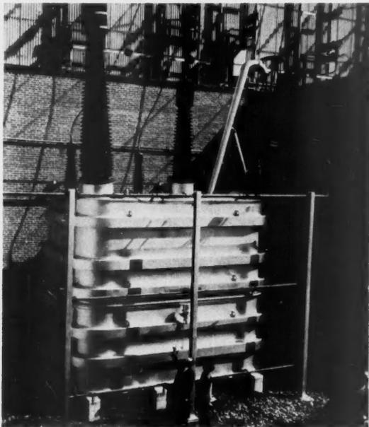
**11** Two 100,000-kva single-phase power transformers supply test power up to 440-kv single phase, 220-kv three phase. They have low reactance to give maximum short-circuit kva
