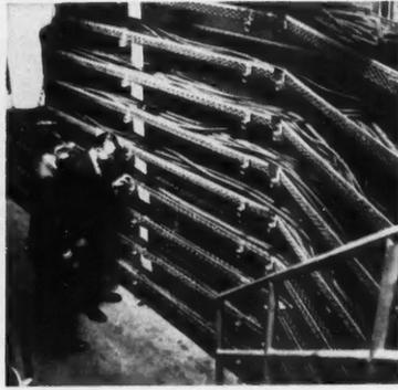
**7** Tunnel connects control and test buildings. Trays on either side carry all control cables
