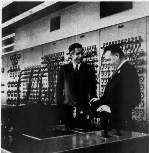
**20** Back in the control building, Gaty and Cox examine one of the six magnetic oscillographs used for recording test results. Test connections are made on the plug board
