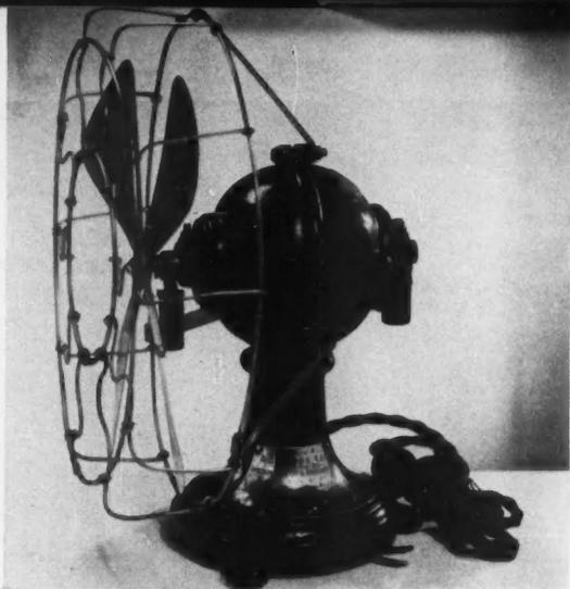
**2** Fans celebrated major events. One occasion commemorated generation of power at Niagara Falls in June, 1896, when this fan was operated for the first time by current transmitted to New York City. To permit either d-c or a-c operation at frequencies from 20 to 133 cycles . . .
