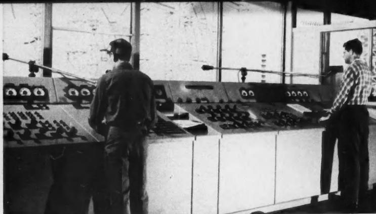
**2** Master control benchboard in the control building. All testing operations are controlled from this point. Microphones tie operators into a two-way public-address system that covers outdoor and indoor areas
