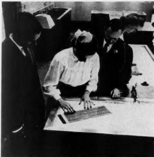
**21** Two minutes after a test, the still-wet oscillograph films are checked on a "wet" reading table. Essential calculations are made to guide in setting up the next test
