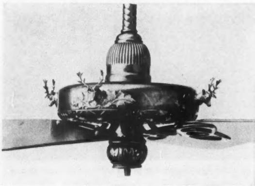
**5** Fans were suspended from the ceiling. They had blade diameters of 52 to 56 inches, operated at 250 rpm, and moved large volumes of air at low velocity. This one was standard equipment for the 1912 trophy room. And . . .
