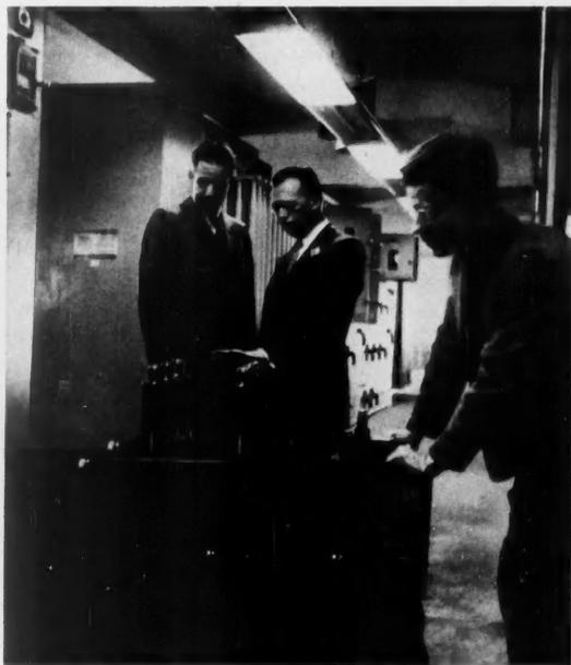
**14** Power for driving motors of the testing generators goes through this 4.16-kv metal-clad switchgear in test building. Substation in background is for auxiliary services
