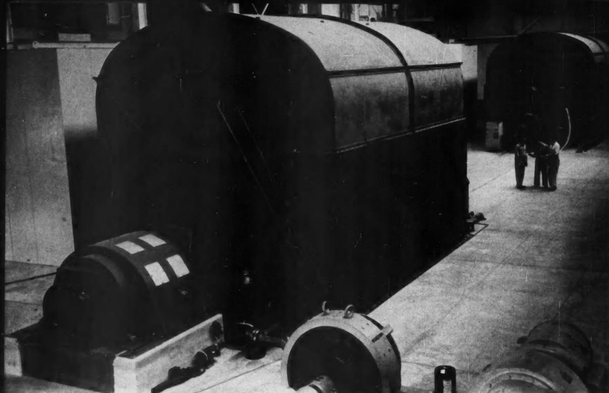
**15** These generators supply the highest short-circuit current available in any laboratory. Together they can deliver at the test bus an asymmetrical three-phase short circuit of 5,250,000-kva (3,200,000-kva symmetrical) at 15.5-kv
