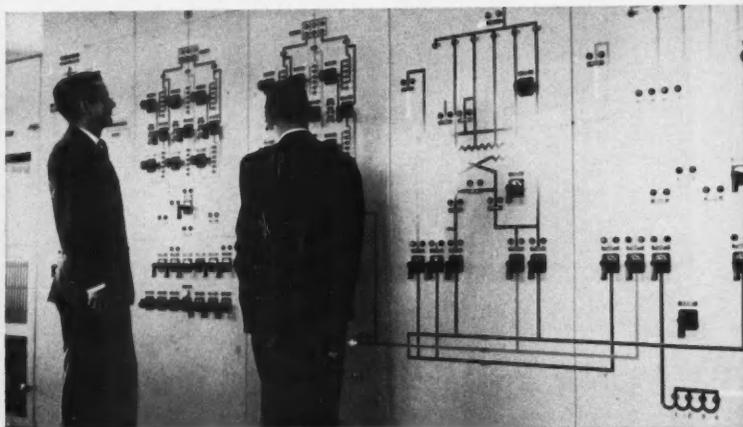
**4** Switchboard where power circuits for tests are set up. Mimic bus diagram and lights help engineer visualize circuit as he sets it up by operating the control switches on the board. One-line diagram is in color on face of switchboard
