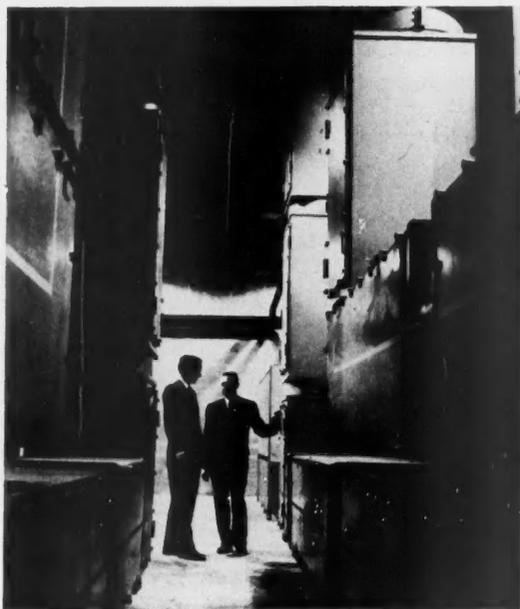
**13** Connections from generator to test cells and power transformers are made with isolated-phase bus runs of conventional design but braced for high momentary current
