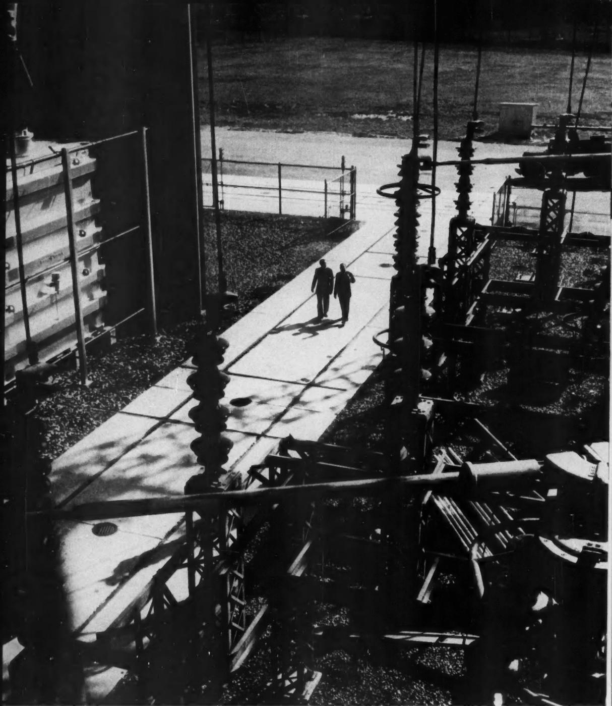
**10** Stretching across the foreground is the blade arm of one of the two five-position transformer tap selector switches. Motor-driven, they are operated from the control building to select the desired transformer tap
