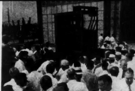
**AFTER DEMONSTRATION**, visitors get a close-up view of damage done in test they have just observed. This 15-kv oil circuit breaker was tested at far above its 90,000-kva interrupting rating.
