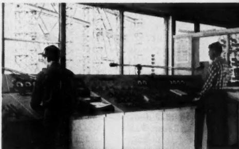
**NERVE CENTER** of new lab is this benchboard in the control building. Here, operators set generator output, then start automatic sequence sending up to 5,250,000 kva through equipment under test.
