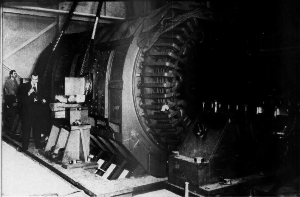
REINFORCED END WINDINGS AND UNIQUE SUPPORTING STRUCTURE CHARACTERIZE THE WORLD'S LARGEST SHORT-CIRCUIT GENERATORS
