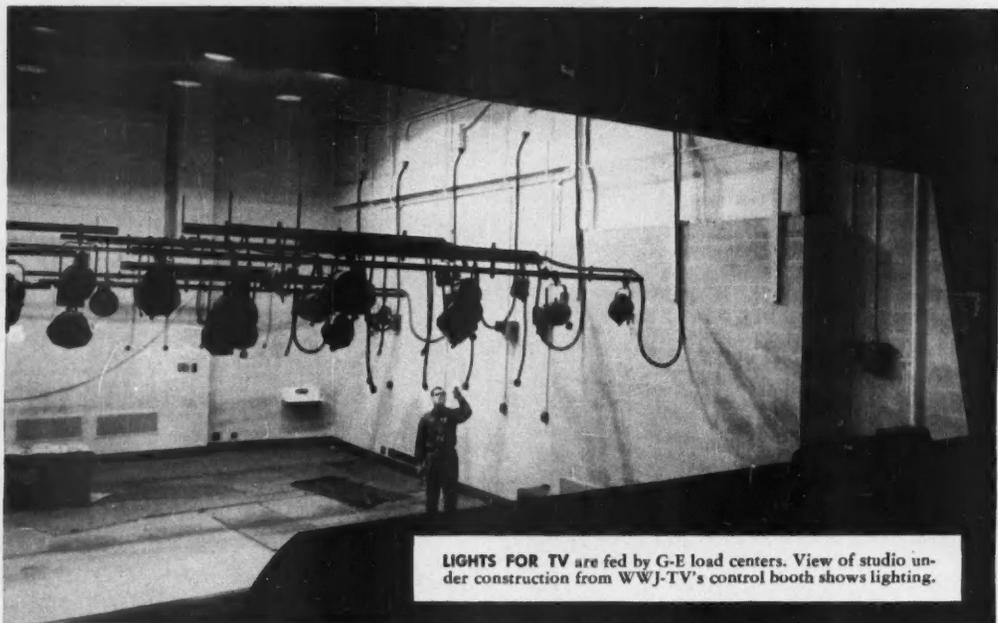
**LIGHTS FOR TV** are fed by G-E load centers. View of studio under construction from WWJ-TV's control booth shows lighting.
