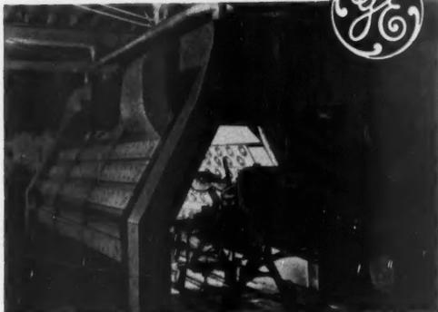
G-E 97.5 kw. infra-red oven drying finish coat on complete tractor assemblies. C.G.E. manufactures a complete line of industrial heating equipment.
