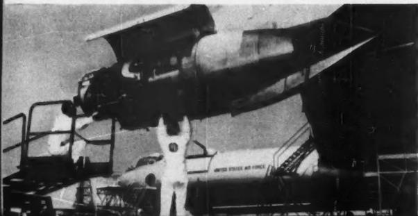
**AIRCRAFT MODIFICATION** for defense uses four G-E service centers, which work on aircraft gas turbines, turbosuperchargers and fire control. Here G-E technicians check a J47 jet engine.
