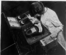
Hand-operated, G-E Inductrol being used in the calibration of a-c voltmeters against standard instrument. Just one of the many ways it helps increase efficiency and speed production.
