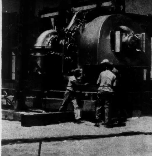
**SUPERVISION OF INSTALLATION** by G-E service engineers assures proper start-up of this gas turbine—one of 28 units for gas-pipeline pumping in the Southwest.
