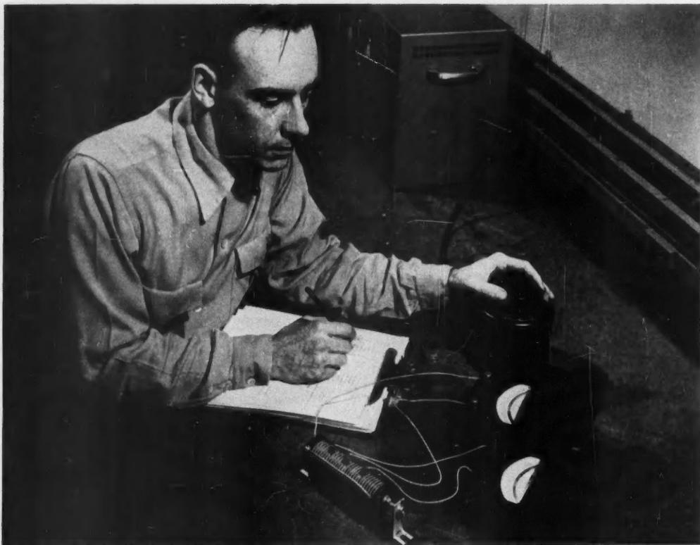
THE TEST FOR FORWARD VOLTAGE DROP OF RECTIFIER REQUIRES ONLY VARIABLE A-C SUPPLY, A-C VOLTMETER AND D-C AMMETER
