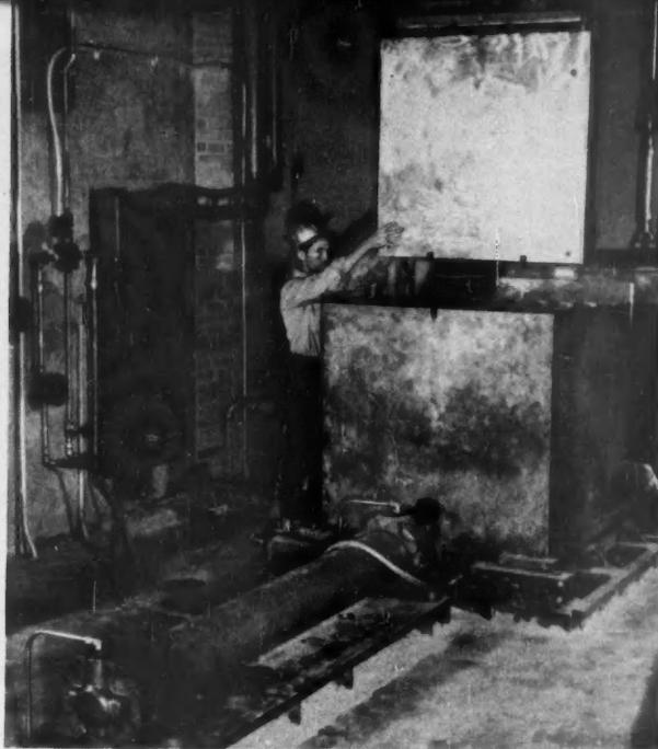
**NUCLEAR EFFICIENCY** of the reactor shielding materials is studied in this developmental facility at Hanford
