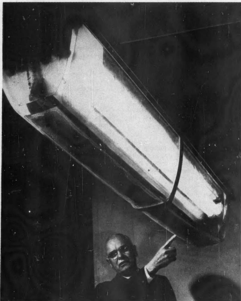
**SIX-FOOT STREET LIGHT** is a new fluorescent unit that doesn't blink or flicker and lights promptly after being turned on. No external starter is used
