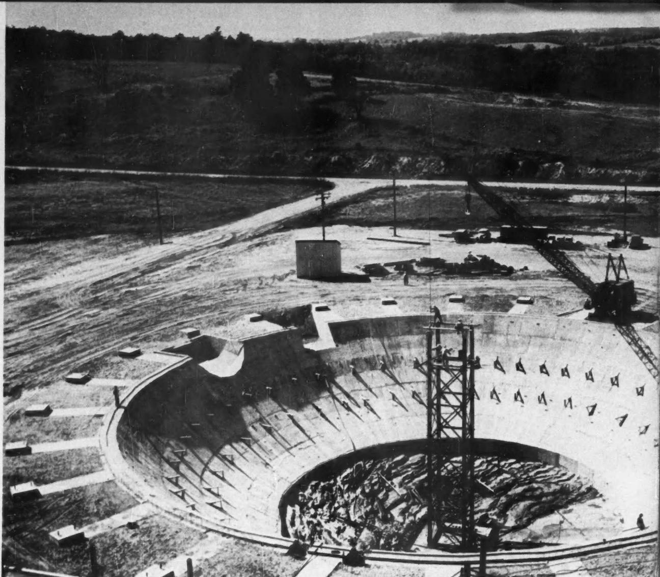
CONCRETE SAUCER IS THE FOUNDATION FOR A 225-FOOT STEEL SPHERE, LARGEST EVER CONSTRUCTED, THAT WILL HOUSE AN ATOMIC POWER
