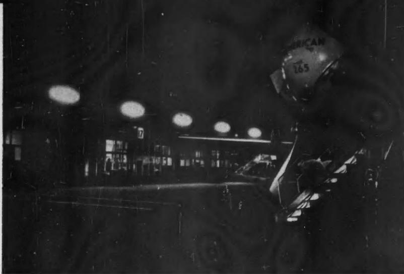
**FLUORESCENT FLOODLIGHTS** allow faster passenger loading and maintenance work. Each aluminum fixture contains two eight-foot-long fluorescent lamps
