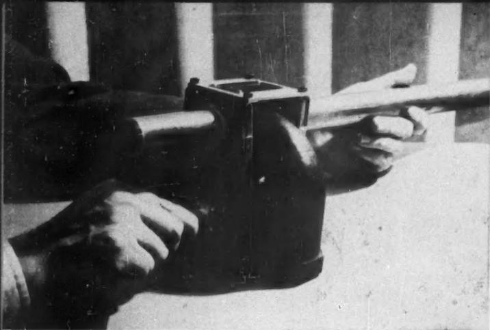
**MAGNETIC FLOWMETER** is completely external to the conducting pipe. It measures the flow of molten metals such as sodium
