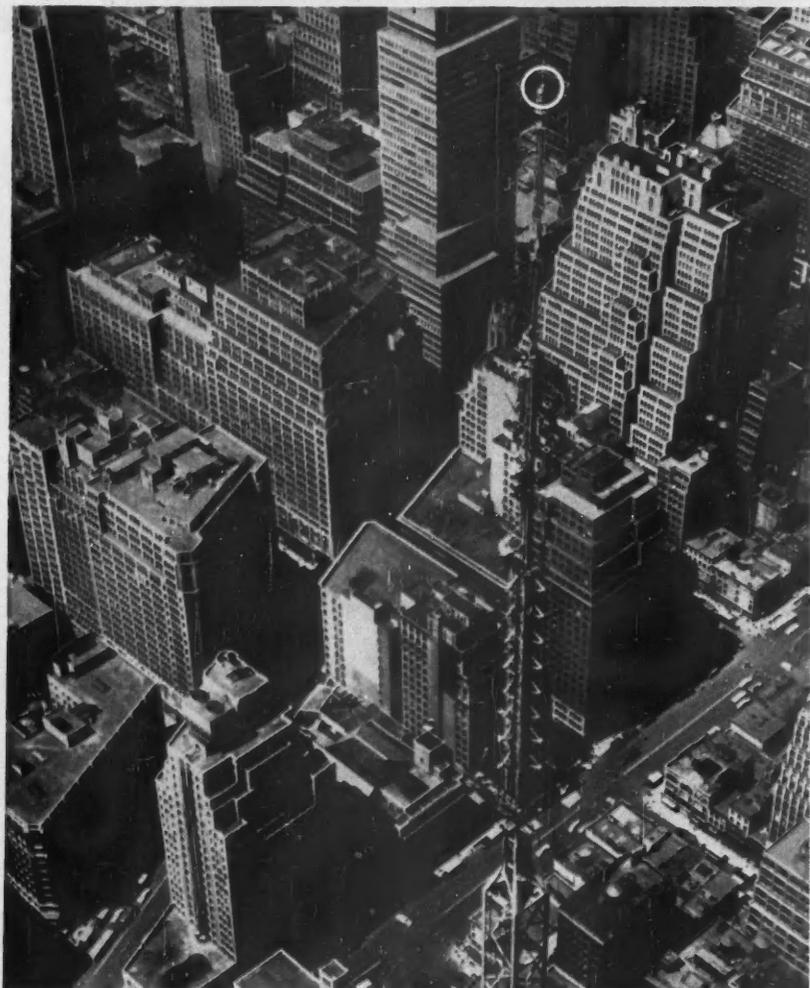
**HARD GLASS LAMPS** installed in red beacon unit atop Empire State Building's TV antenna (top) are heat and shock resistant. Aviation beacon (circled) must withstand bad weather. Ordinary lamps were replaced after hard storms
