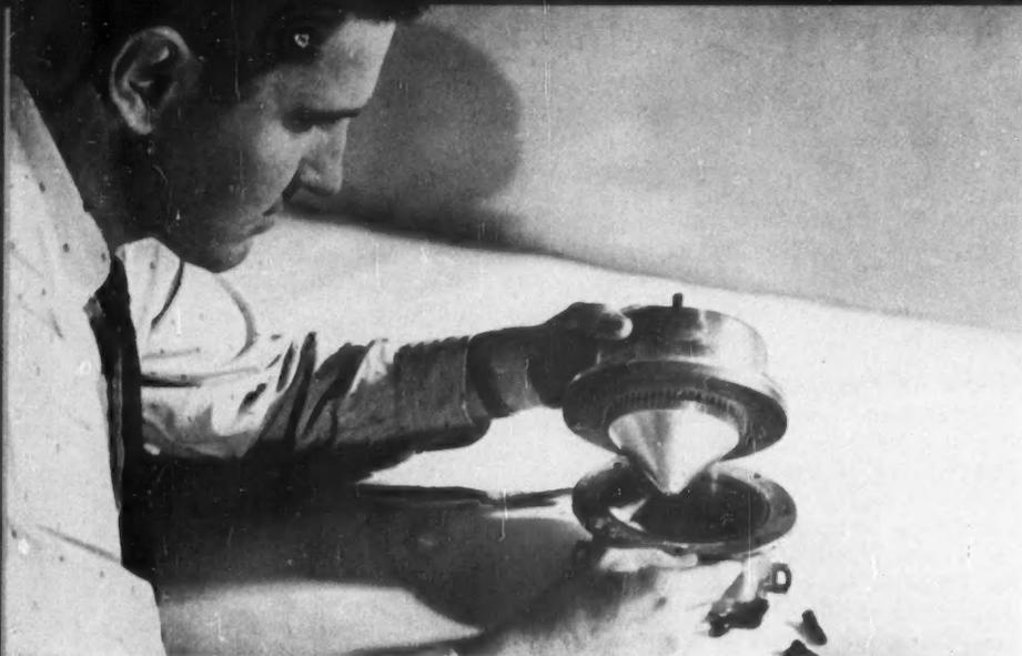
**MERCURY JET SWITCH** monitors 48 thermocouples at a rate of 480 per second. It is able to expand to scan additional couples at the same rate
