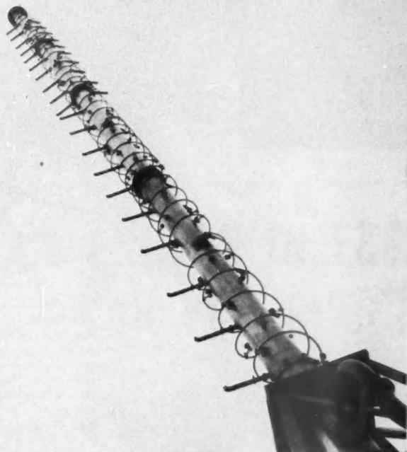
**SIDEFIRE HELICAL** type of UHF-TV high-gain transmitting antenna to operate at 500 megacycles. Power gain is 20 over a dipole—each of the four 10-foot sections shown have a gain of five. Unit has a 50-kw input that equals 1000-kw ERP (effective radiated power).
