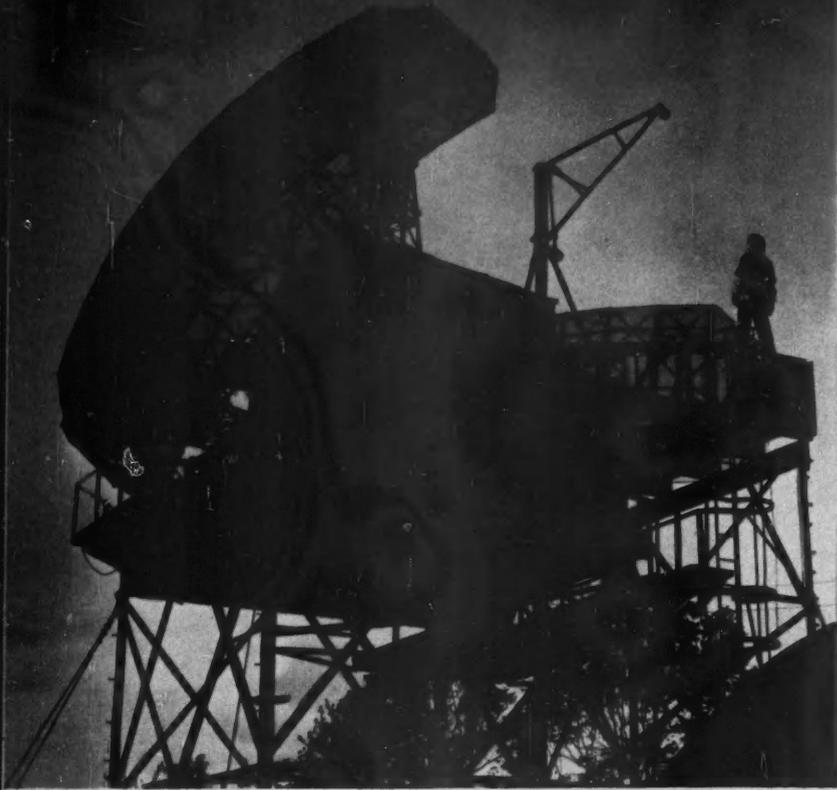
**ELLIPTICAL** antenna of this aircraft detection station has "sails" of lace-like steel to cut down wind resistance. Radomes of rubberized fabric often cover these antennas to protect them from weather.
