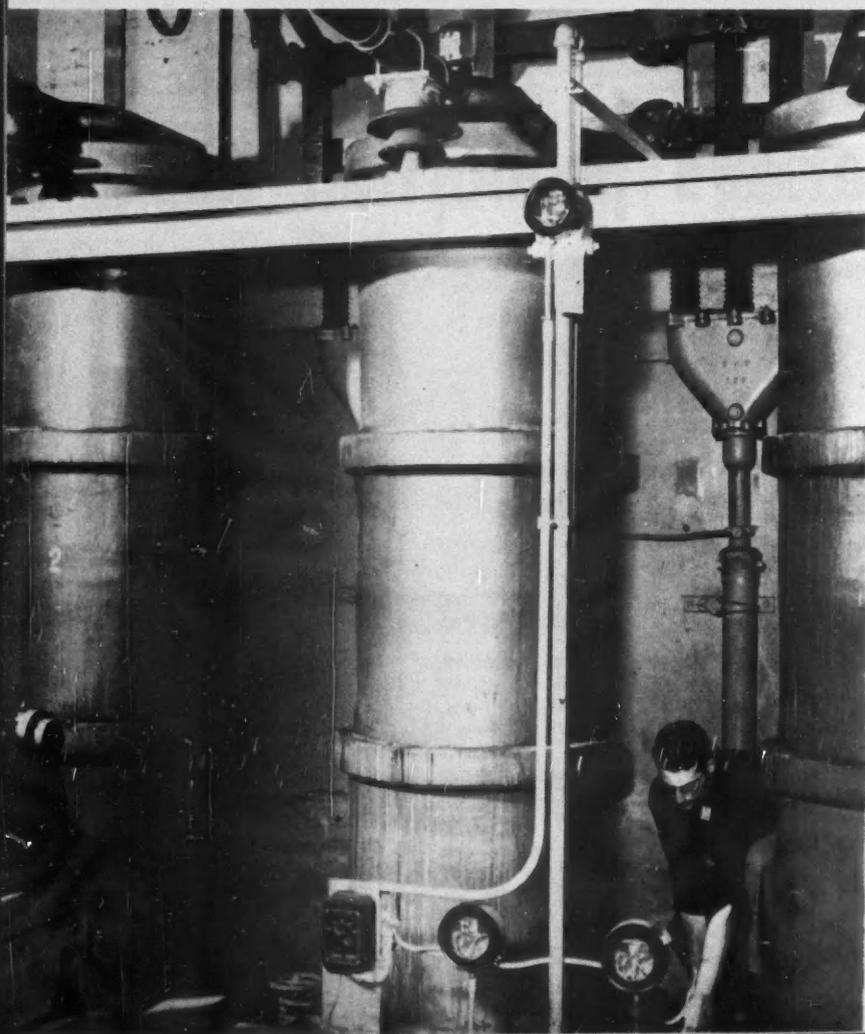
**NEW** There's no steaming in the new indoor liquid rheostat, for the average liquid temperature is well below the boiling point. It converts electric energy to heat in three columns of circulating brine cooled by river water. Resistance of each phase is changed by varying column height. A 45 F decrease in normal cooling-water temperature almost doubles its capacity over the old rheostat.
