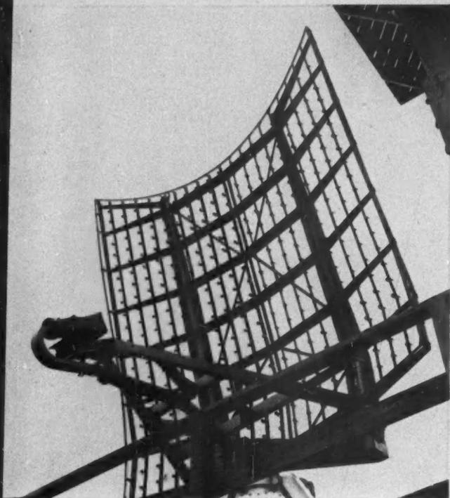
**COSECANT SQUARED** "dish" is used on this airport surveillance and search-type radar antenna for both receiving and transmitting. The antenna gain is 15 and it operates at 2700 to 2900 megacycles with a wave length of 10 centimeters. Output of the radar system is 500,000 watts.
