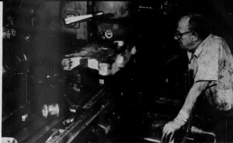
**SHOCK STRESSES** of milling operation are absorbed by rotating steel cutter. Carboloy carbide tips do cutting. The low impact-resistance of early tungsten carbide was a problem.
