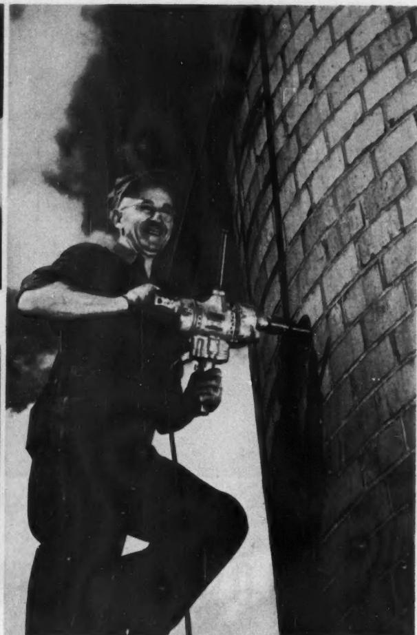
**CARBIDE-TIPPED** drill bores clean holes in masonry and retains its sharpness up to 50 times longer than a conventional steel bit.
