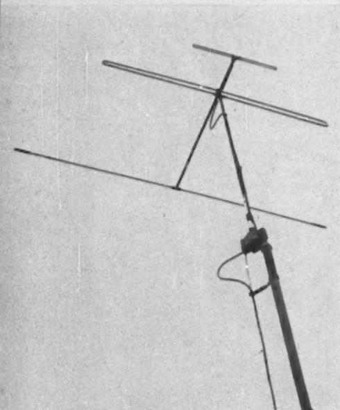
**INLINE** antenna consists of a Hi-band and a Lo-band folded dipole with one reflector. It is used in primary service areas where TV reception is good. One of the unusual features of this antenna that improves its performance is that the Lo-band folded dipole is used as a reflector for the Hi-band dipole.
