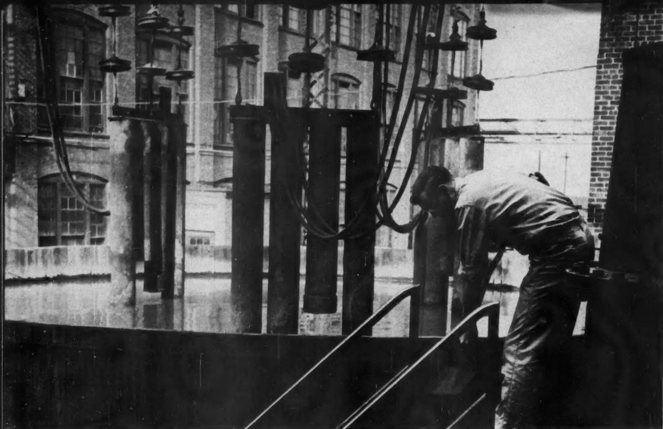
**OLD** Conventional three-phase water-box rheostat (above) dissipates power from the test generator as the current flows between the partially submerged electrodes and boils the water. Salt is added to increase the load. Billows of steam blanket the actual operation and the surrounding areas.
