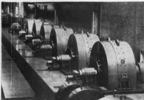
These D.C. motors, totalling 20,500 hp—built at the Peterborough Works of Canadian General Electric—drive Canada's largest continuous hot-strip steel mill.
