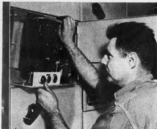
**EASY TO INSTALL,** inspect, and interchange starters, which are assembled as complete units, including pushbuttons and wiring terminals for easy front-connecting. Door swings more than 90°
