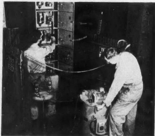
**HIGH-POTENTIAL TESTS** are made of each completed General Electric control center before shipment, to assure adequate short-circuit protection, safety for plant personnel and equipment.
