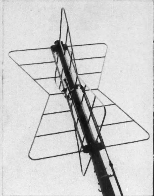
**BAT WING**, also known as a "super turnstile," is a TV transmitting antenna for low-channel (2) operation. Only one bay is shown, but stacks of three to six are used on low channels; six, eight, or twelve bays on high channels.
