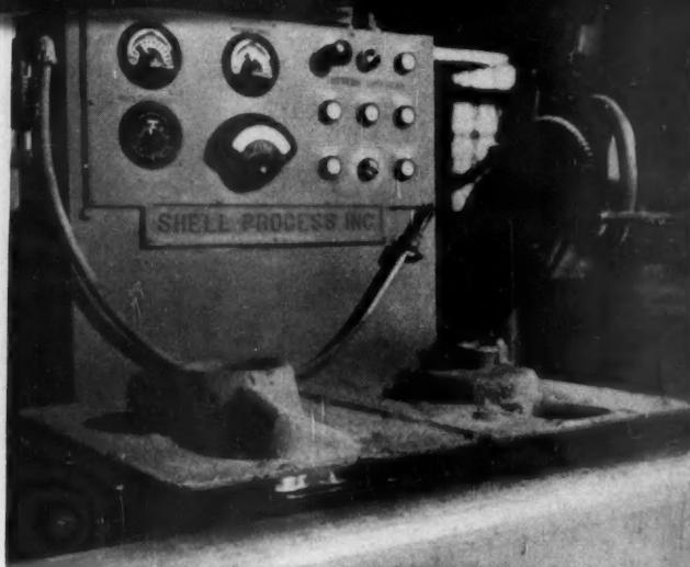
**5** The pattern moves from investment box to the oven; there the dough-like mass is baked to a hard shell. When done, its color will vary from bright yellow to dark brown. A final shift back to the ejection station and the hardened shell (above) is "stripped" from its pattern. This is done by an ejector plate that applies upward pressure against knockout pins. After this operation . . .
