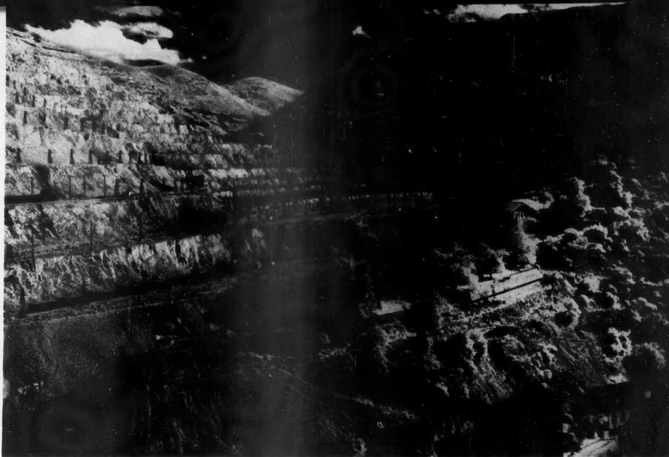
MOUNTAIN OF COPPER ORE, BINGHAM CANYON, UTAH—REMOVAL OF 135,000 TONS OF ROCK PRODUCES 92,000 TONS OF ORE DAILY.
