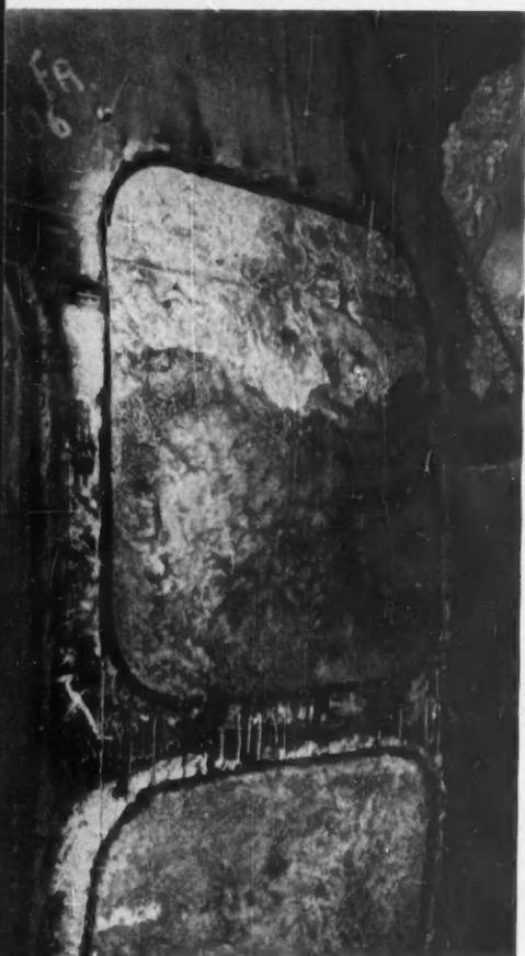
**3** Cover plates removed to show how plastics foam assumes shape and fills void spaces. Highly buoyant foam keeps carrier from listing in event of a shell hit.
