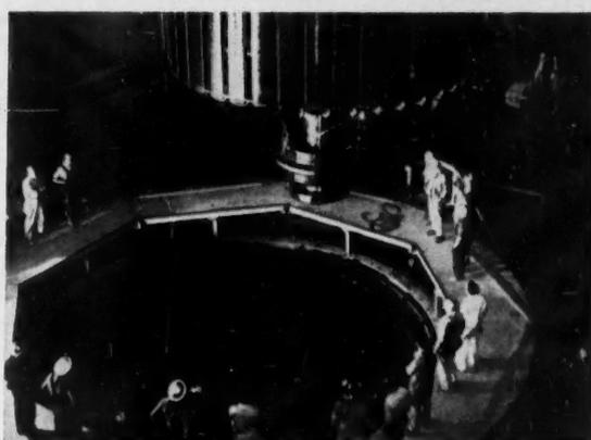
**MORE AUTOMATIC VOLTAGE CONTROL.** G-E engineers applied amplistats in the voltage regulator system for this giant alternator, being positioned at a hydro-electric installation.
