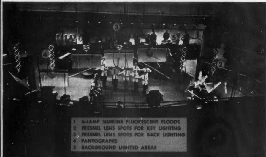
TV LIGHTING EFFECTS ARE OBTAINED BY COMBINATIONS OF WELL-DESIGNED EQUIPMENT.
