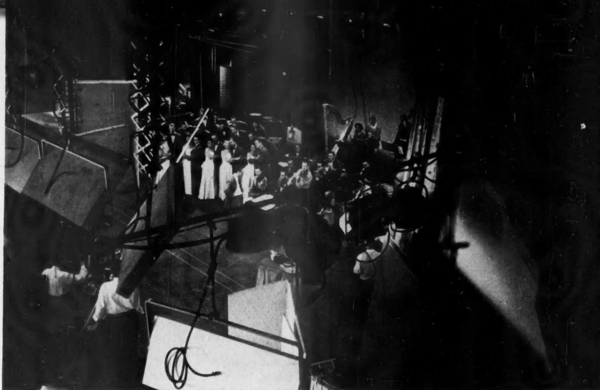
**MODERN TV LIGHTING** offers flexibility and efficiency. Contrast the highlights on hair and shoulders of performers in the Fred Waring program (*above*) with the lighting of an early installation at WRGB, Schenectady (*right*). Overhead lighting with fluorescent lamp banks and Fresnel lens spotlights combine to effectively provide base, back, and key lighting, replacing water-cooled mercury lamps.
