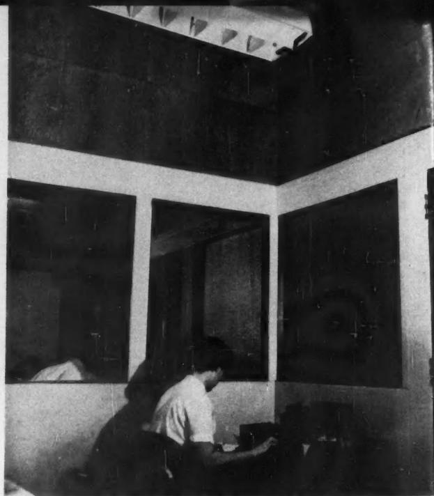
**INTERCONNECTED** cells of phenolic foam make it an ideal acoustical insulation. In closely grouped offices, the clatter of office machines is deadened by slabs of foam placed between partitions and ceiling.
