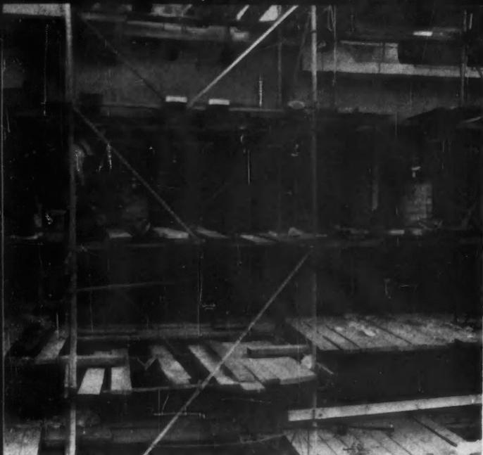
**1** Filling blister voids of an aircraft carrier—14 feet above and below water line—with phenolic foam. Electric mixer beats air into the liquid resin, then catalyst is mixed in. Ten seconds later the mixture is sent down wooden chute and workers move away, as . . .
