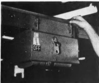
**POWER TAKE-OFF PLUG** is utilized in a plug-in-type busway distribution system.
