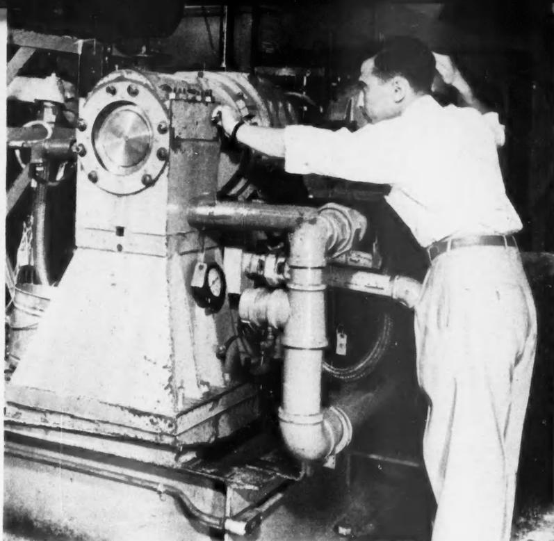
OIL WHIP IN HIGH-SPEED JOURNAL BEARINGS IS STUDIED ON THIS TEST STAND.
