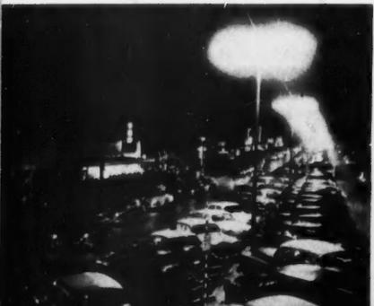
COMFORTABLE SEEING is provided by the low-brightness of fluorescent luminaires even where low mounting height is necessary—such as in the amusement park below (left) and the mile-long, high-speed viaduct (right). Tunnels and underpasses are ideal locations for fluorescents.
