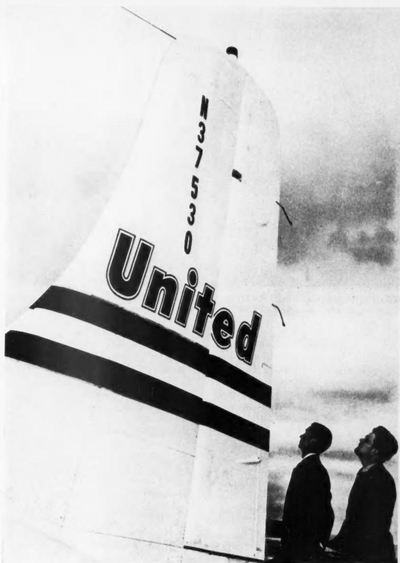
**HIGH-INTENSITY BEACON** mounted on the vertical fin of an airliner increases air safety. A fixture rotates the beam horizontally making it visible from all points of the compass.
