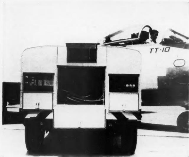
**MOBILE POWER SUPPLY** for aircraft—a 400-cycle a-c alternator rated 30 kva—is complete with its own regulated d-c power supply.
