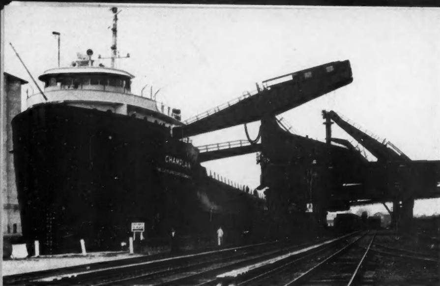
ORE UNLOADER USES SEVERAL REMOTELY CONTROLLED ADJUSTABLE-VOLTAGE D-C DRIVES.
