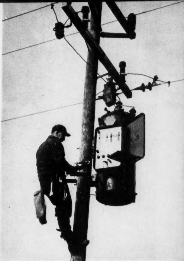
**VOLTAGE REGULATOR** designed for urban lines provides 10 percent higher and lower range of regulation in 32 steps.
