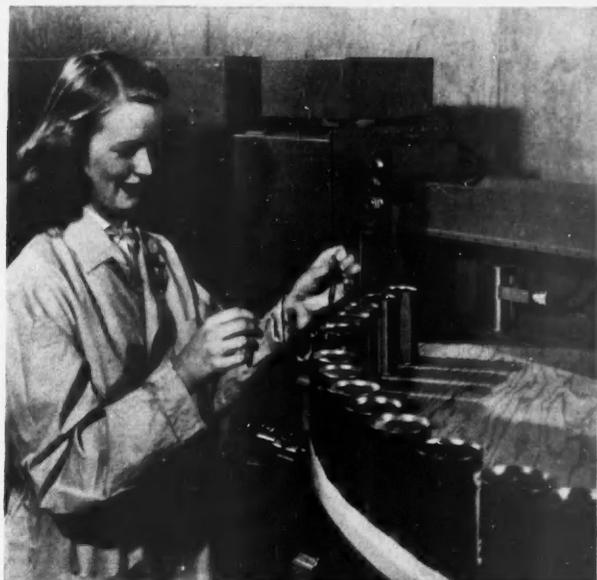
**LIQUID-LEVEL CHECKER** used in canning industry inspects 900 containers per minute and detects levels to one thirty-second inch.
