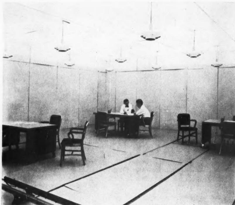
**FLEXIBLE TEST ROOMS** to study fundamentals in lighting design have adjustable walls and ceilings. Extensive measurements of actual and representative lighting systems are made.
