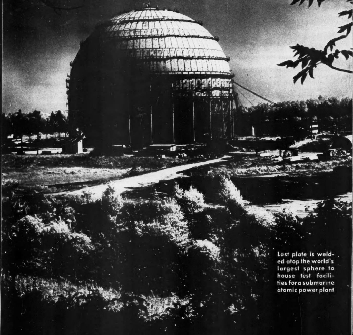
Last plate is welded atop the world's largest sphere to house test facilities for a submarine atomic power plant
