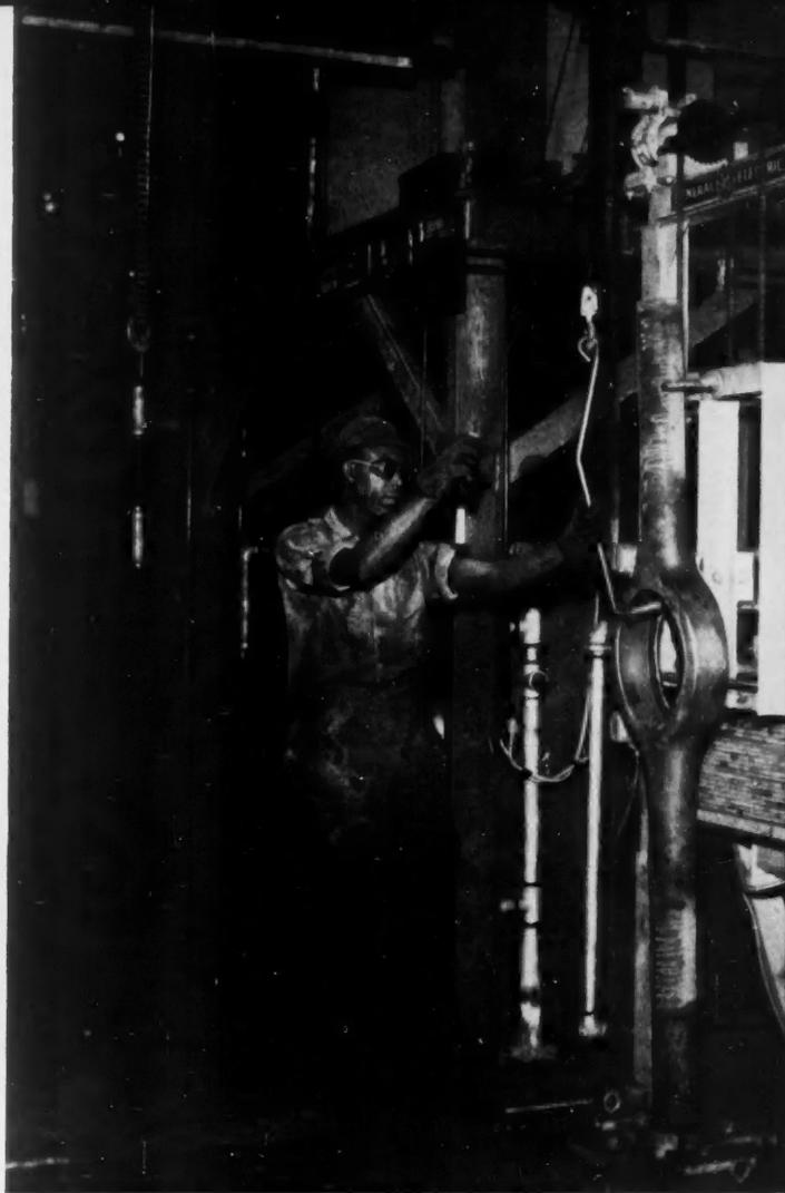
**TO IMPROVE WORKING CONDITIONS**, G-E engineers concentrate heat required to treat these axle housings, reducing radiation.
