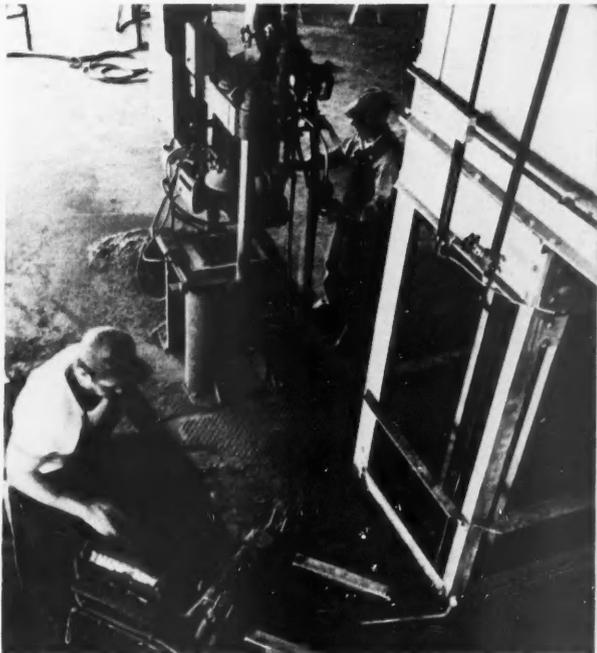
**2** From silos, sand drops to mezzanine floor where it is milled, then dropped to core-making area. Cores are formed, then . . .
