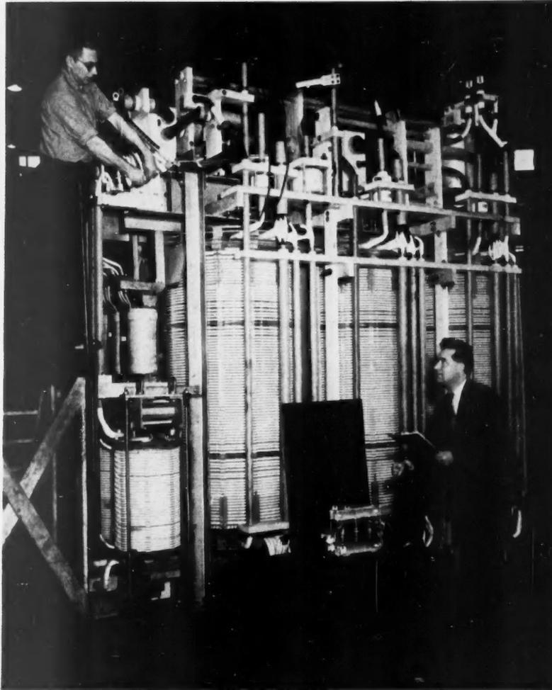
PLACEMENT OF INSULATION IN THIS 20,000-KVA TRANSFORMER WAS AIDED BY ONE-TWELFTH SCALE MODEL OF UNIT. AUTHOR IS AT RIGHT.
