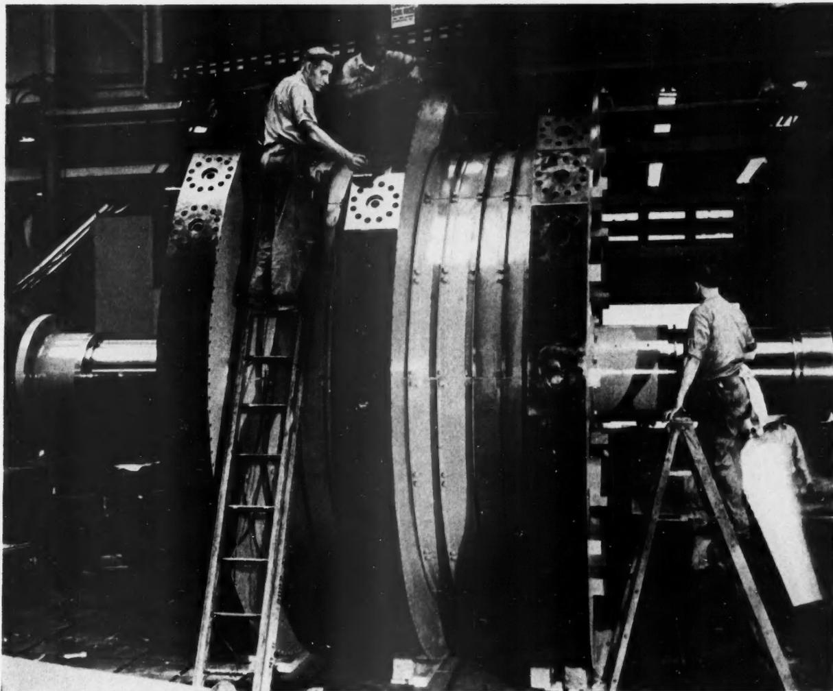
PROTECTIVE TECTYL COMPOUND IS APPLIED TO THE 122½-TON WIND-TUNNEL FAN ROTOR BEFORE IT BEGINS THE 4750-MILE JOURNEY.
