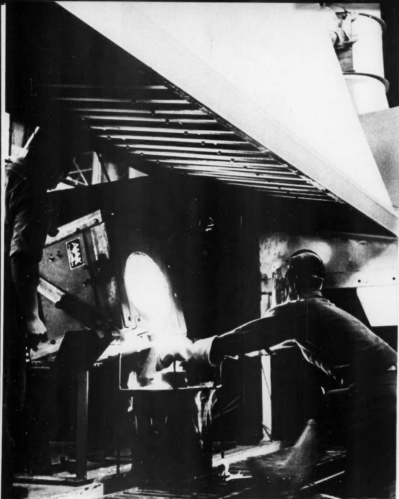
**4** As metal ingredients for magnets are melted down in electric furnaces, stacked cores are conveyed to pouring position. Test bars from each heat are immediately analyzed by a direct-reading spectrometer and by the metallographic laboratory.
