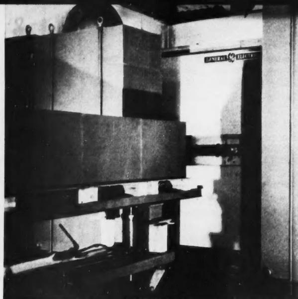
AUTHOR ADJUSTS NEUTRON-COUNTING ELECTRONIC APPARATUS USED IN CONJUNCTION WITH THE 100-MEV BETATRON (RIGHT) TO DETERMINE . . .
