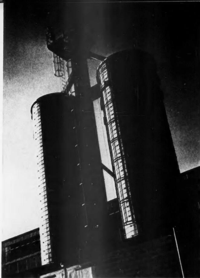
**1** Each silo holds 250 tons of dry sand used in making magnet cores. In each are 30 tons of "live" sand immediately available. Remainder is in storage.
