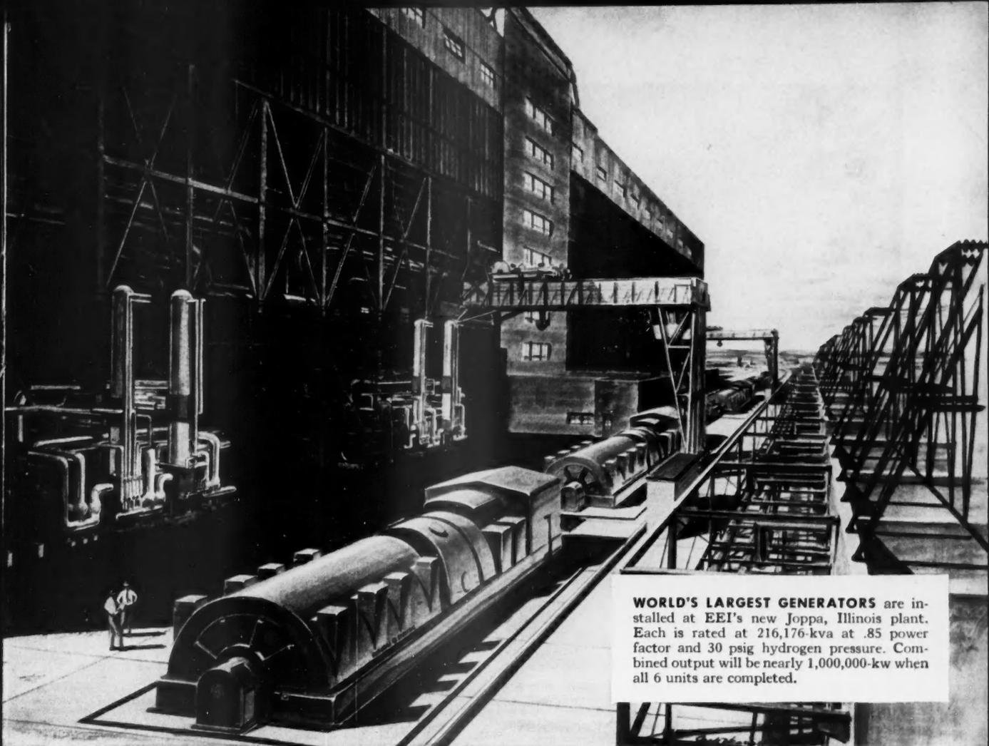
**WORLD'S LARGEST GENERATORS** are installed at EEI's new Joppa, Illinois plant. Each is rated at 216,176-kva at .85 power factor and 30 psig hydrogen pressure. Combined output will be nearly 1,000,000-kw when all 6 units are completed.
