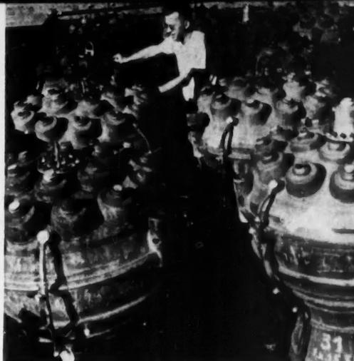
**V-2 MOTORS** burned liquid oxygen and alcohol, developed 50,000 pounds thrust.
