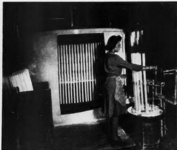
IN THE 30'S LARGE OVENS FIRED PHOSPHORS AND A COATING PROCESS COVERED GLASS TUBES WITH A FLUORESCENT POWDER SUSPENSION.
