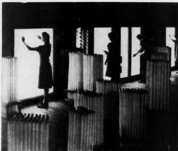
LABORATORY EXHAUST EQUIPMENT TESTS EARLY LAMPS. RACKS HOLD LAMPS WHILE THEY BURN FOR AGING PURPOSES.
