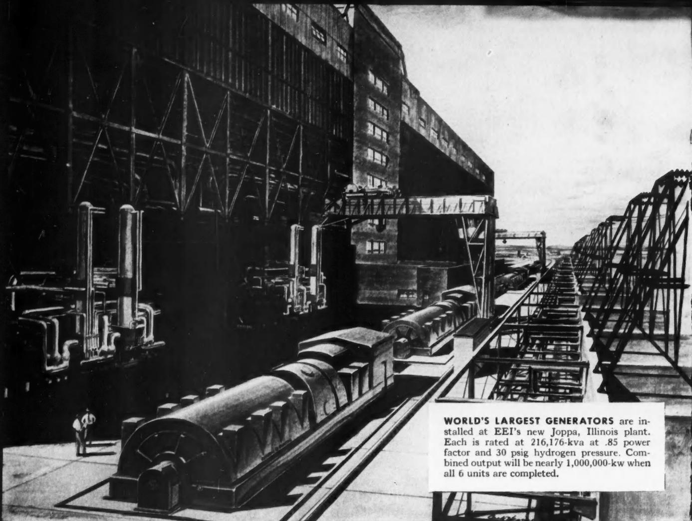
**WORLD'S LARGEST GENERATORS** are installed at EEL's new Joppa, Illinois plant. Each is rated at 216,176-kva at .85 power factor and 30 psig hydrogen pressure. Combined output will be nearly 1,000,000-kw when all 6 units are completed.
