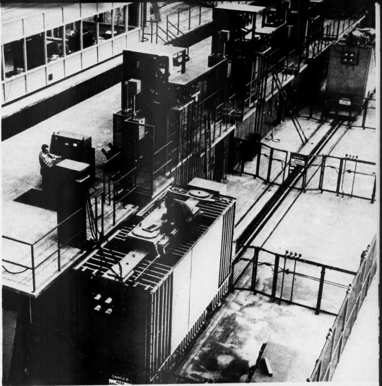
**TESTING** is also done on a production-line basis (*above*). Each operator does his own particular test when a unit stops in his berth. After final inspection, transformers are loaded on flatcars at end of production line, sent on their way to final destination.  $\Omega$
