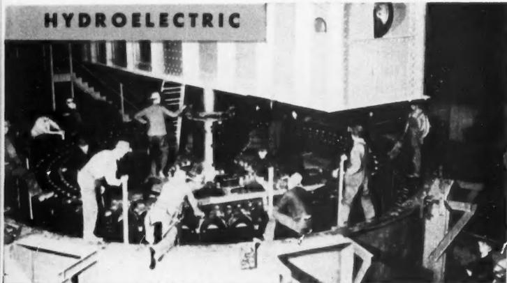
**HYDRAULIC** turbine-driven generators, similar to this 75,000-kw unit being installed at California's Shasta Dam, utilize the amplistat. Since 1948 their a-c output voltages have been accurately and dependably regulated by an amplistat in combination with an
