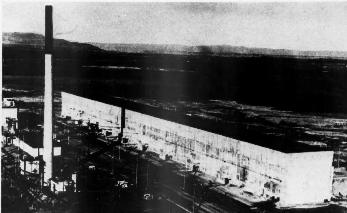
HIGH-DENSITY CONCRETE FOR BULK SHIELDING IS USED IN MANY OF THE FACILITIES AT GE'S HANFORD ATOMIC PRODUCTS OPERATION.
