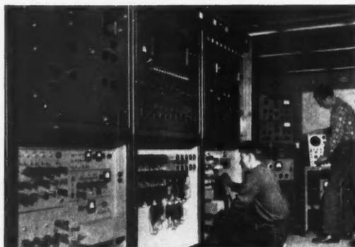
*Television transmitter undergoing final tests at Royce Works before shipment to a new Canadian television station.*
