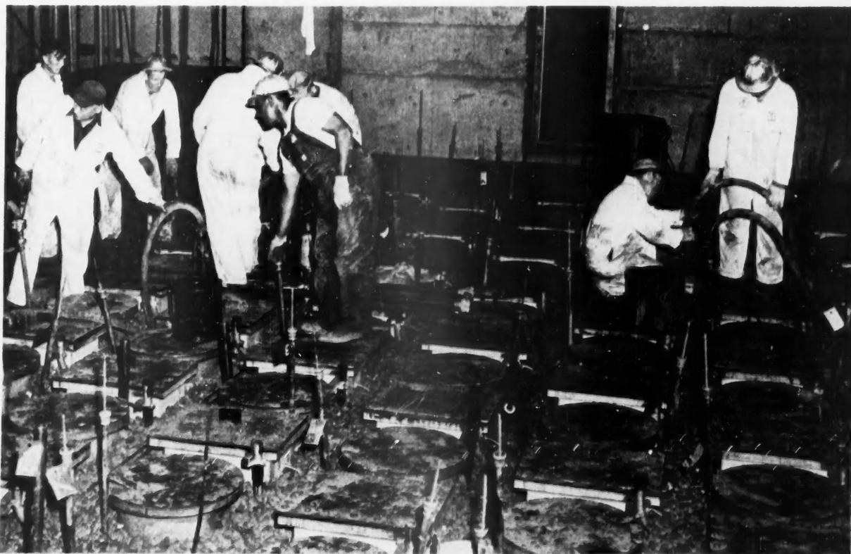
IN THE NEXT STEP, PUMPS FILL VOID IN THE AGGREGATE MASS WITH AN INTRUSION MORTAR OF CEMENT, HIGH-DENSITY SAND, AND WATER.
