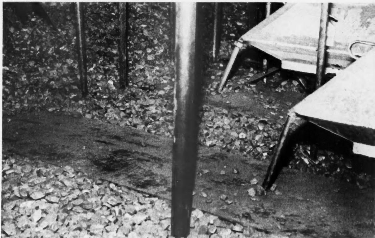
MAGNETITE-LIMONITE AGGREGATE IS PLACED IN LESS CRITICAL AREAS OF A SHIELD (FOREGROUND), STEEL AND LIMONITE AROUND BEAMS.
