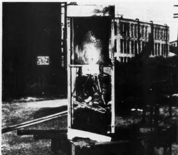
DESPITE HIGH TEMPERATURE OF FIRE TEST, PRESSURE BUILD-UP WAS MINOR WITH NEW COMPRESSOR. THE COOLER PASSED ITS FINAL EXAM.
