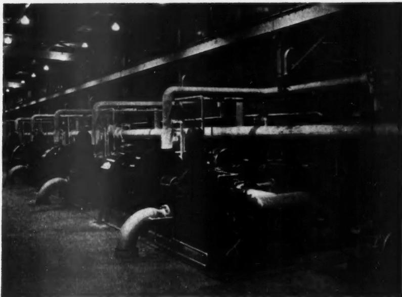
**MAIN PUMP SETS** supply coolant for the reactor's high transient flow requirements. Each set consists of a steam-turbine-driven pump in series with an electric-motor-driven pump.
