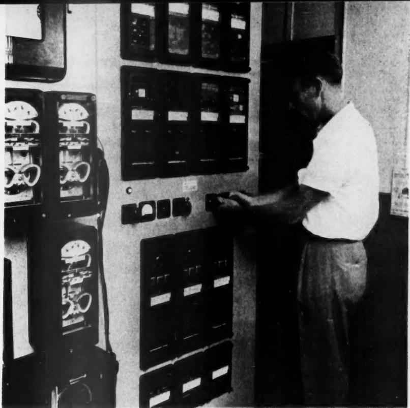
**CARRIER RELAYING PANEL** is part of two complete terminals of all-electronic relays installed to protect the 132-kv line owned by the Appalachian Electric Power Company.
