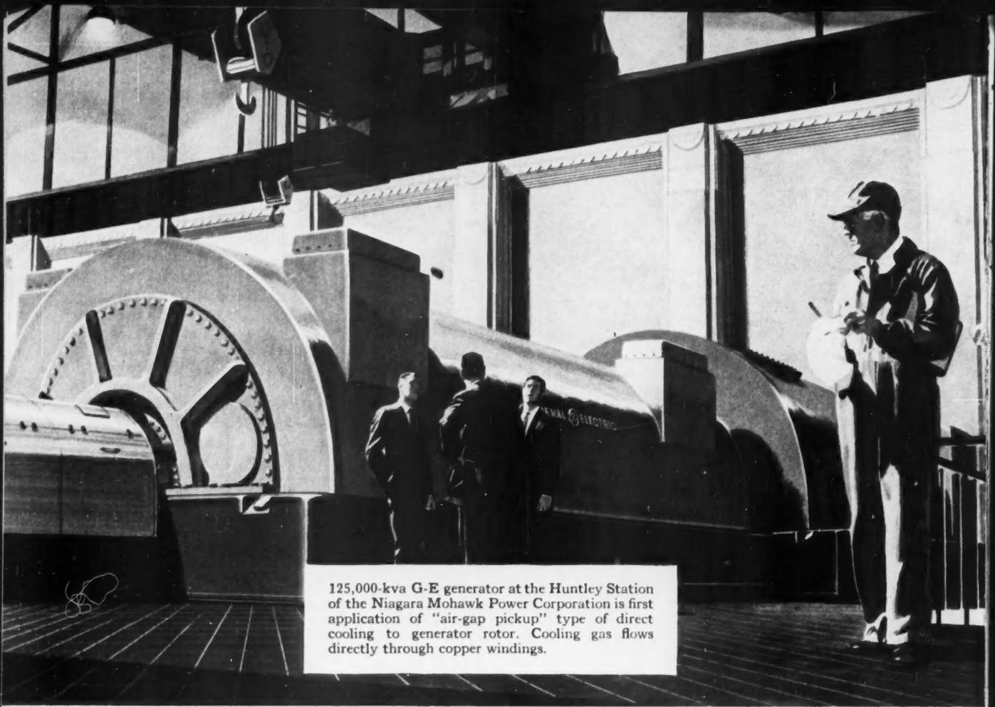
125,000-kva G-E generator at the Huntley Station of the Niagara Mohawk Power Corporation is first application of "air-gap pickup" type of direct cooling to generator rotor. Cooling gas flows directly through copper windings.
