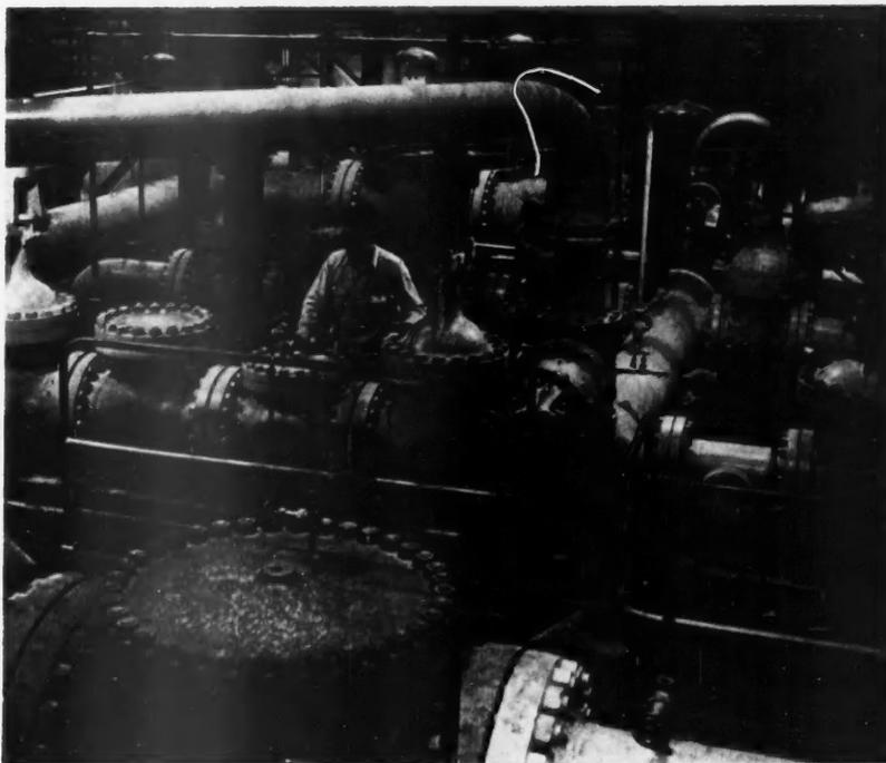
**VALVE PIT** is the cooling-water diversion point where coolant from main pumps is directed through the reactor and to other points, such as control rods, where energy is generated.
