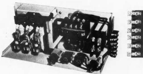
Control unit showing neat arrangement for easy maintenance. Type "B" Terminal Blocks (shown right) permit unit to be removed without disturbing wiring. Notice the fusible disconnect that can accommodate either or both Type NEC or Type CLF current limiting fuses.
