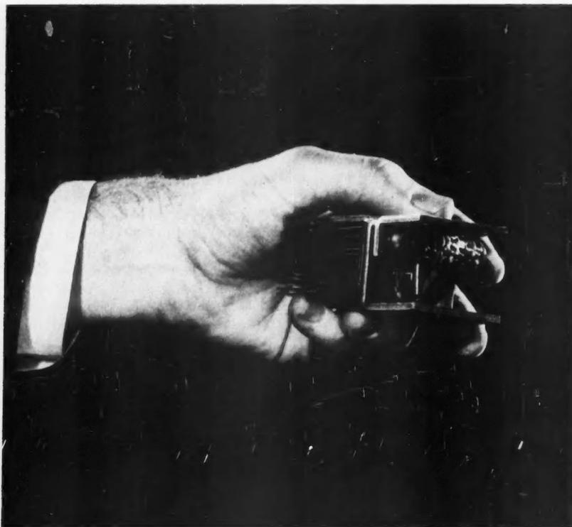
**HEART** of this 2000-watt rectifier cell is a wafer of germanium the size of a dime. The complete unit, including cooling fins and mounting brackets, weighs only 12 ounces.
