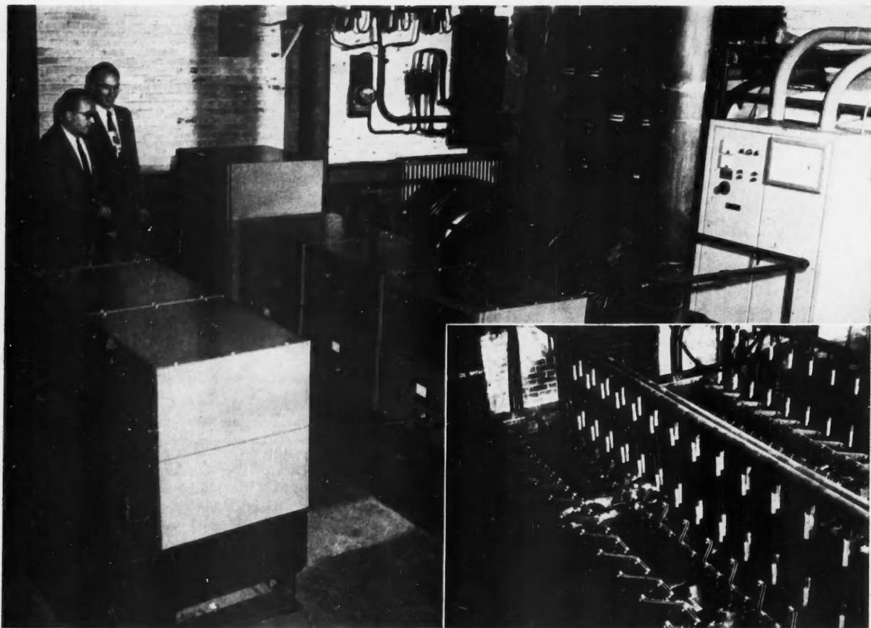
**APPLICATION** typifying great flexibility of germanium rectifiers is used in hydrogen-oxygen plant. Interchangeable with motor-generator set or incoming power at control panel, six 25-kw rectifiers supply 1200-amp 125-volt d-c power to 80 cells in adjoining room (*inset*).
