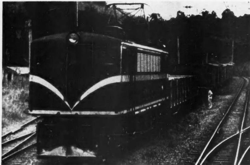
**ELECTRIC LOCOMOTIVES** on the meter-gauge Sorocabana Railroad, operated by the State of Sao Paulo in Brazil, have more than doubled the capacity of the line over steam operation.
