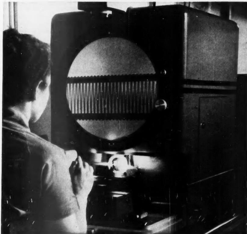
OPTICAL COMPARATOR HELPS DETECT ANY DEVIATION FROM MANUFACTURING TOLERANCES.
