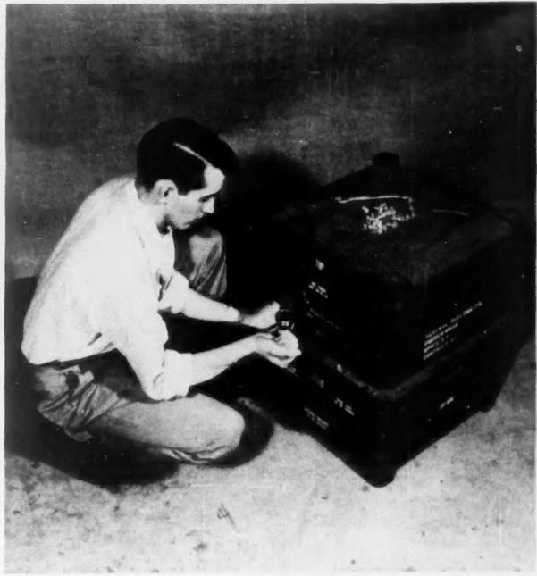
PRESSURE-RELIEF VALVES ARE PROTECTED BY COVER ON CONTAINER FRONT. BOLTING COMPLETES JOB. NEW WAY IS 80 PERCENT TIMESAVER.
