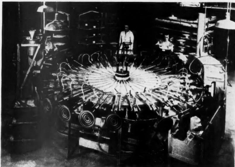
**AUTOMATIC GLAZING MACHINE** controls glaze thickness and uniformity within extremely narrow limits to obtain maximum strength from the glaze and porcelain combination.
