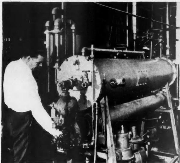
**EXOTHERMIC-GAS PRODUCER**—the most common atmosphere-gas generator—burns inexpensive hydrocarbon fuel gases mixed with air.
