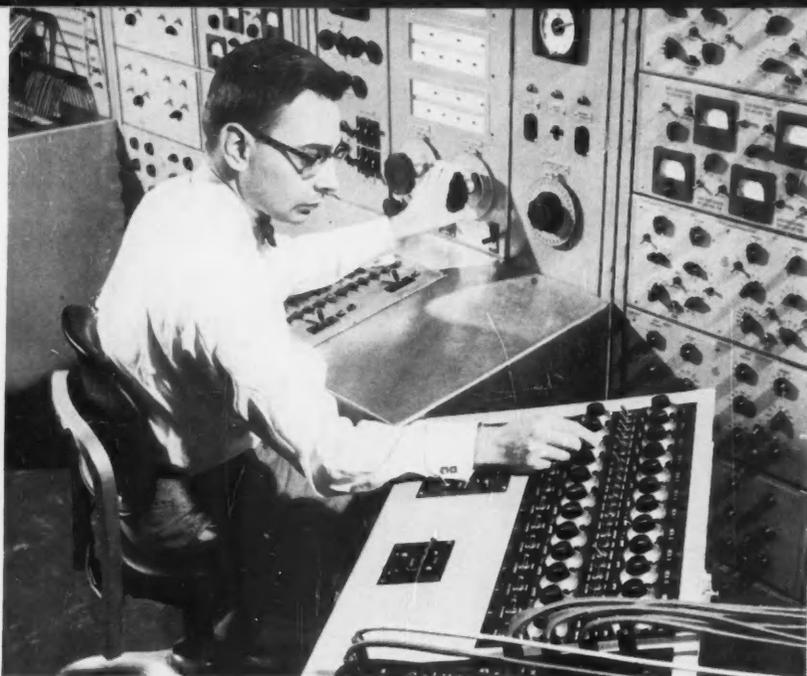
ENGINEERS PLAN EFFECTIVE SYSTEM PROTECTION WITH AID OF SWING CURVE CALCULATOR.
