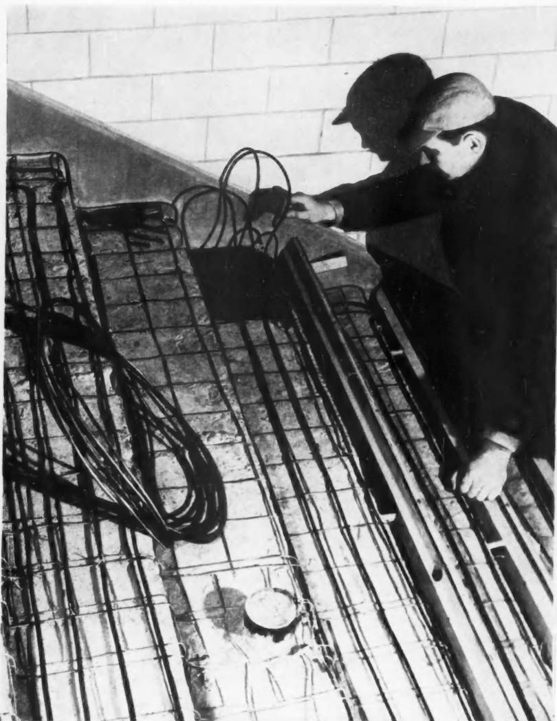
**INSTALLATION OF HEATING CABLE** embedded in the steps of the Pennsylvania Railroad's Suburban Station in Philadelphia keeps stairways free from ice and snow.
