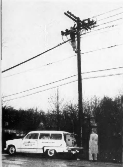
**HIGH-VOLTAGE** d-c cable test unit is mounted in station wagon for field service.
