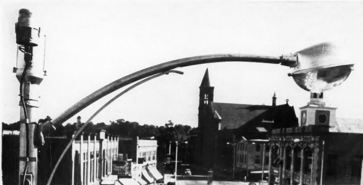
TWO DIFFERENT LIGHT DISTRIBUTIONS ARE AVAILABLE BY MERELY CHANGING SNAP-IN REFLECTORS IN MERCURY STREET-LIGHTING DEVELOPMENT.
