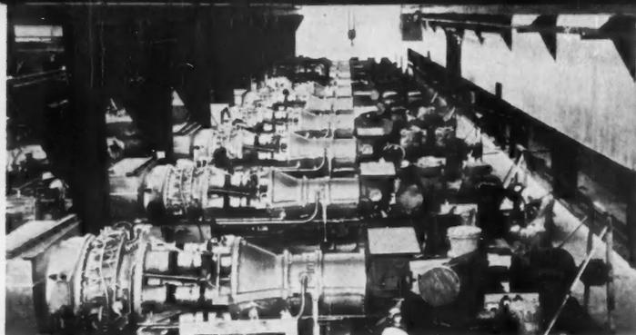
**TEN SIMPLE-CYCLE** 2-shaft gas turbines began operation in a Venezuelan oil-field pressure-maintenance project on a platform in Lake Maracaibo.
