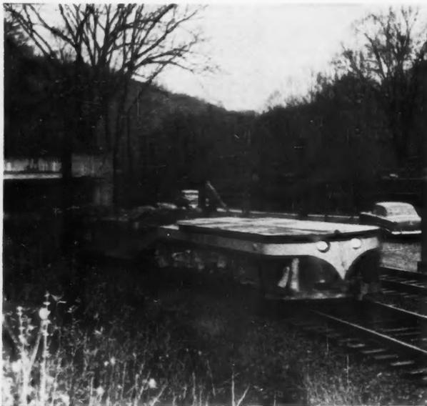
**LARGEST MINING LOCOMOTIVE** for underground service, capable of hauling record tonnages of coal, is 35 feet long and 4 feet high.
