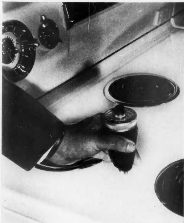
**FILM-THICKNESS GAGE** utilizes new principle to measure coatings on magnetic materials from 0 to 0.060 inch thick.
