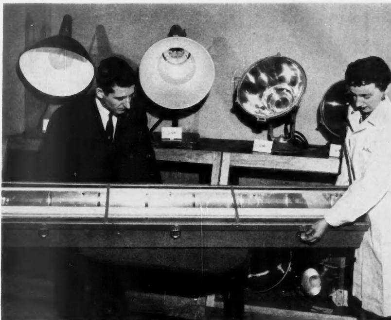
**FLOODLAMPS**—tungsten, mercury, and fluorescent—fill a specific need in architectural lighting. Using reflectors in fixtures concentrates the light in definite beam patterns.
