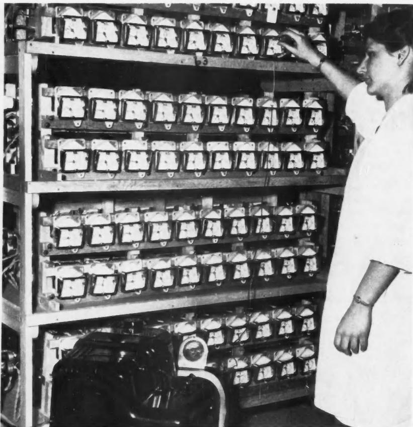
**EACH MOTOCHRON CLOCK** undergoes a timekeeping test. The impulses of the clock's escapement are picked up by a microphone and then amplified and recorded for observation.
