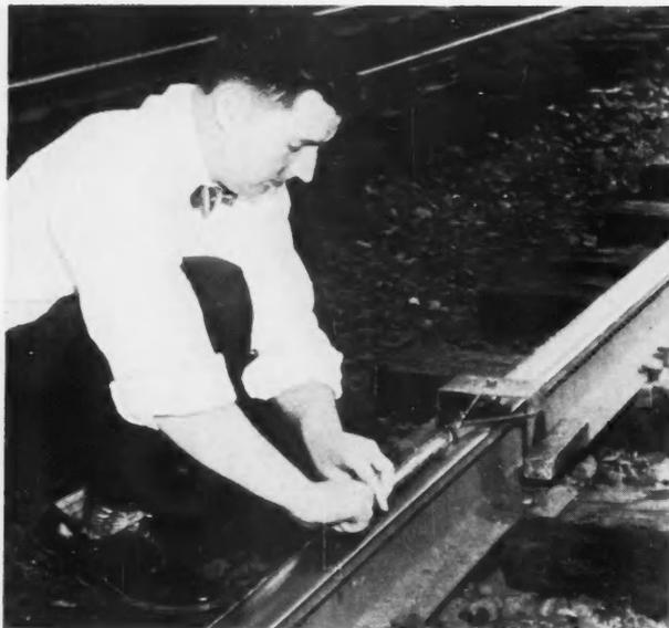
**TO SUBSTANTIATE** laboratory findings on the importance of oil films, test equipment was modified for use on actual railroad track.
