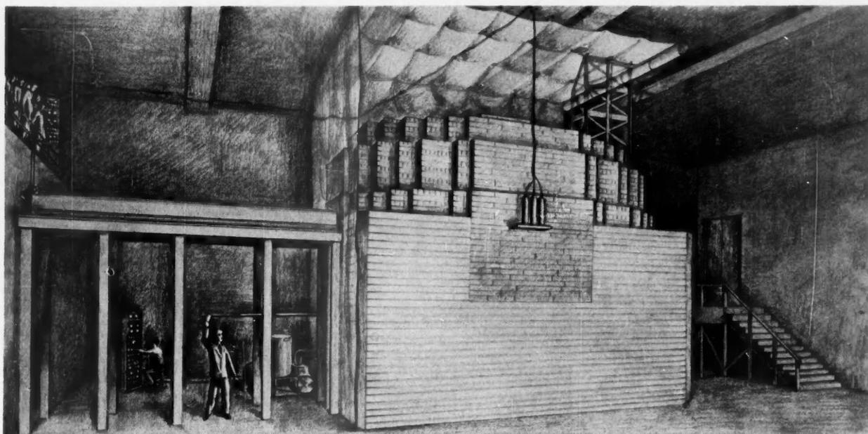
FIRST NUCLEAR REACTOR, ERECTED IN 1942 AT THE UNIVERSITY OF CHICAGO, NOW FUNCTIONS AT THE ARGONNE NATIONAL LABORATORY.
