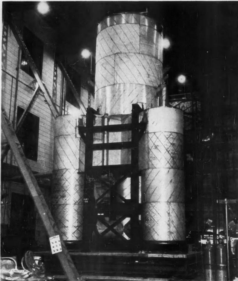
STAINLESS STEEL USED IN THIS 40-TON VESSEL ILLUSTRATES THE APPLICATION OF . . .
