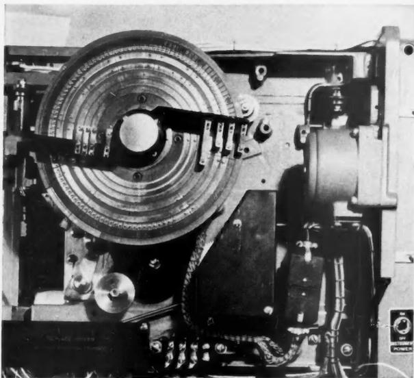
**ANALOG-TO-DIGITAL** converters in addition to the associated relay-network system activate the proper key-punch machine.
