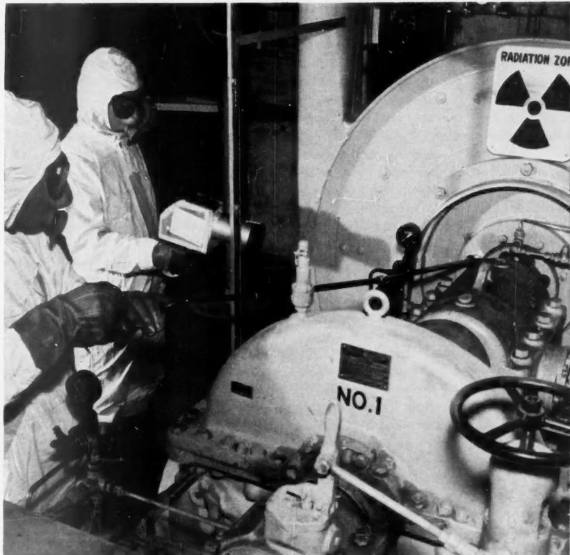
LONG-HANDLED SOCKET WRENCH EXTENDS THE TIME A MECHANIC CAN SPEND ON REPAIR JOB.
