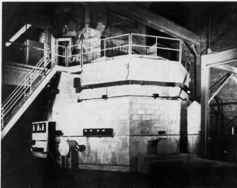
**EBR** Generating about 250 kw of electric power, the Experimental Breeder Reactor was the first to explore fissionable fuel breeding and prove it technically feasible.
