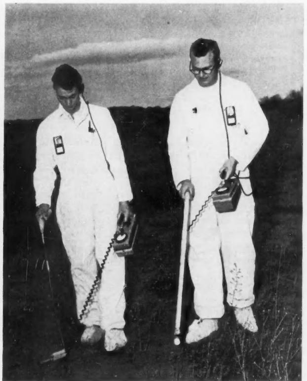
. . . POLICING THE INTERIOR AND THE SURROUNDING AREA TO DETERMINE AND CONTROL THE LEVELS AND ZONES OF CONTAMINATION.
