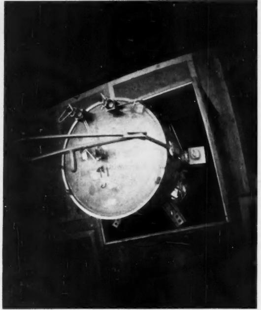
PERISCOPES GUIDE TECHNICIANS AS THEY REMOVE A FAILED VESSEL (RIGHT) FROM ITS WORK LOCATION BY REMOTELY CONTROLLED CRANE.
