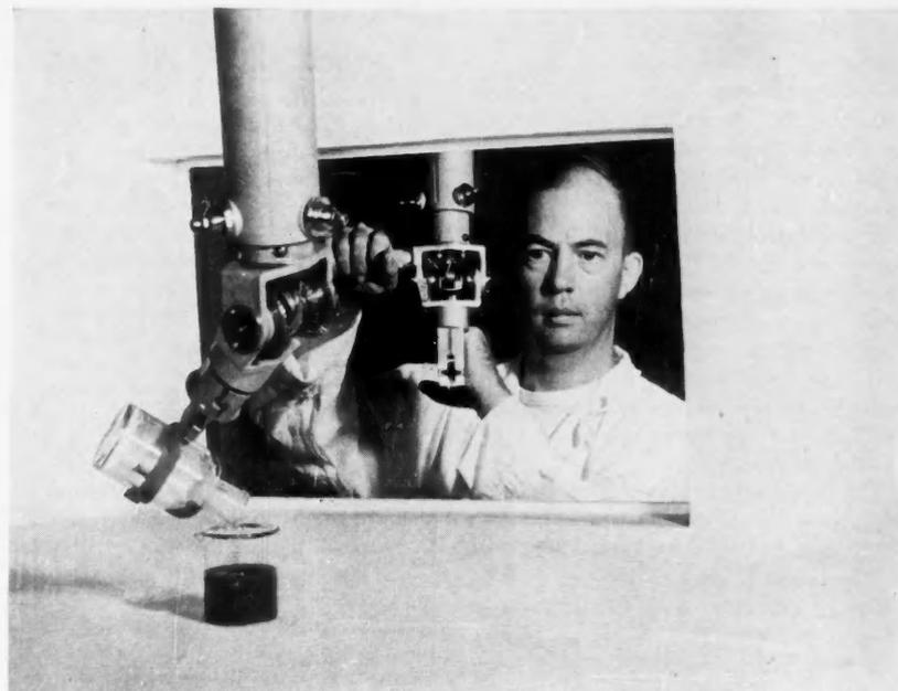
**MECHANICAL HAND**, through control coupling, follows movements of the operator's hands. Forces met by the slave arm are transmitted back, giving operator a feel for his work.
