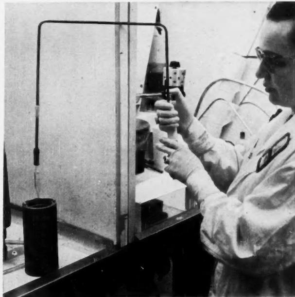
HANDLING EQUIPMENT PERMITS POURING AND MIXING OF HOT SAMPLES AND MEASURES A RADIOACTIVE SAMPLE WITH A REMOTE PIPETTE.
