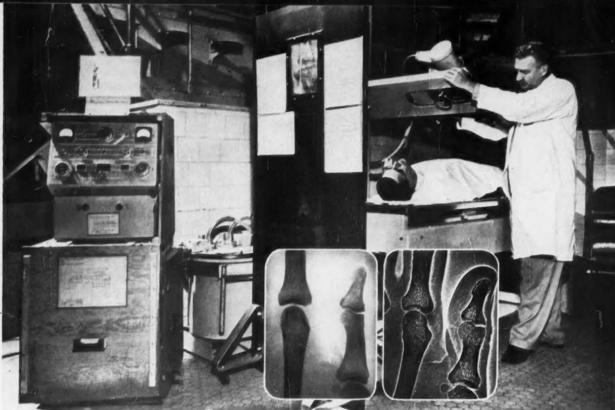
**MOBILE XERORADIOGRAPHIC EQUIPMENT**, using its own packing case as a support, can be set up in any building for emergency purposes in the event of a civil disaster. This process produces a wider range image density (inset, right) than conventional methods.
