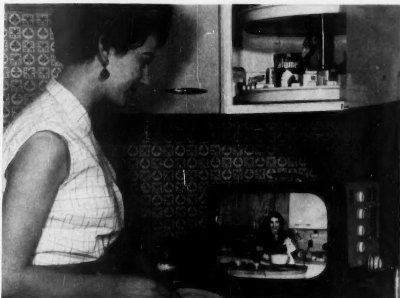
**PORTABLE 14-INCH TV**, symbolizing TV progress, uses 13 tubes and weighs 32 pounds. Five years ago, a 14-inch screen required 22 tubes and weighed more than 100 pounds.
