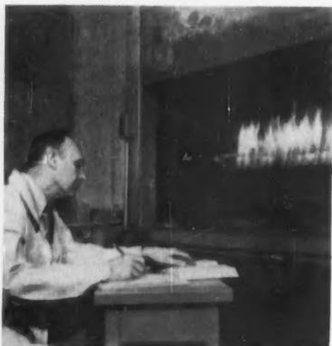
Silicone-rubber insulated cable being subjected to 1400°F flame for 24 hours in laboratory tests. Superior materials and rigid testing go into each G-E cable.
