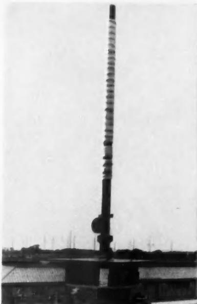
**HELICAL ANTENNAS**, interlaced for experiment, give good radiation patterns.
