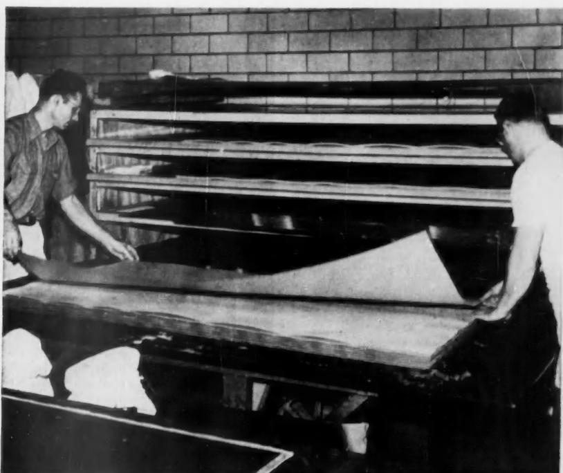
**3** After papers are cut to size, they are stacked in a build-up for pressing. Build-ups are composed of eight or nine sheets of kraft paper topped with the decorative print, transparent overlay, and a steel press pan to give the laminate its desired finish.
