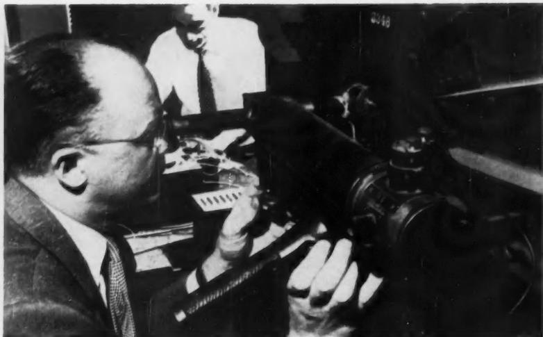
HEMISPHERICAL PHOTOMETER MEASURES TOTAL FLUX EMITTED BY SOURCE, WHETHER STANDARD LAMP, LUMINAIRE, FLOOD, OR SEARCHLIGHT.
