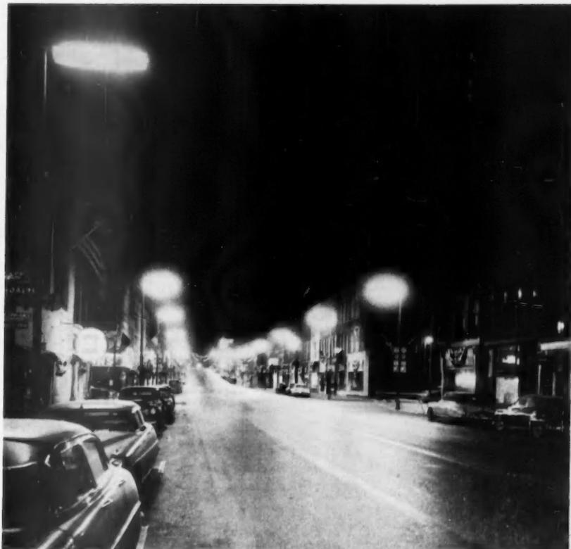
**WELL-DESIGNED STREET LIGHTING** provides a pleasant environment for pedestrians and drivers who are accustomed to comfortable interior lighting. The brightness of the obstacle against the pavement and the amount of unwanted light reaching the driver's eyes from the luminaire (illustration, left) determine whether he will see the obstacle he is approaching.
