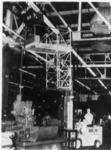
*Special equipment like this platform on a lift truck enables maintenance crew to change lamps quickly and easily.*
