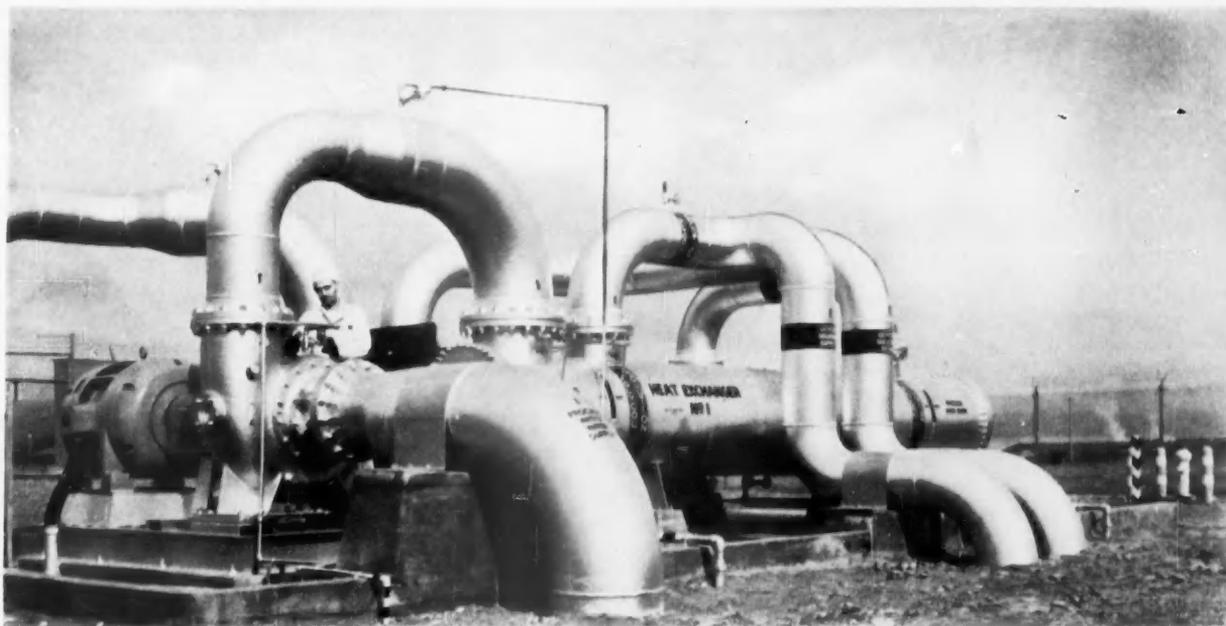
**MAIN HEAT EXCHANGER** of space-heating system utilizes heat energy from plutonium-producing reactors for heating Hanford buildings.
