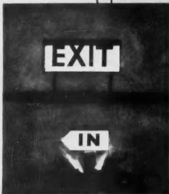
**GUIDE LIGHTING**—concealed fluorescent lamps light EXIT signs; IN have reflector flood or spot lamps in plant box.
