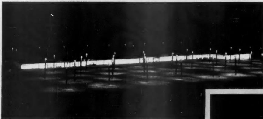
**STREETLIGHTING TECHNIQUES** (left) provide a simple lighting system, minimizing shadows. But many poles produce a cluttered effect and detract from show windows and signs. However, floodlighting (below) on 100-foot poles—above the line of sight—400 feet apart results in a much cleaner appearance.
