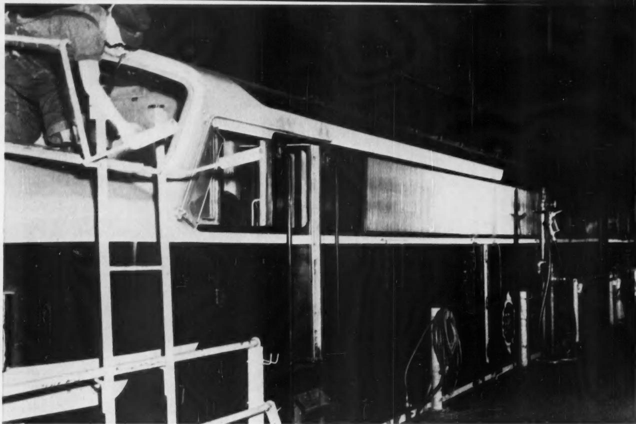
**1** For final grooming of the diesel-electric locomotive before its run, energetic Erie shop men wash down each unit; fuel it; check brakes and air lines; and make a general inspection before dispatching the locomotive to the yard for coupling to the train.
