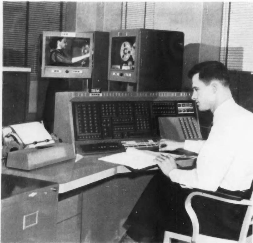
**HUMAN BEING** would have to compute 8 hours a day 5 days a week for 8 years without error to equal half-hour output of modern computer such as the IBM 702 or 704, which carries out 2000 to 5000 operations per second, also operating without error.
