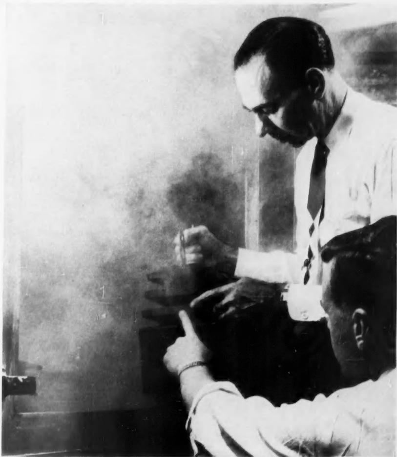
TRANSFORMER UNDERGOES EQUIVALENT OF YEARS OF EXPOSURE IN SALT-FOG CHAMBER.
