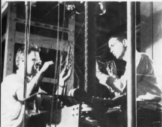
**SIMULATED FUEL ELEMENT** being installed in a heat transfer loop for tests under reactor thermal conditions. This is one of G.E.'s supporting atomic development programs to advance reactor design.
