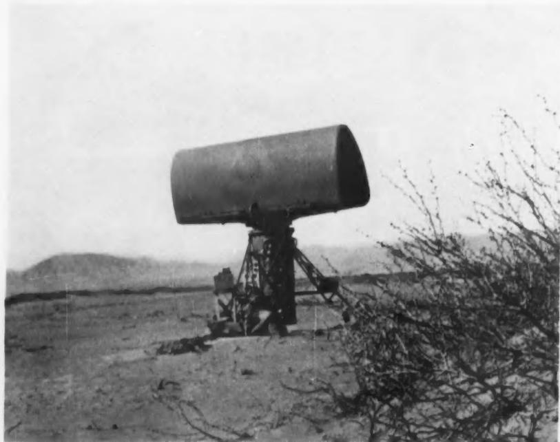
**GROUND-LOCATED RADARS** developed for Army Ordnance installations form an essential part of the beam-riding missile guidance system by directing the Nike to its target.
