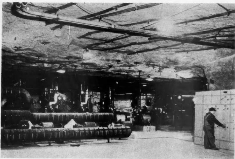
**UNDERGROUND FREEZER** warehouse uses rigid conduit to carry cables in electric system.
