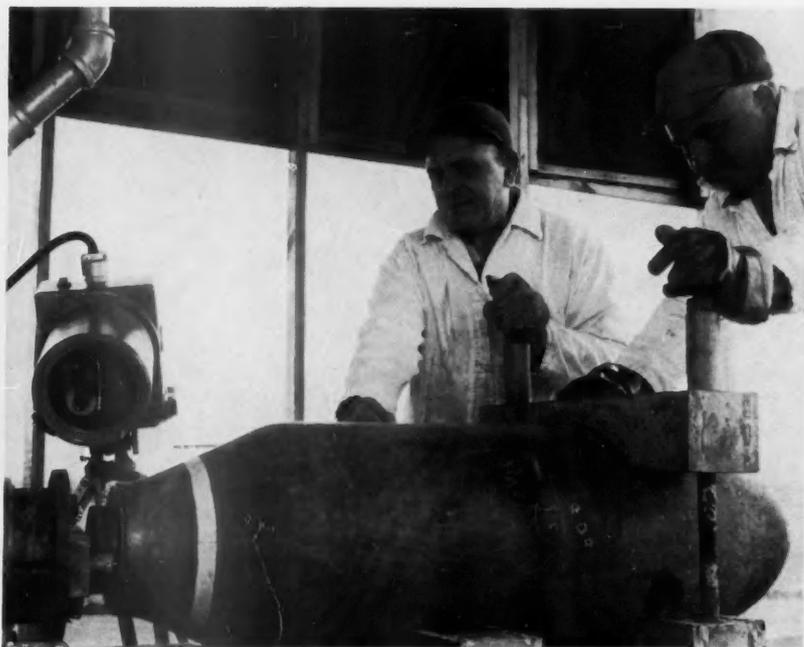
**TV CAMERA** in explosion-proof housing transmits picture of bomb deactivation to monitor.
