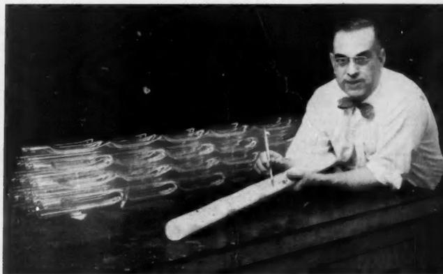
**LENGTHWISE DENTS** in a series along one side of 8-foot fluorescent "power groove" lamp give increased light output.
