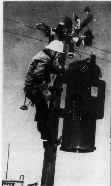
**LIMIT SWITCHES** on voltage regulators permit linemen to adjust units in service.
