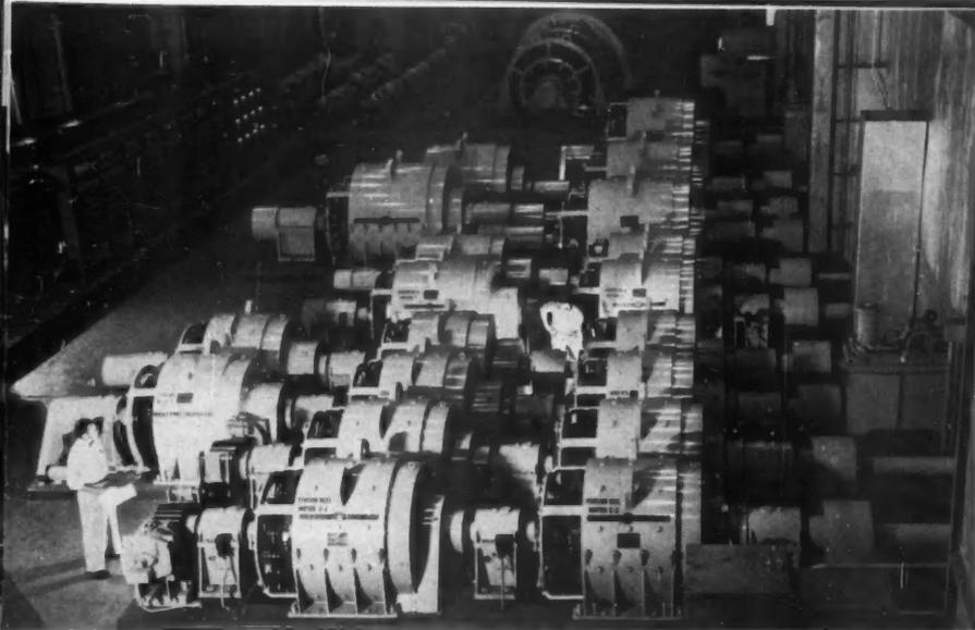
**D-C MOTOR DRIVE** at the new Weirton Steel Company supplies 28,000 hp. The installation makes steel strip at 80 mph, with thickness control within precise limits.
