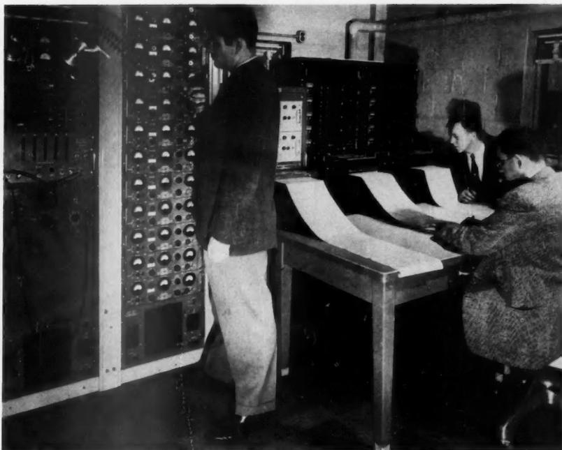
**RADIO TELEMETRY SYSTEM** aids the ground personnel in gathering test data from planes.
