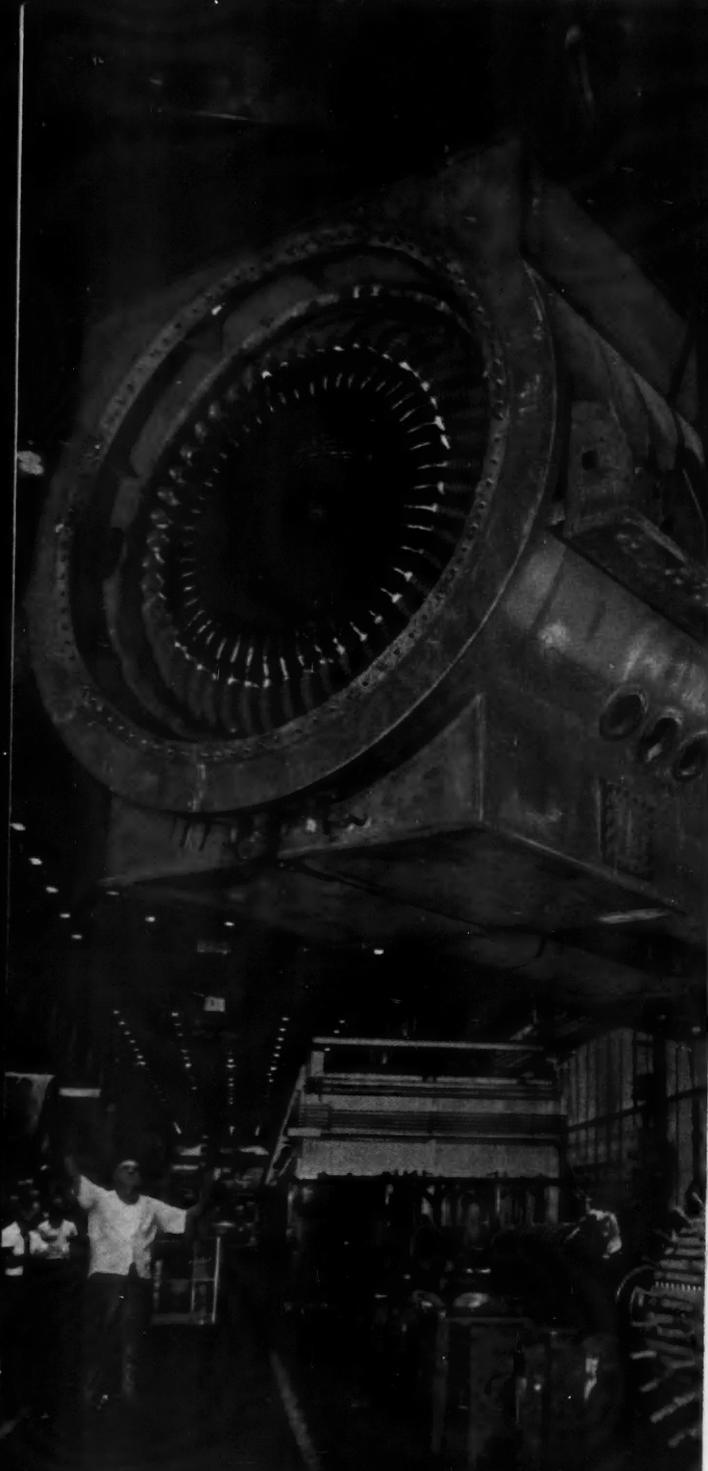
World's first large generator with liquid-cooled stator windings shown prior to shipment to The Cleveland Electric Illuminating Company's Eastlake Plant.
