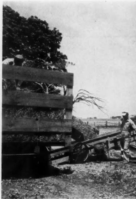
**Conveying** Electric conveyor system operated by generator loads baler.
