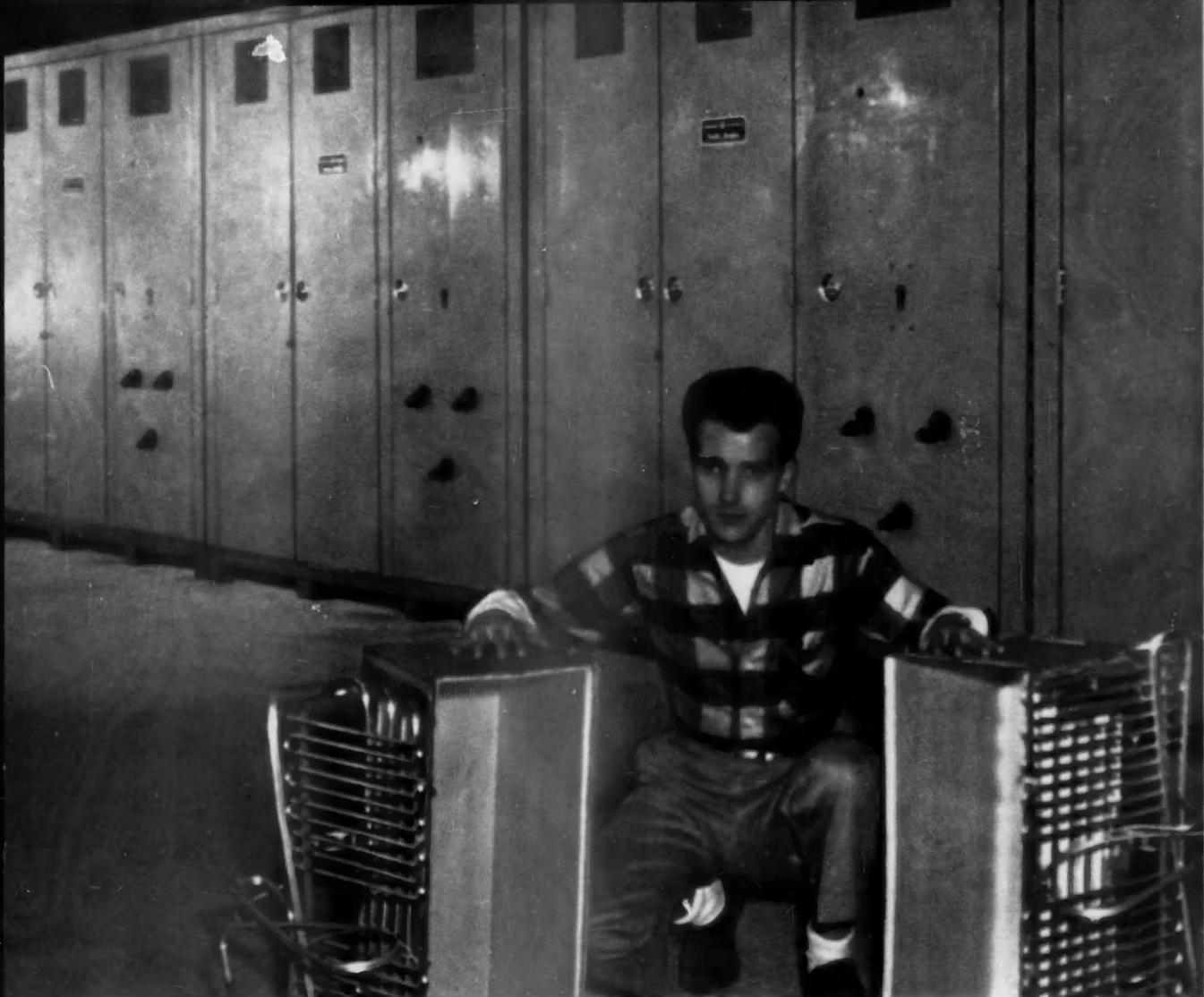
**DC POWER FOR ALUMINUM ANODIZING**—The G-E Germanium rectifier installation shown in the background supplies d-c power for anodizing the aluminum evaporators used in home refriger-
