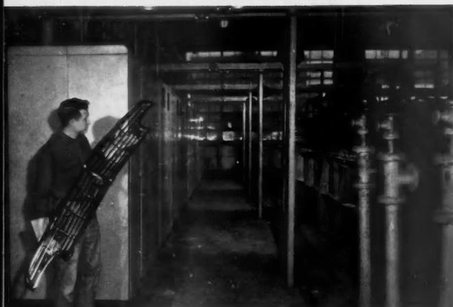
**DC POWER FOR AUTOMOTIVE PLATING**—This automobile grille has just been removed from the chromium plating tank shown at the right. Behind the inspector is a G-E Germanium rectifier installation of eight cubicles which delivers 48,000 amperes at 12 volts d-c. The plating industry has been quick to realize the increased economy and reliable service offered by Germanium rectifiers.
