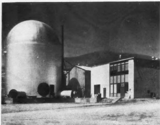
**PURPOSE OF EXPERIMENTS** to be conducted in Developmental Boiling Water Reactor is to develop economic nuclear power. Facility will furnish steam to 5000-kw turbine-generator, owned and operated by Pacific Gas & Electric Company.
