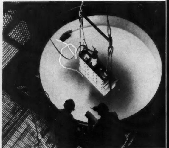
**REFUELING PROCEDURES AND EQUIPMENT DESIGN** are studied in 54-foot-high refueling test tank in San Jose. Tank simulates reactor pressure vessel conditions, including heat and water-circulating factors.
