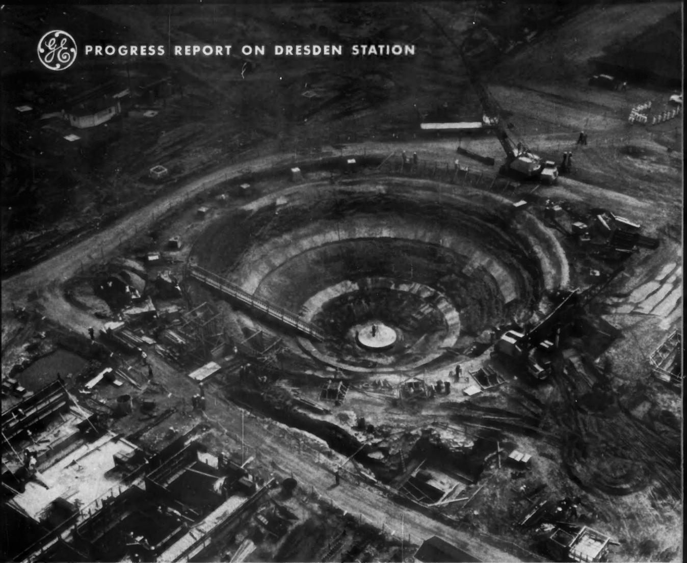
**GENERAL ELECTRIC DUAL-CYCLE BOILING WATER REACTOR** will be housed in 190-foot steel sphere on foundation already completed at Dresden site. Turbine building construction, lower left, is well under way.
