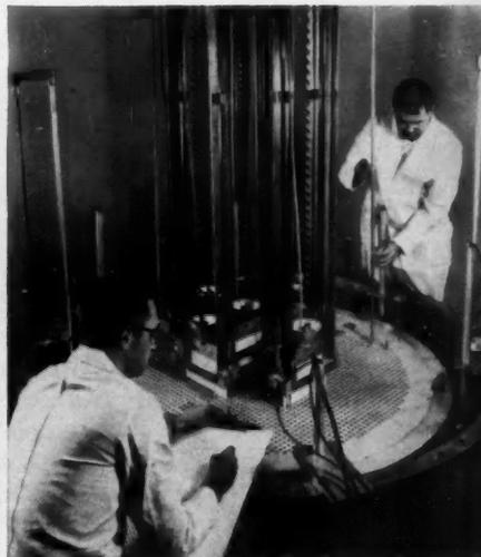
**CRITICAL EXPERIMENTS** at Vallecitos Atomic Laboratory will be performed with Dresden core mock-up to study core configurations and fuel loadings.
