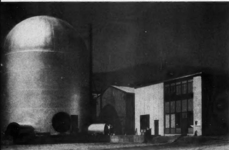
**DEVELOPMENTAL BOILING WATER REACTOR** at General Electric Vallecitos Atomic Laboratory will furnish vital operational data to be used for Dresden Station. Turbine-generator for facility will be owned and operated by Pacific Gas and Electric Company.
