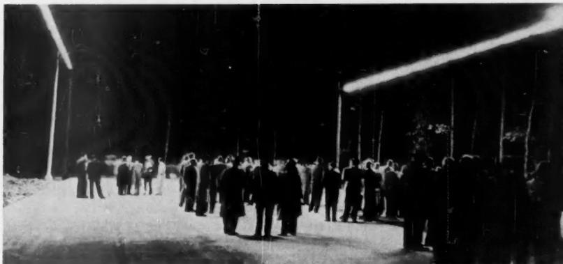
**PARALLEL-TO-ROADWAY** fluorescent luminaires in a continuous row at a distance of about 25 feet above the pavement give almost perfect uniformity of light on the road.
