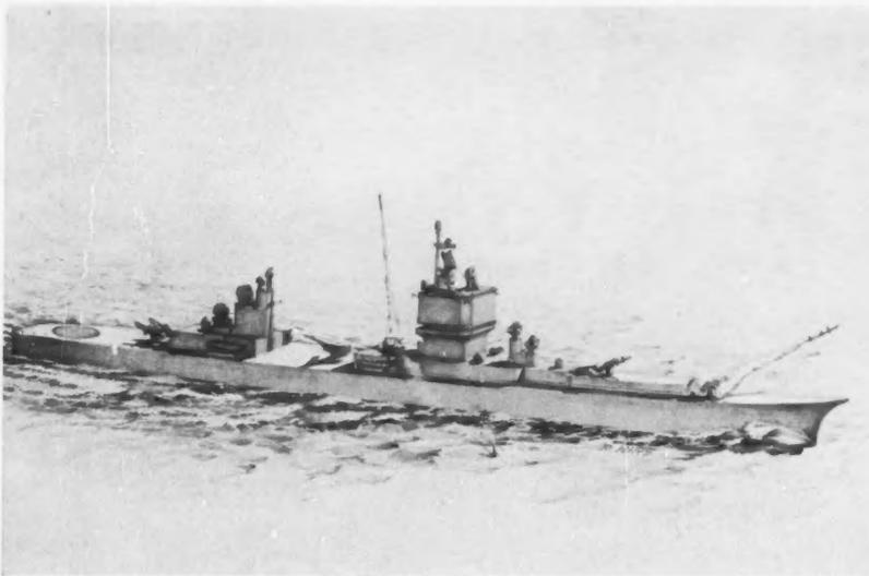
**ATOMIC POWERED GUIDED-MISSILE CRUISER**, the first nuclear propelled surface ship, will utilize steam supplied by cross-compound turbines from a pressurized water reactor.
