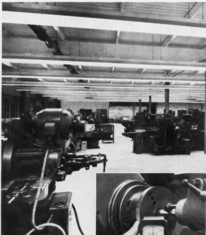
**AT ERICKSON TOOL COMPANY** (above), 450 G-E Power-Grooves, eight feet long, mounted 10 feet high, with 10 feet between rows, maintain a lighting level of 160 footcandles economically. This means there is plenty of light right at the machines (see footcandle reading at right)—where extra light means extra safety, extra accuracy for workers. No supplementary lighting is needed. Powerful Power-Grooves do it all!
