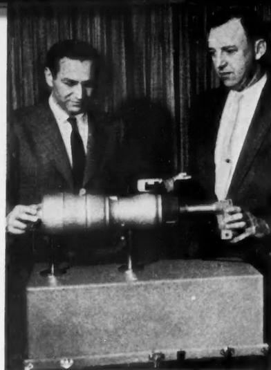
**TWO-IN-ONE** aircraft gas-turbine engine is both turboshaft and turboprop power plant.
