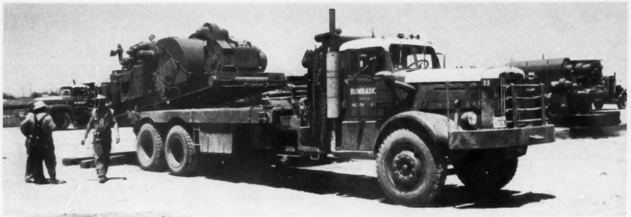
**DIESEL-ELECTRIC POWERED** oil-well drilling-rig drives have the advantage of excellent portability, speeding preparation cycle.
