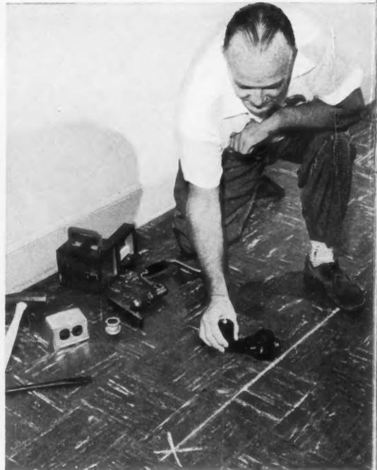
**MAGNETIC INSERT FINDER** locates concrete-buried steel-duct inserts in underfloor distribution systems.
