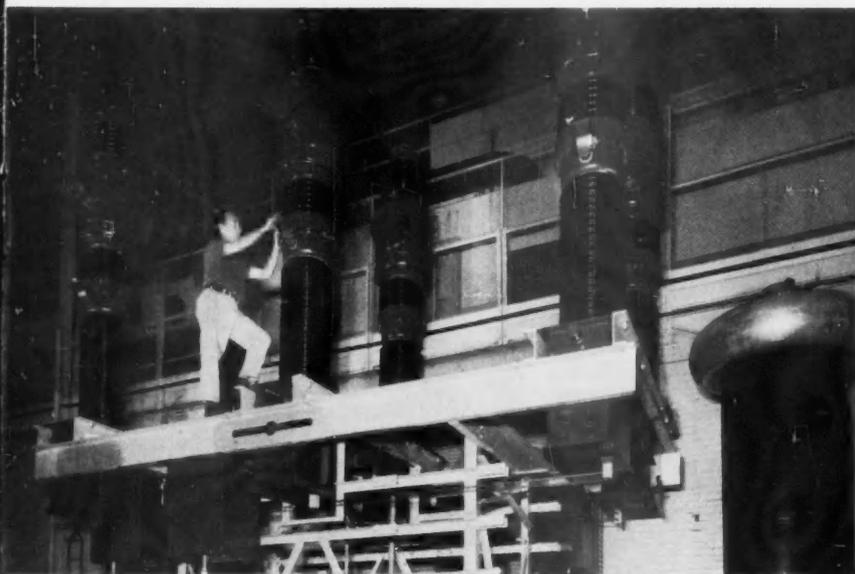
**AIR-BLAST CIRCUIT BREAKERS** improve interrupting efficiency and operating speed with newly designed interrupter elements mounted within their own high-pressure air-storage tank.
